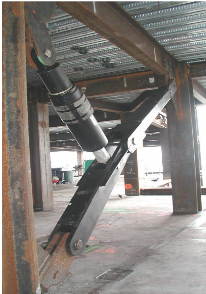
FIGURE 11-6 Reverse-toggle Brace Installation
