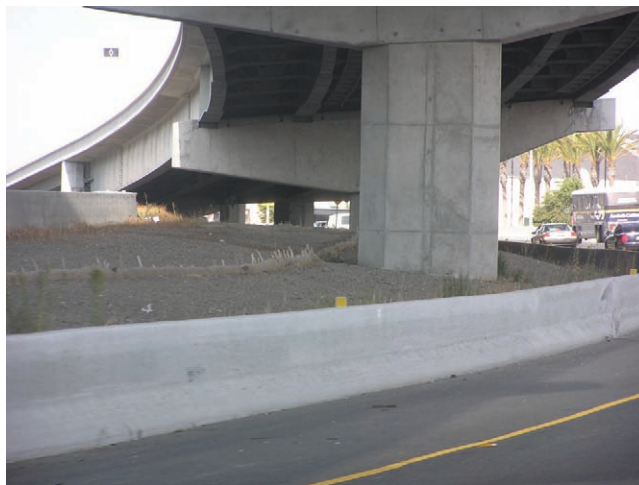
FIGURE 2-2 Reinforced Concrete Pier-Bent Cap Construction
