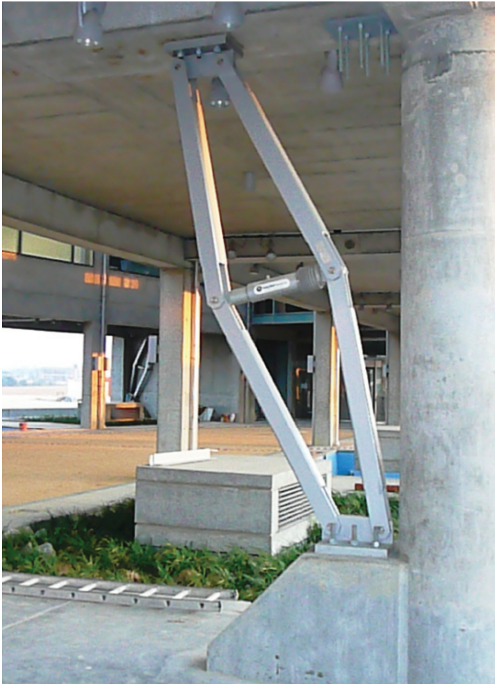
FIGURE 11-7 Scissor-jack Assembly Installation
