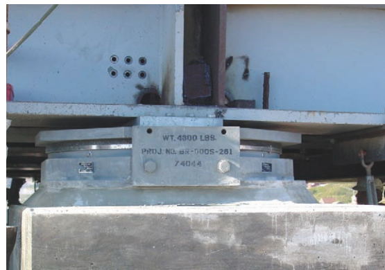
b. Friction Pendulum seismic isolator
