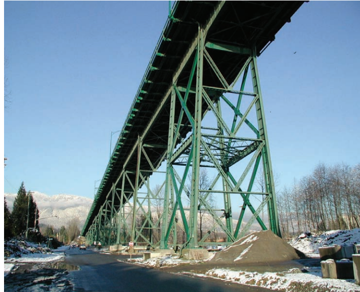
FIGURE 11-1 Braced Steel Piers
