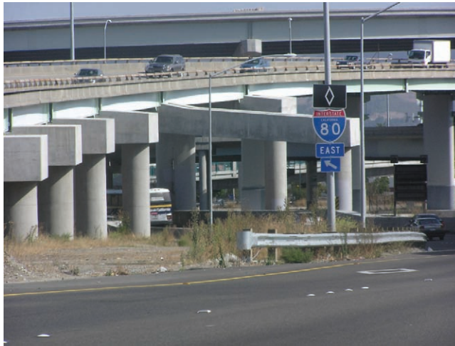
FIGURE 2-1 Reinforced Concrete Moment-Resisting Frame Construction
