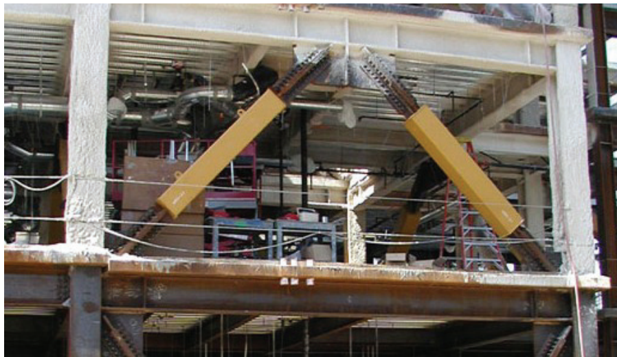
FIGURE 11-2 Chevron Brace Installation of Buckling Restrained Braces
