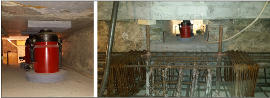
Fig. 9. Position of the hydraulic jacks and LVDTs.
