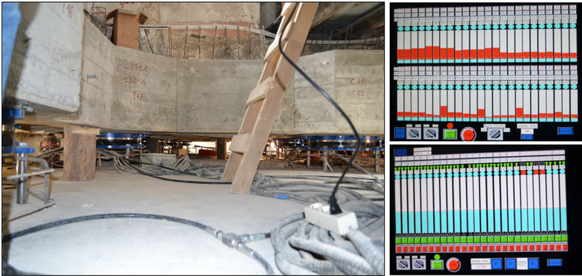
Fig. 15. Lifting process and the digital software for controlling the pressure in the hydraulic jacks.
