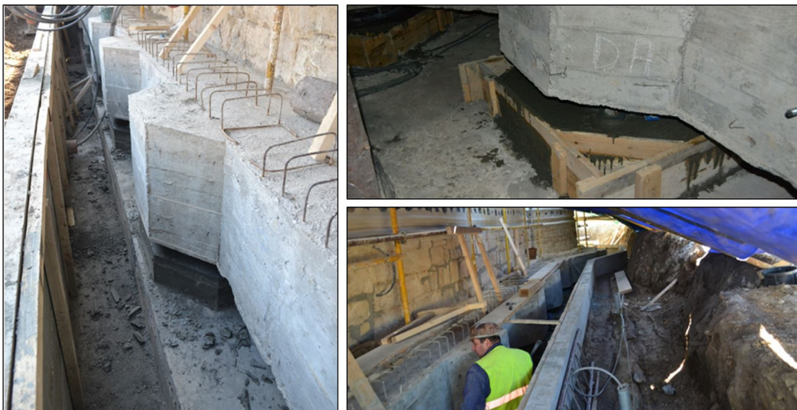
Fig. 16. Casting the base of the FPS isolators.
