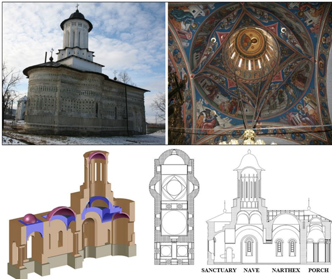
Fig. 3. St. Nicolae Aroneanu church: northern façade, the interior tower, 3D model – isometric view, plan view of walls and vaults, longitudinal section.
