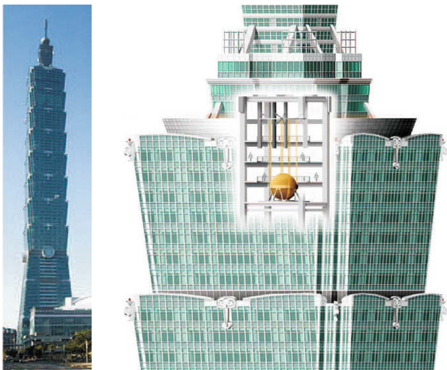
Figure 1. Dynamic Vibration Absorber of the Taipei 101 building. The DVA consists of a pendulum with a mass of 730 tons suspended with 4 cables extending over 4 floors.
