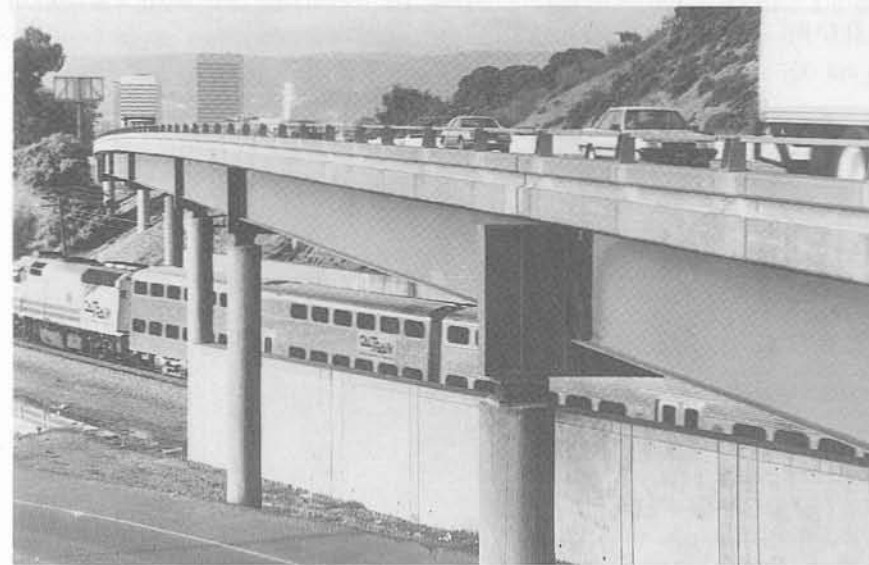
Figure 6.28 Sierra Point Overhead Bridge, San Francisco, seismically isolated by retrofitting with lead-rubber bearings (photograph courtesy Dynamic Isolation Systems, Incorporated)
