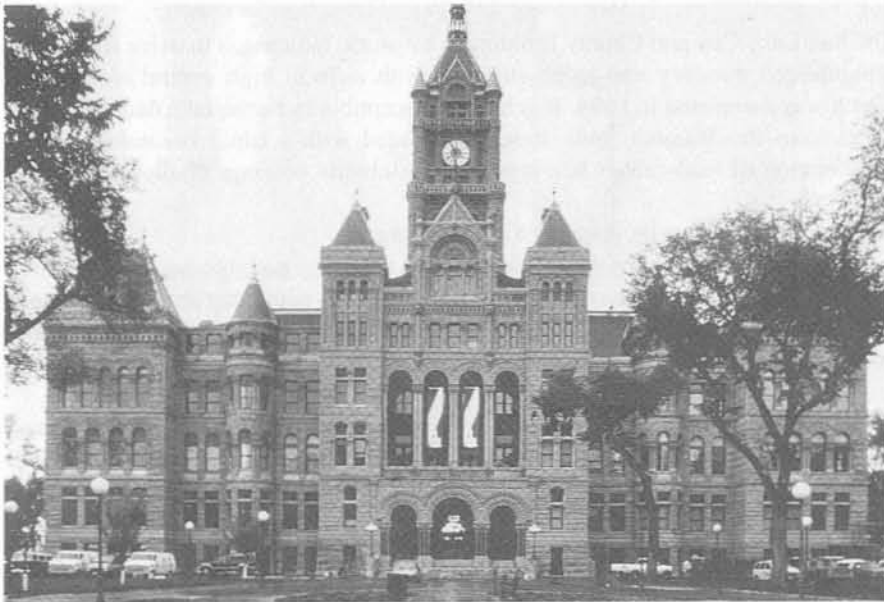
Figure 6.25 Salt Lake City and County Building, Utah; an historic building retrofitted with seismic isolation (photograph courtesy Dynamic Isolation Systems, Incorporated)
