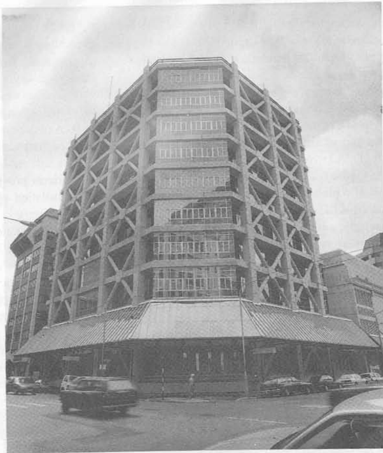
Figure 6.12 Wellington Central Police Station; note the external diagonal bracing
