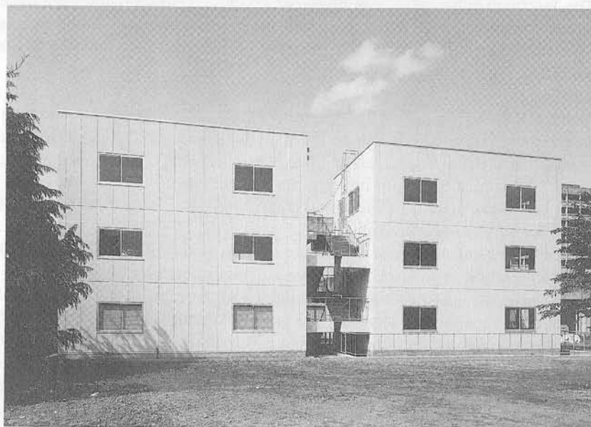
Figure 6.16 Test Buildings at Tohoku University. On the left is the conventional building, and on the right is the seismically isolated building (photograph courtesy Shimizu Corporation)
