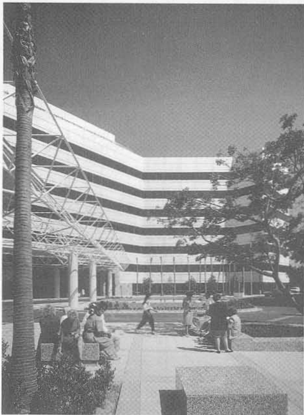
Figure 6.27 Completed USC Hospital, Los Angeles, California (photograph courtesy Dynamic Isolation Systems, Incorporated)
