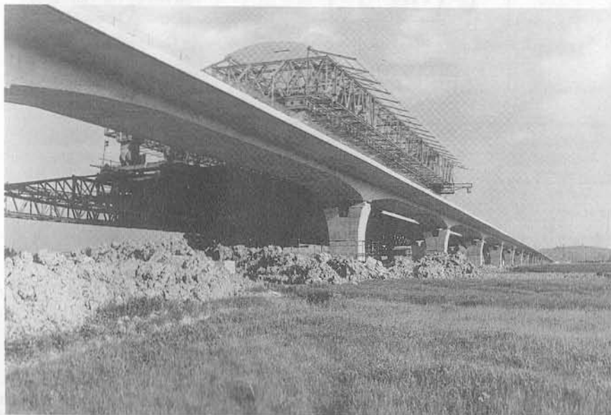
Figure 6.33 Mortaiolo Bridge near completion (photograph courtesy A Parducci)
