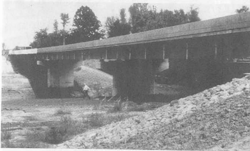
Figure 6.29 Sexton Creek Bridge, Illinois, fitted with lead-rubber bearings (photograph courtesy Dynamic Isolation Systems, Incorporated)
