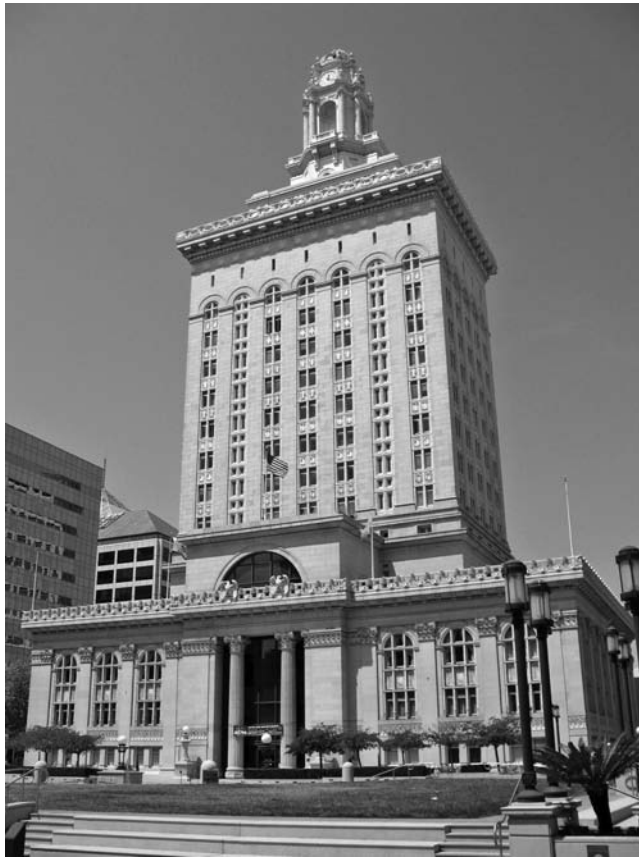
Figure 1.8 The Oakland City Hall, Oakland, California. Courtesy of James M. Kelly, University of California, Berkeley
