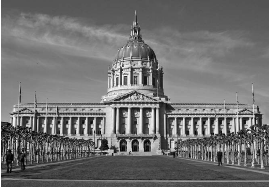
Figure 1.10 The San Francisco City Hall, San Francisco, California. Courtesy of James M. Kelly, University of California, Berkeley
