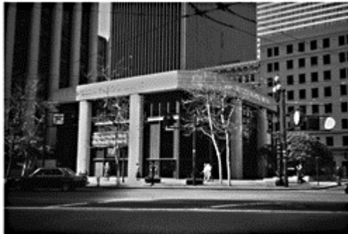
Figure 5.7.7 Wells Fargo Building, San Francisco, California
