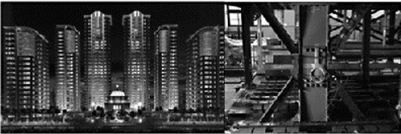
Figure 5.6.10(a) Application of VE dampers, Taipei Treasure Palace
