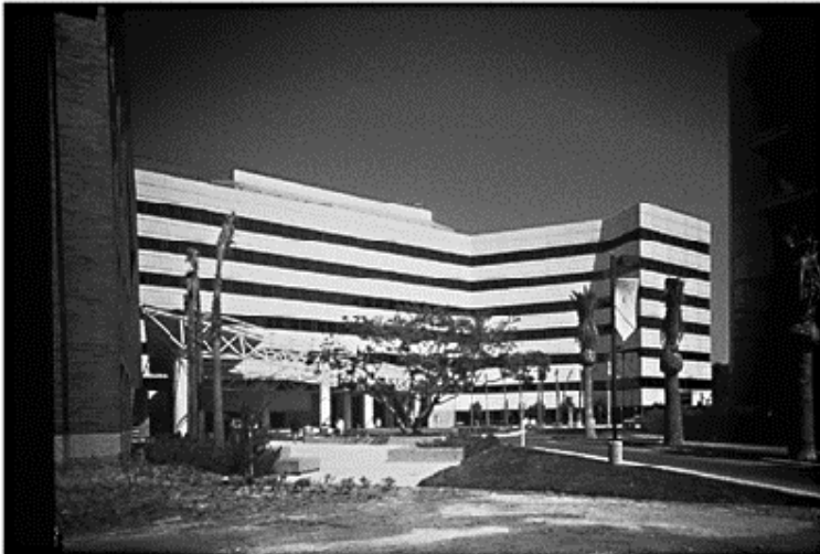
Figure 4.6.1 University hospital building
