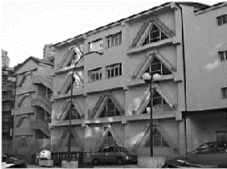
Figure 5.2.9 Dissipative braces provided with EPDs at their ends installed in the “Domiziano Viola” school at Potenza for its retrofit (photographs by the courtesy of Tis, Rome, Italy)
