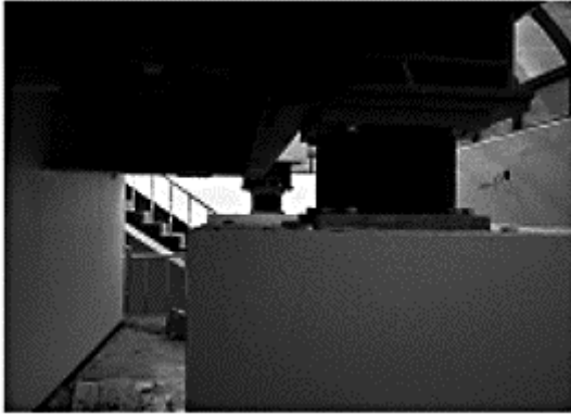
Figure 5.4.8 LRB on a pedestal
