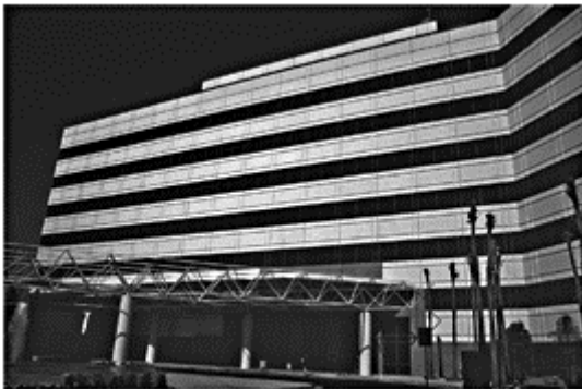
Figure 5.7.4 USC University Hospital, Los Angeles, California
