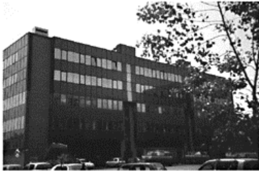
Figure 5.2.3b Mobile Brigade building of the new Fire Station at Naples (1985) (photograph by the courtesy of Prof. F.M.Mazzolani)
