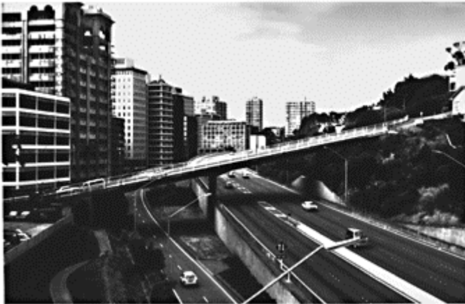
Figure 5.5.6 An over-bridge in Wellington city seismically isolated by using flexible piles and lead extrusion dampers (supplied by Robinson Seismic Ltd.)
