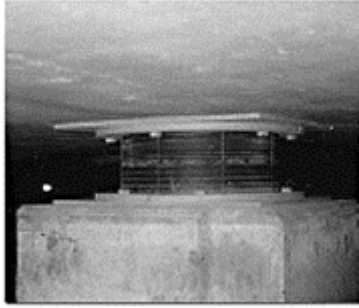
Figure 5.4.4 LRB on pedestal
