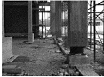
Figure 5.2.26 Isolated fire building being constructed at the Foligno Civil Defence Centre and view of some of its HDRBs and SDs (2004) (photographs by the courtesy of Tis, Rome, Italy)
