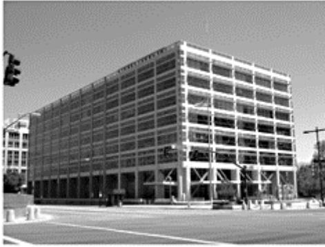
Figure 5.7.10 Wallace F. Bennett Federal Building, Salt Lake City, Utah
