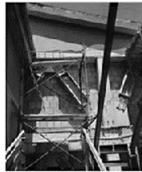
Figure 5.2.9 Dissipative braces provided with EPDs at their ends installed in the “Domiziano Viola” school at Potenza for its retrofit (photographs by the courtesy of Tis, Rome, Italy)
