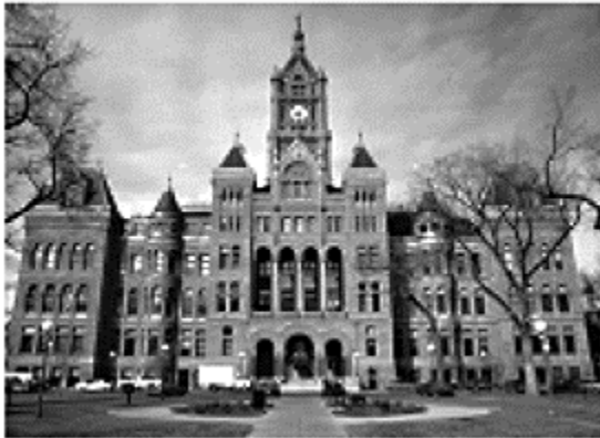
Figure 5.7.2 City and County Building Salt Lake City, Utah
