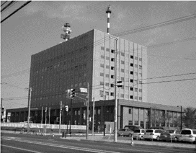
Figure 4.3.1 Government office building
