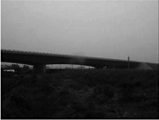
Figure 5.6.13(a) General view of the seismically isolated Bai-Ho bridge
