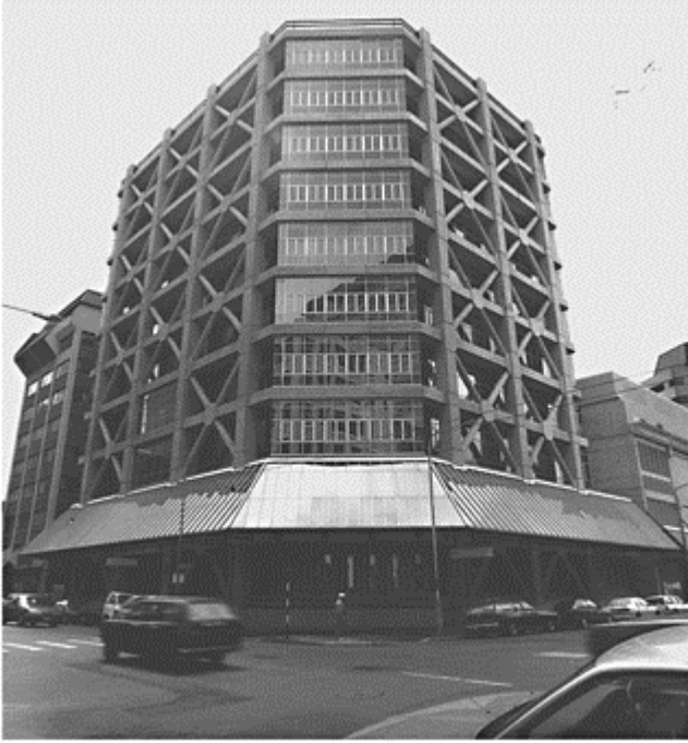
Figure 5.5.10 Wellington Central Police Station (supplied by Robinson Seismic Ltd.)
