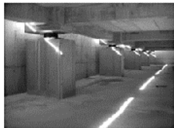
Figure 5.2.25 New isolated section of the Gervasutta Hospital being erected at Udine and view of some of its
