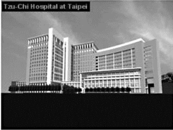
Figure 5.6.14(a) Application of isolation, Tzu-Chi Medical Center
