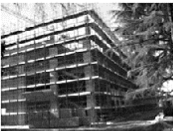
Figure 5.2.25 New isolated section of the Gervasutta Hospital being erected at Udine and view of some of its
