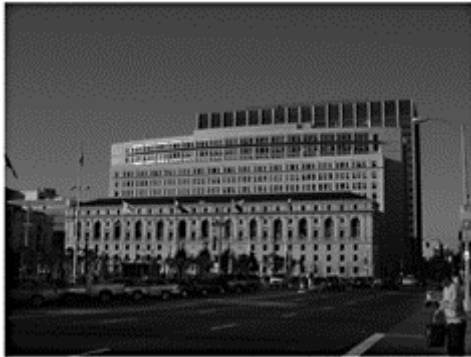
Figure 5.7.9 State Office Building, San Francisco, California
