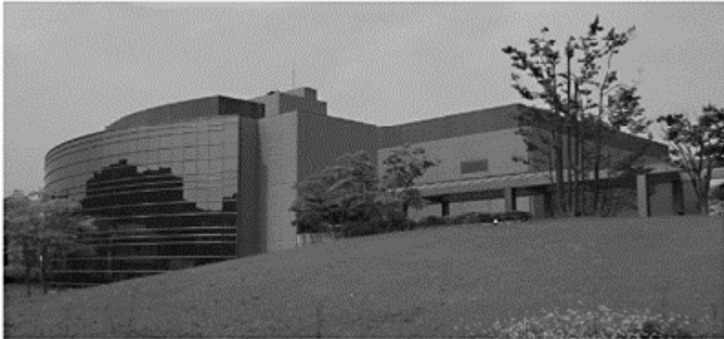
Figure 4.4.1 Computer service building
