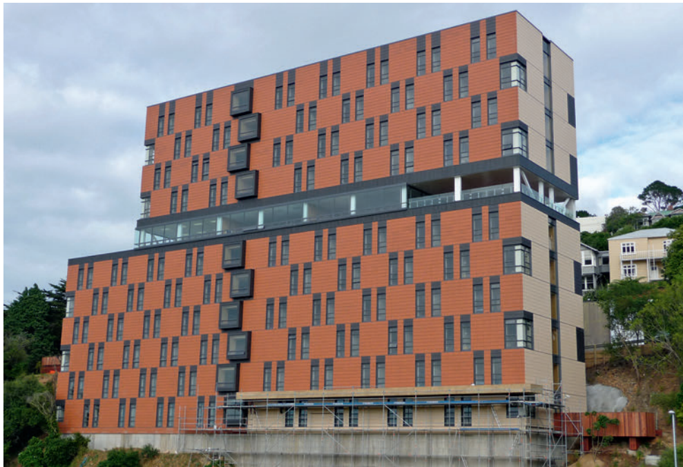
1.6 A damage-free structure in a hostel at Victoria University of Wellington, New Zealand. In the event of seismic overload, structural steel connections in the moment frames (along the building) and cross-braced frames (across), slip rather than break
