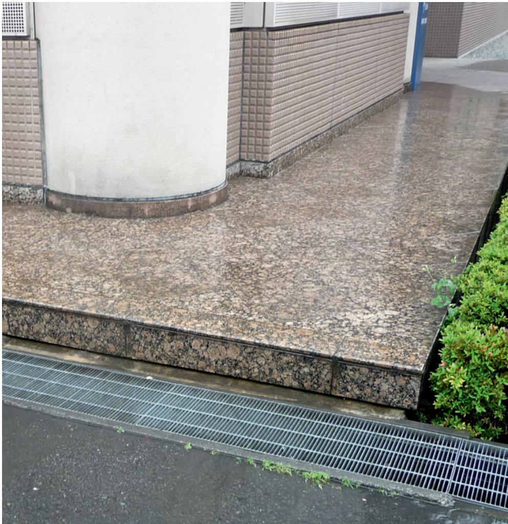
8.9 A cantilever slab moat cover moving into and away from a garden on one side and forming a step at a paved area on the other, Tokyo, Japan
