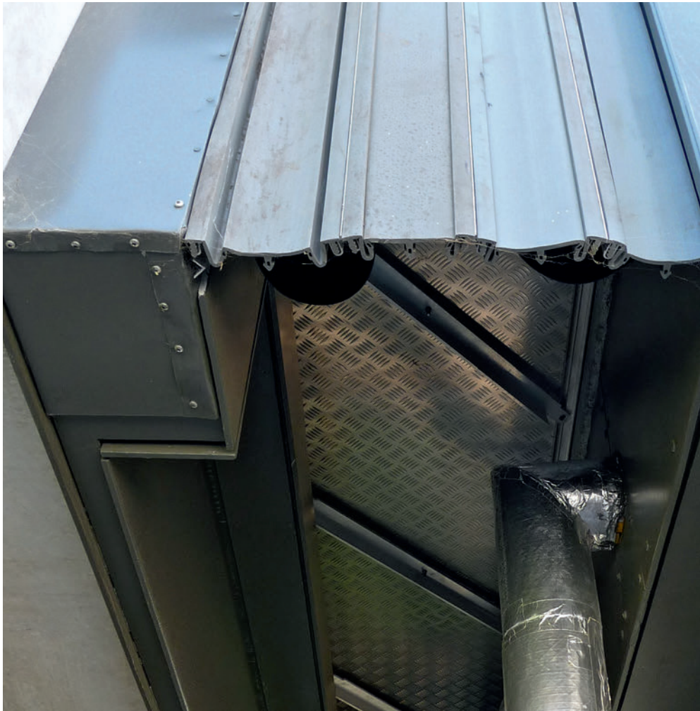
8.20 The underside of a self-centring floor cover plate. Diagonal bars that centre and support the plate are visible as well as a flexible elastomeric wall joint, Wanganui, New Zealand
