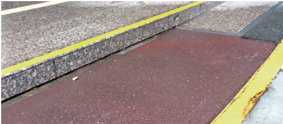
8.14 A transition area where the surface of a cantilever moat cover that moves above the surrounding paving gradually becomes level with that paving, Tokyo, Japan
