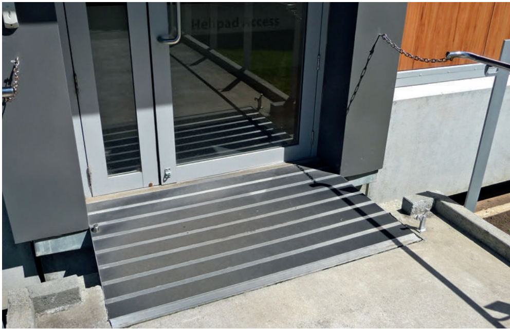
8.12 A steel cover plate at a secondary entrance slides over the exterior concrete paving. The chain linking the building to the handrail is considered sacrificial. It will break and be replaced after an earthquake, Wanganui, New Zealand
