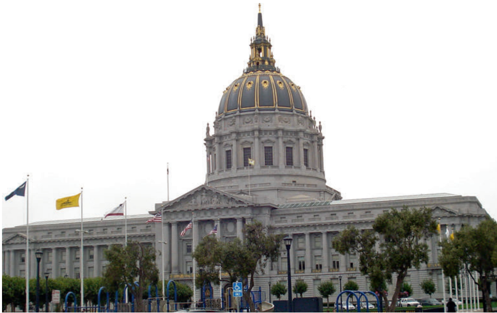
2.11 San Francisco City Hall, San Francisco, USA, retrofitted 1999
