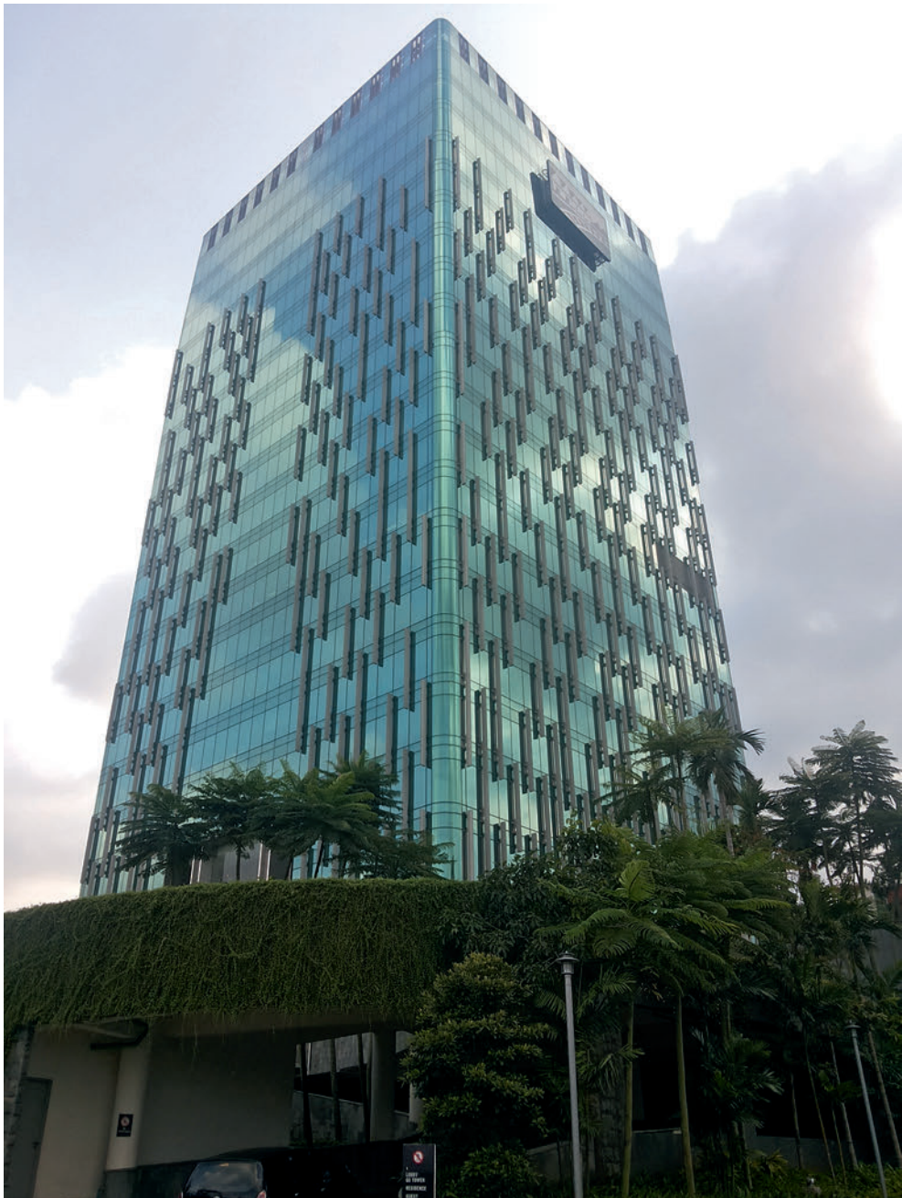
5.14 The Gudang Garam Tower, Jakarta, Indonesia. A seismically isolated 25 storey building
