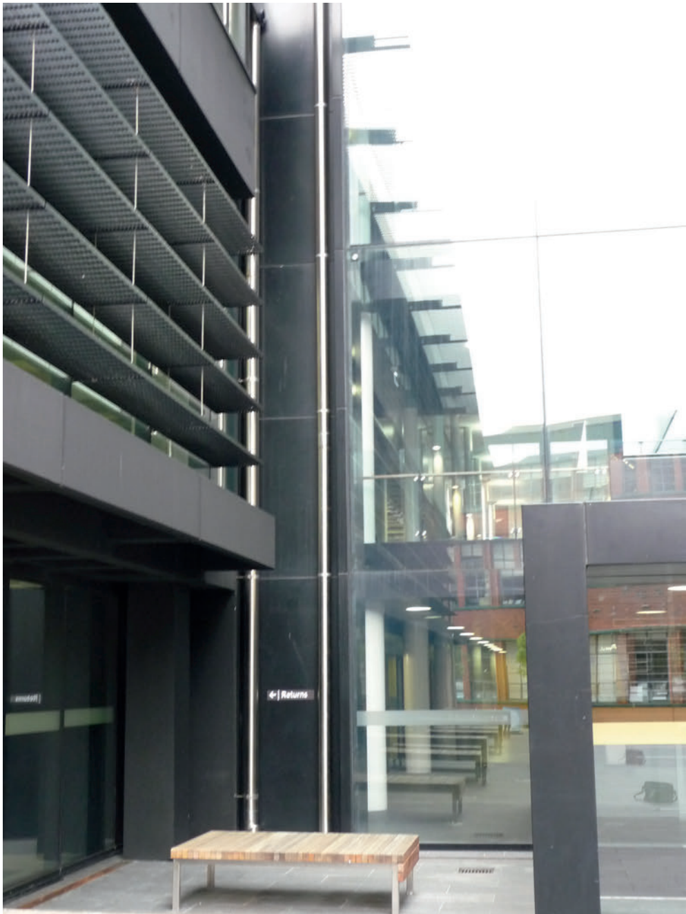
8.28 The vertical black painted thin metal covering is part of the wall movement joint between the seismically isolated building to the left and the fixed-base building to the right. The choice of materials and colour achieve an elegant transition. Sacrificial steel elements and frangible interior linings will need replacement after a moderate to large earthquake, Wellington, New Zealand
