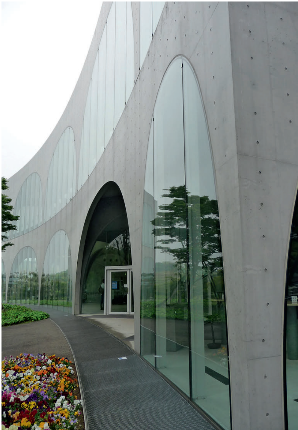
6.4 The smoothness of the façade looking towards the front entrance
