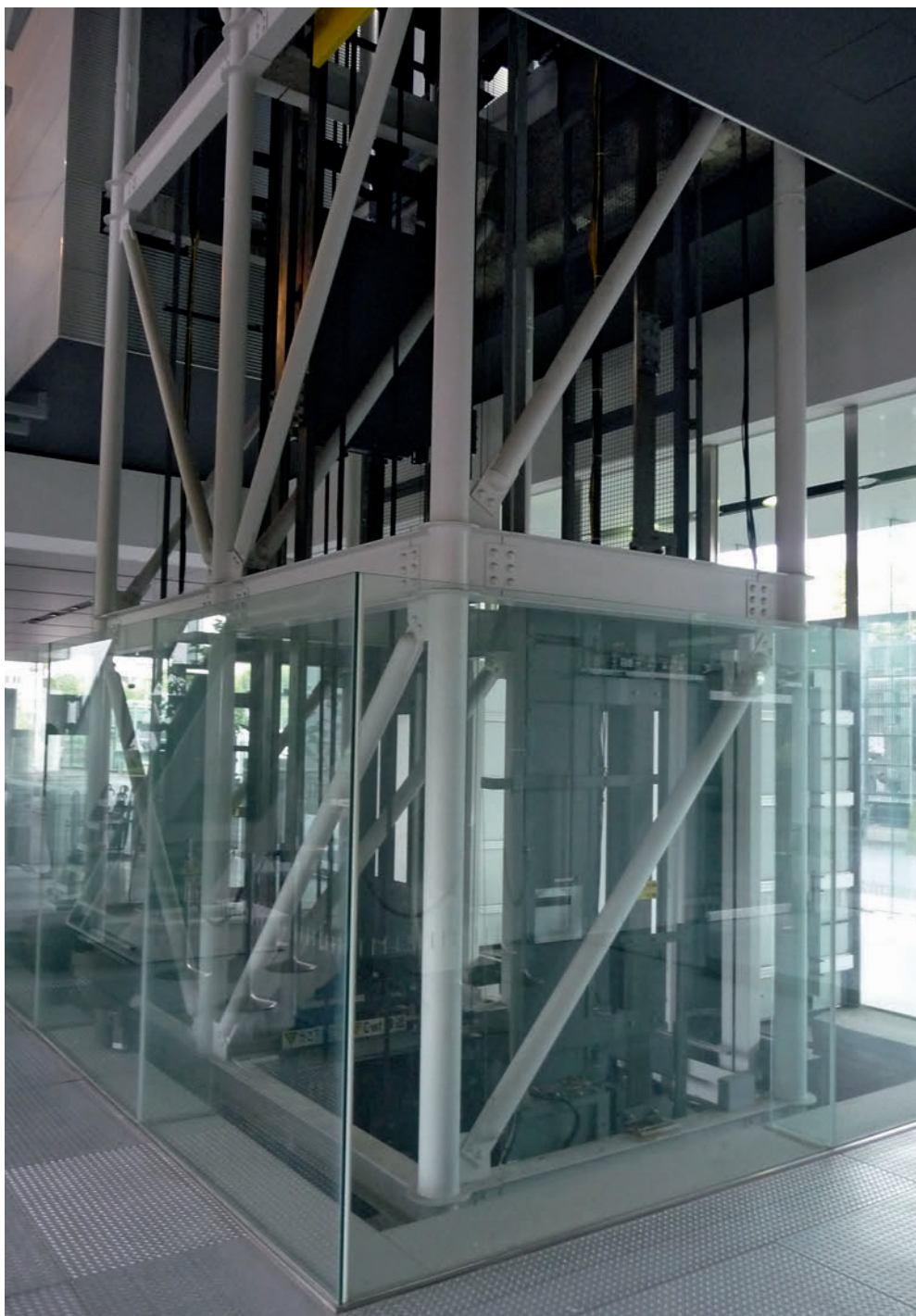
6.7 Structure around the elevators
