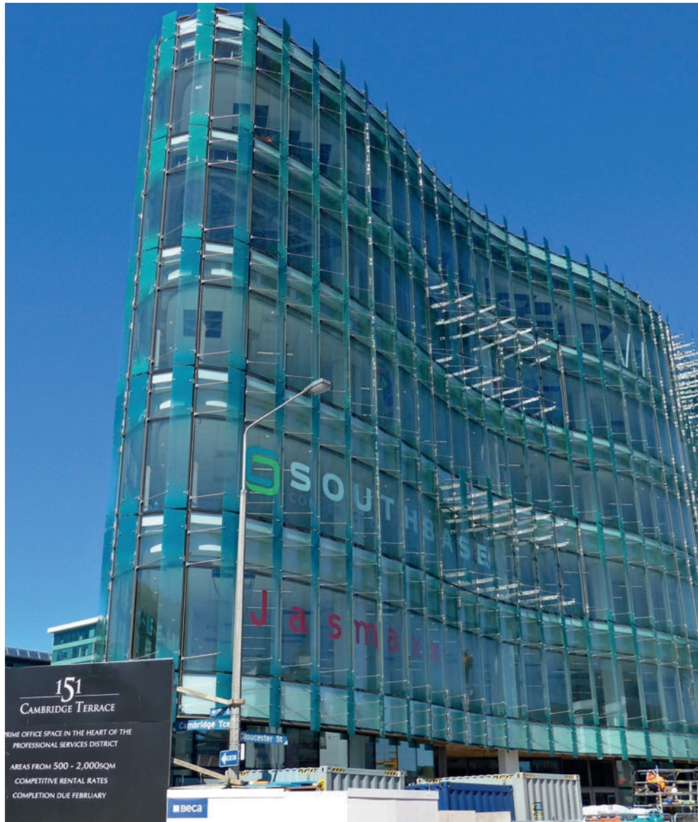
9.1 Office building in Christchurch where reduced horizontal inter-storey movement as a result of seismic isolation reduced the costs of the curved wall glazing
