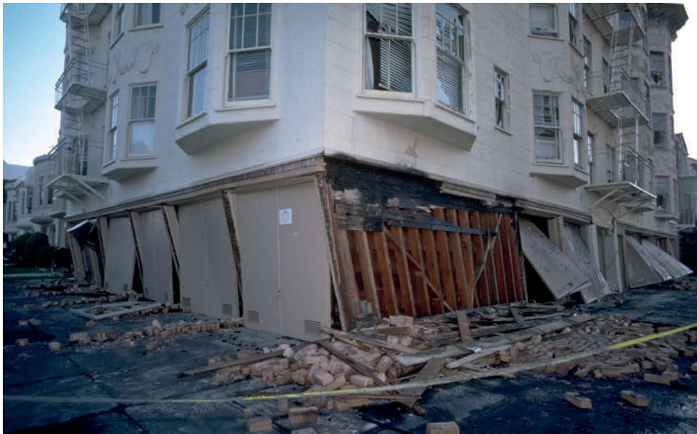
1.1 Example of structural damage in a building with inadequate shear walls at the garage level. Loma Prieta earthquake, San Francisco USA, 1989
