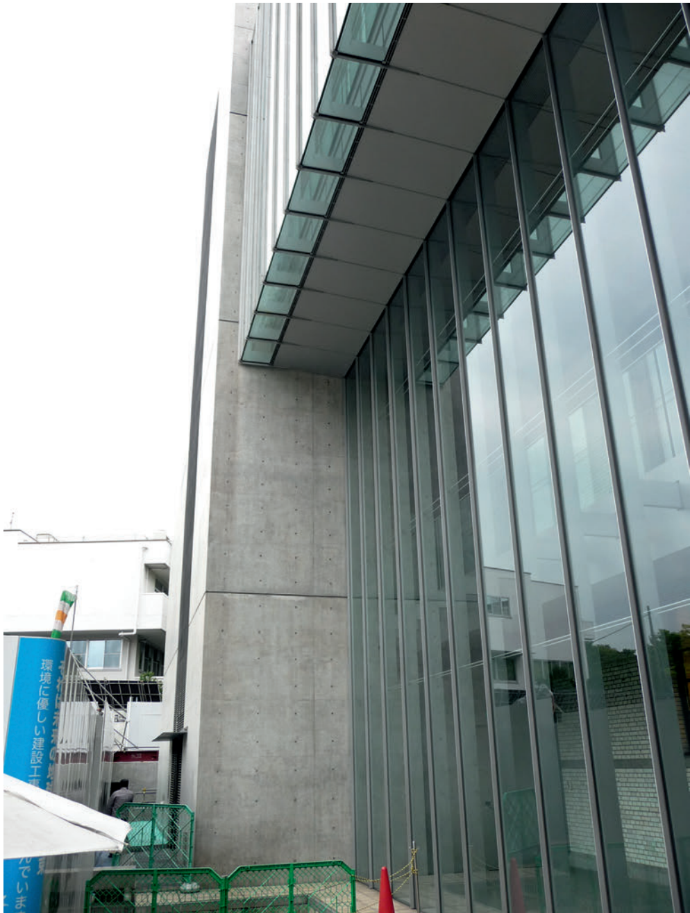
7.7 The new rear façade of the library that comprises two reinforced concrete cores and glazed walls
