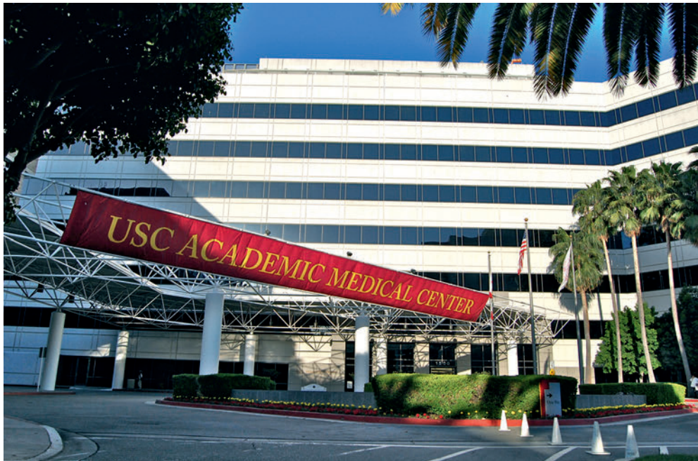
4.5 USC Hospital, USA, the world's first seismically isolated hospital, survived the 1989 Loma Prieta earthquake without damage
