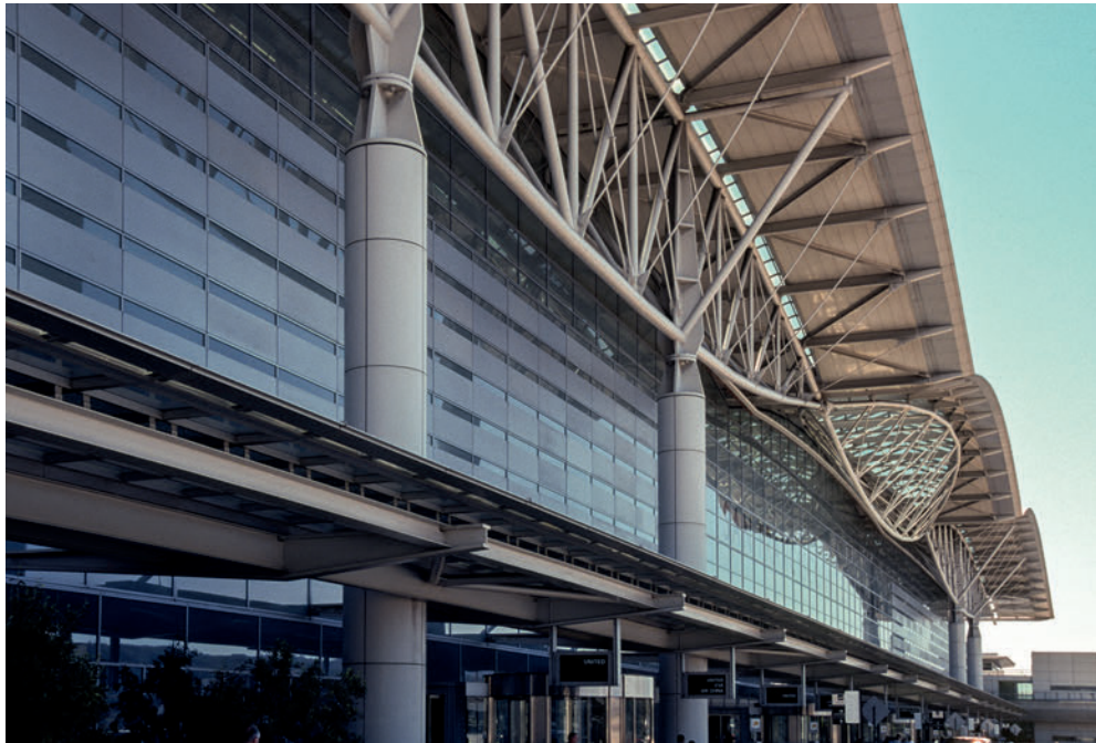
6.24 A view along the front of the building showing the cantilever columns
