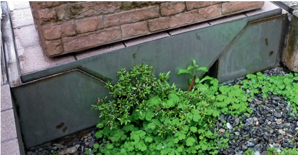
8.17 Detailing of a movement joint between isolated and fixed paving that utilizes angled sliding planes, Tokyo, Japan
