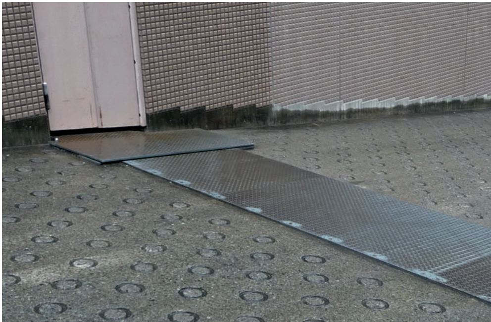
8.13 A steel moat cover across a vehicle ramp, Tokyo, Japan
