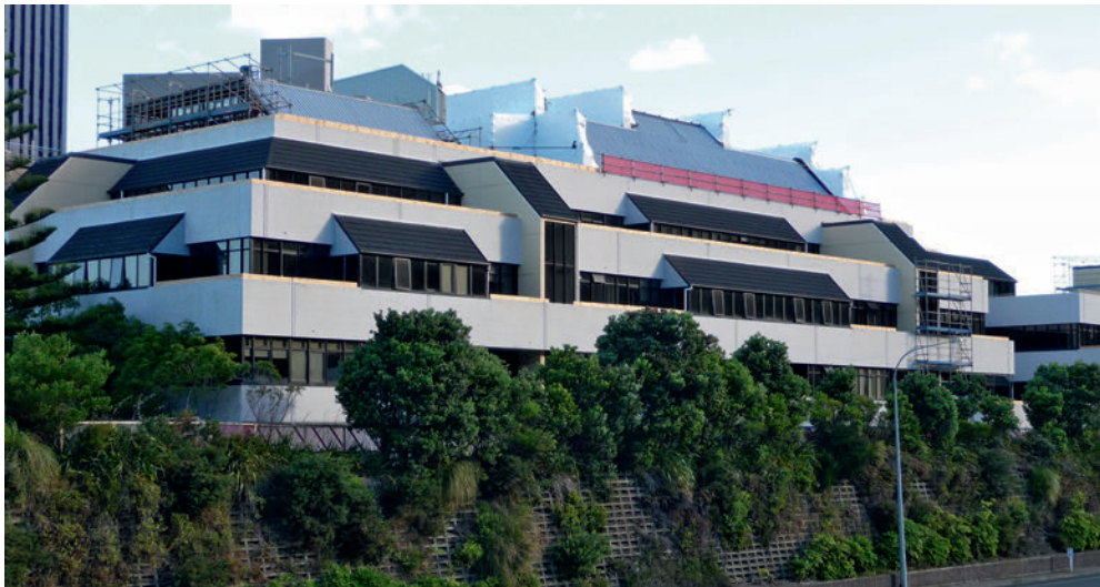
2.1 The William Clayton Building, New Zealand, Wellington, 1981. The first example of the comprehensive application of seismic isolation
