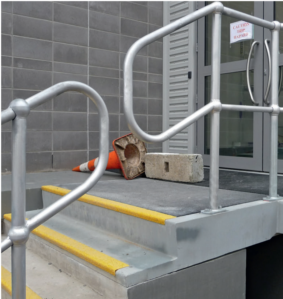
8.30 An external secondary stair. The stair landing cantilevers from the isolated building to the right and slides on the supporting pier. The handrails are separated to allow movement, Lower Hutt, New Zealand
