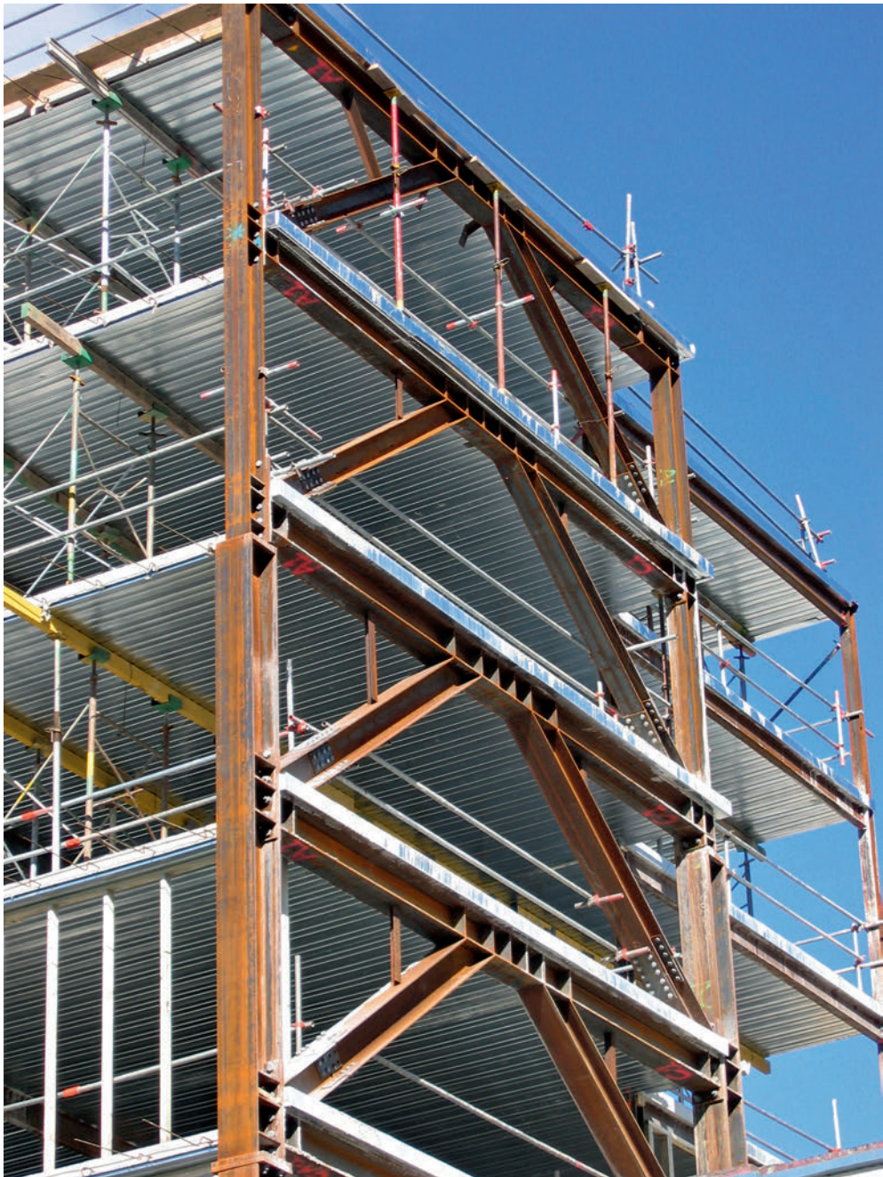
1.4c Example of a type of structural system: eccentrically braced frame
