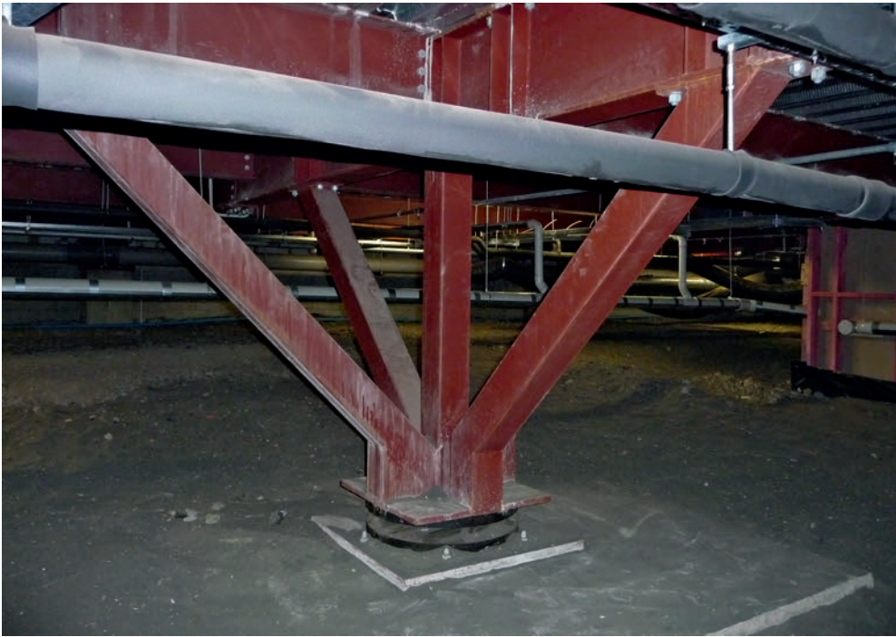
3.19 A RoGlider™ installed between a foundation pad and substructure framing under the Wanganui Hospital, New Zealand
