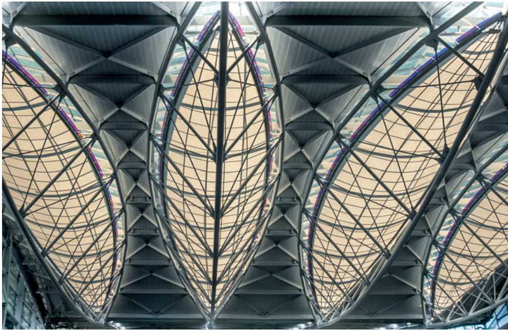
6.25 The three-dimensional steel roof trusses that flood the Departures Hall with light
