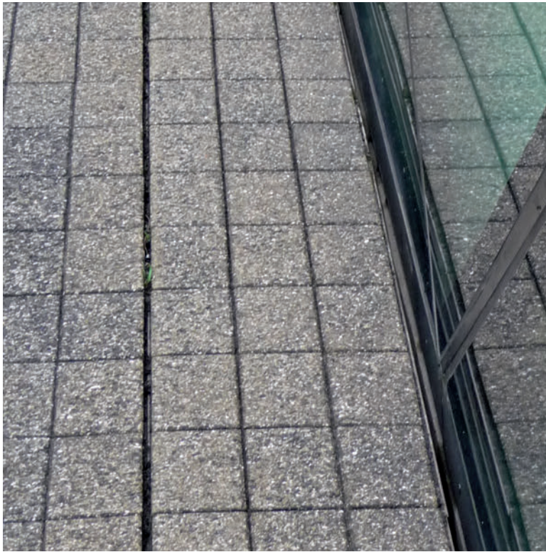
8.21 A cover plate allowing a full range of movement is almost indistinguishable from the surrounding area of paving. The plate is fixed to the building and due to its 45 degree sliding surface will slide across and along the moat gap below, Tokyo, Japan
