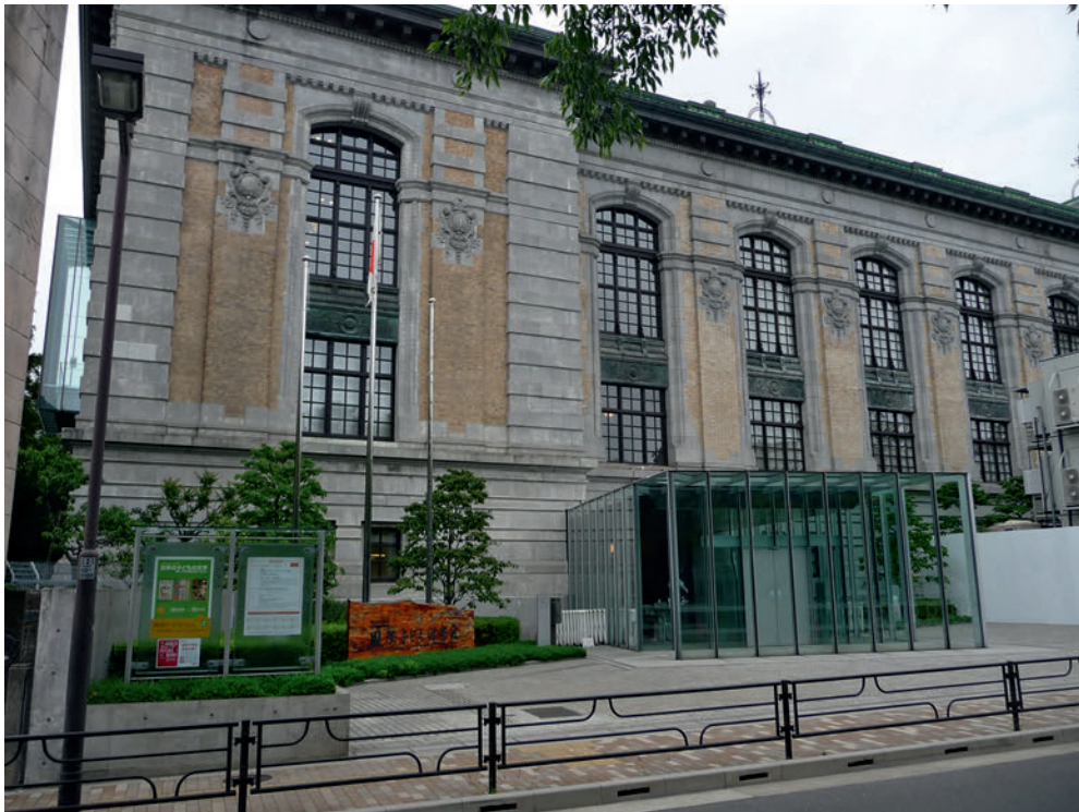
7.6 The International Library of Children's Literature, Tokyo, Japan. The main façade with the new glazed entry
