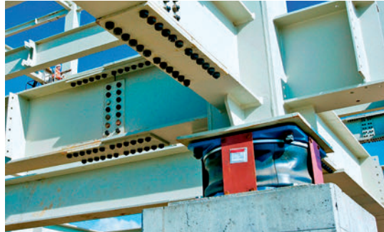
5.7 A bearing with its protective covering supports the steel framework
