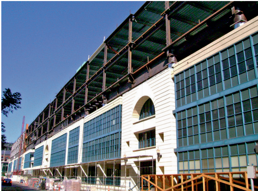
7.26 China Basin Landing office building during construction
