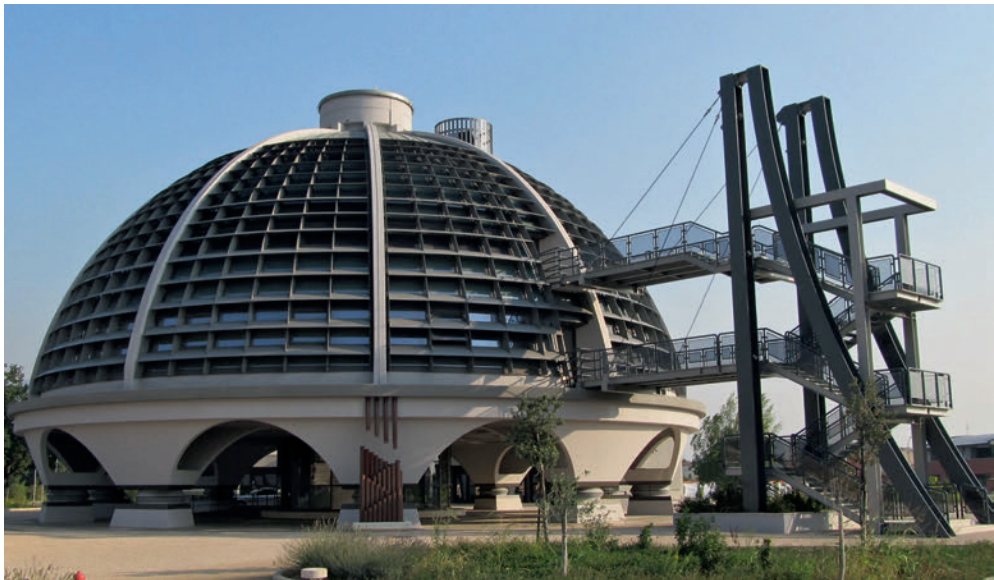
6.9 Emergency Management Centre, Foligno, Italy. Overall view including stairs
