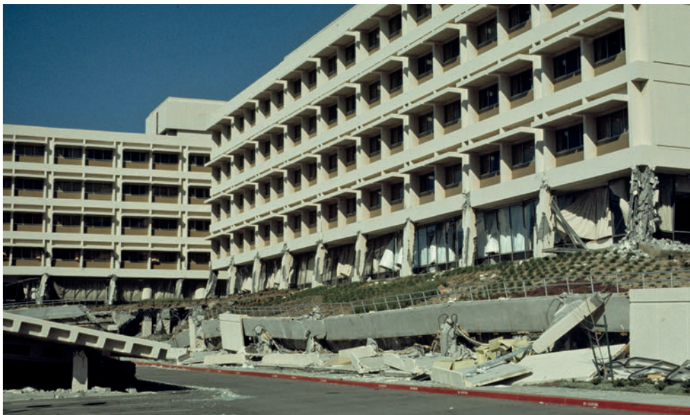
1.2 The seriously damaged Olive View Hospital moment frame building. San Fernando Valley earthquake, California USA, 1971
