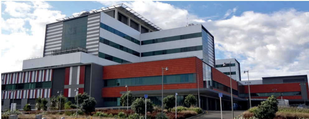
2.14 Wellington Regional Hospital, New Zealand, 2008
