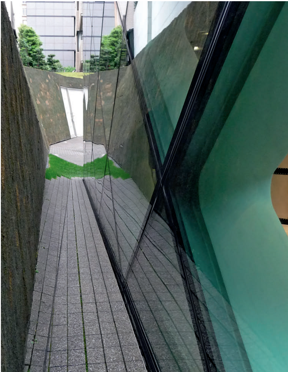
8.5 Horizontal clearance between a boundary retaining wall to the left and an isolated building to the right, Tokyo, Japan
