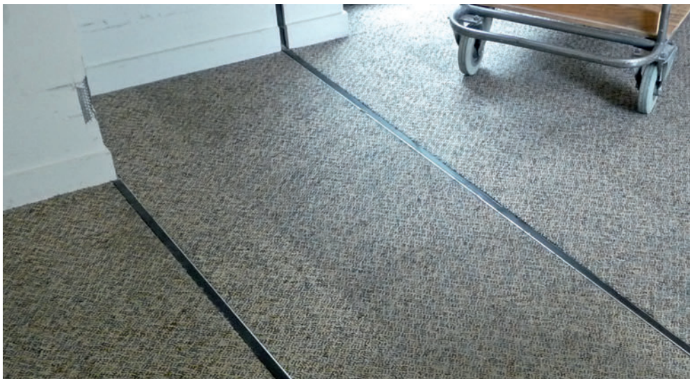
8.24 A flush mounted interior floor plate, Wanganui, New Zealand
