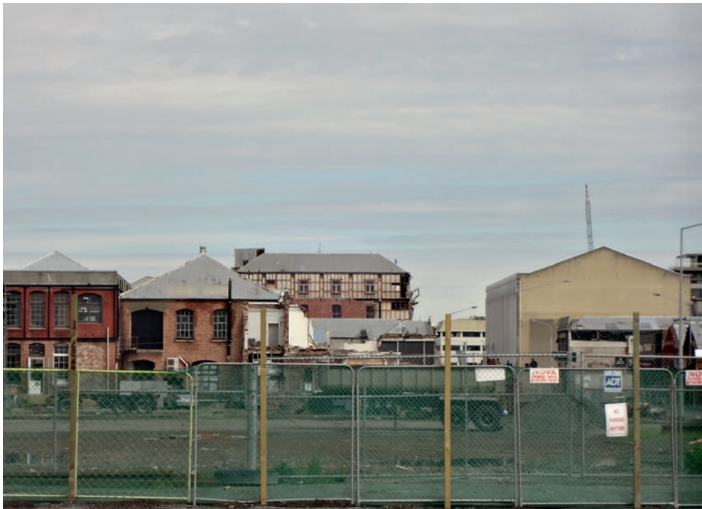
5.18 Buildings in Christchurch cordoned off in the 'red zone' of the city following the 2011 earthquake
