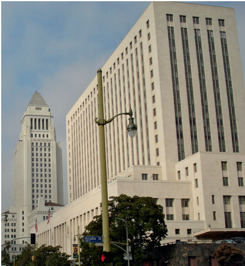
2.12 Oakland City Hall, Oakland, USA, retrofitted 1995
