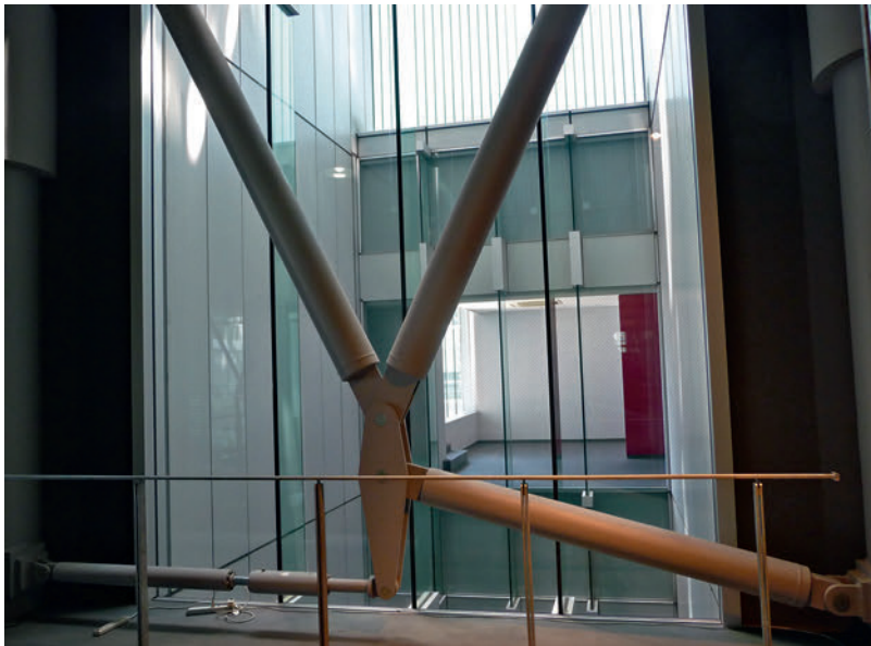
1.5 A damping device on the bottom left incorporated into cross-bracing in the National Museum of Emerging Science and Innovation, Tokyo, Japan
