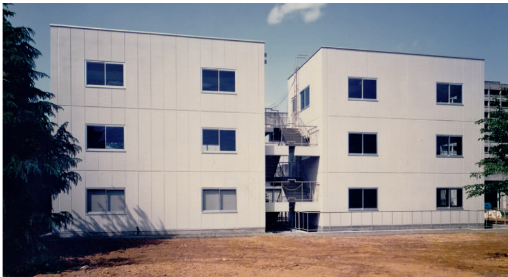
4.4 Two identical buildings, one base-isolated and the other a conventional fixed-base building, at Tōhoku University, Sendai, Japan
