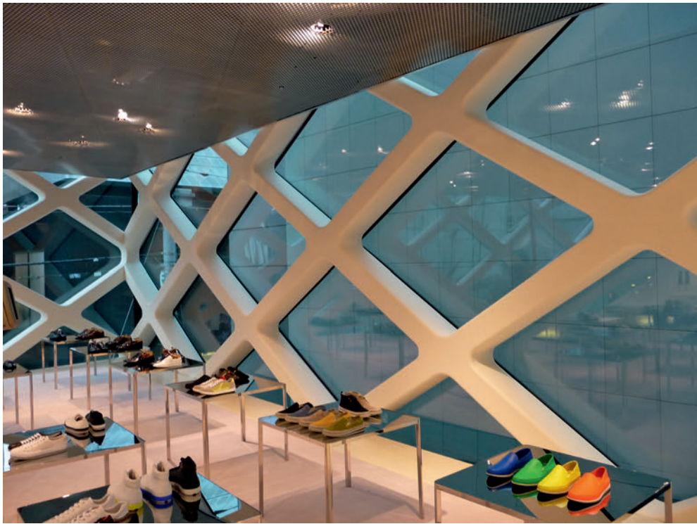
6.18 The structural diagrid wall is most clearly visible from within the building
