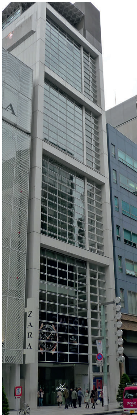
6.20 Nicolas G Hayek Center, Tokyo, Japan. Shigeru Ban Architects. 2006. Front façade
