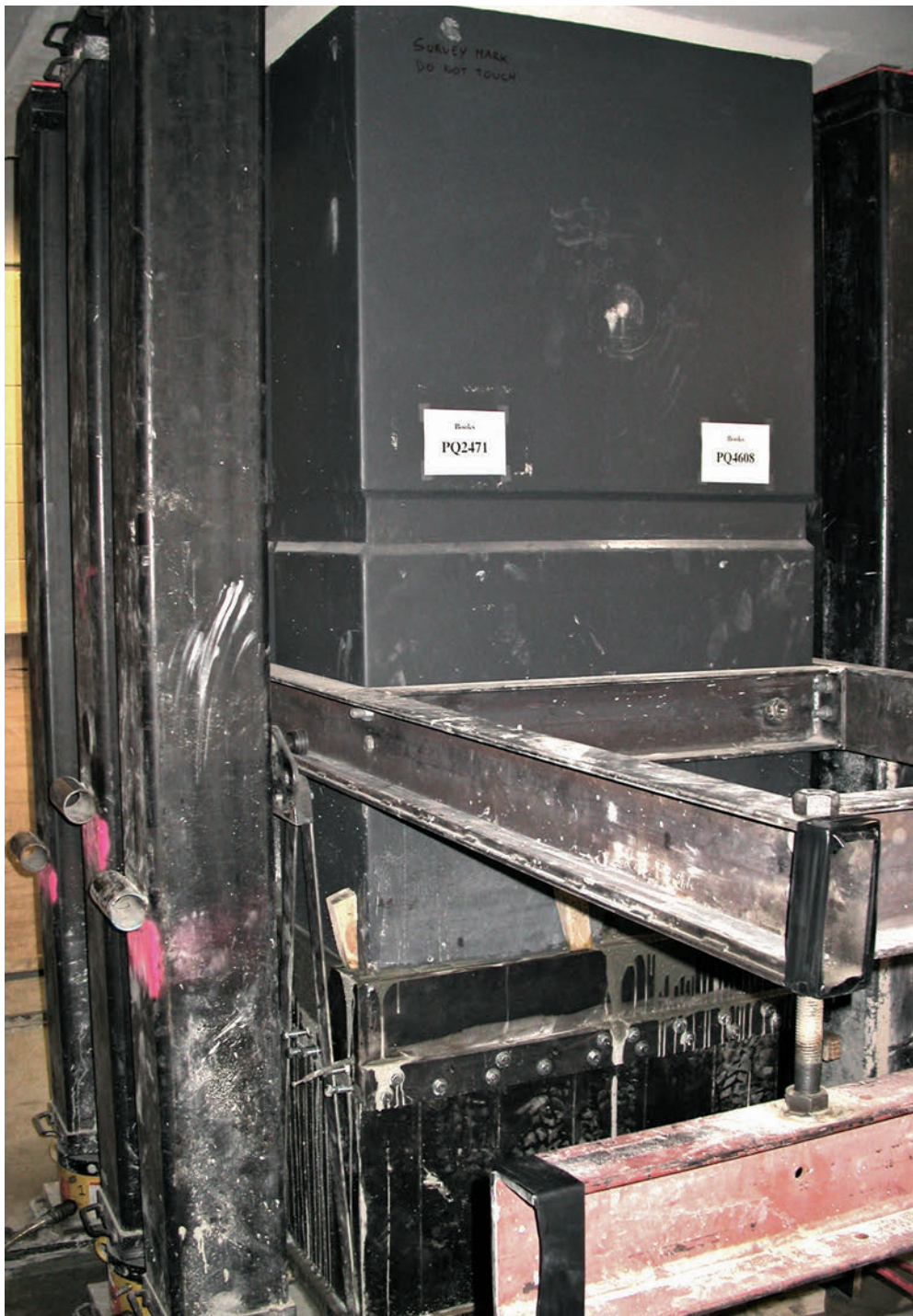
7.17 Three props on each side carry the column load as a new bearing is inserted into the gap cut out of the bottom of the column
