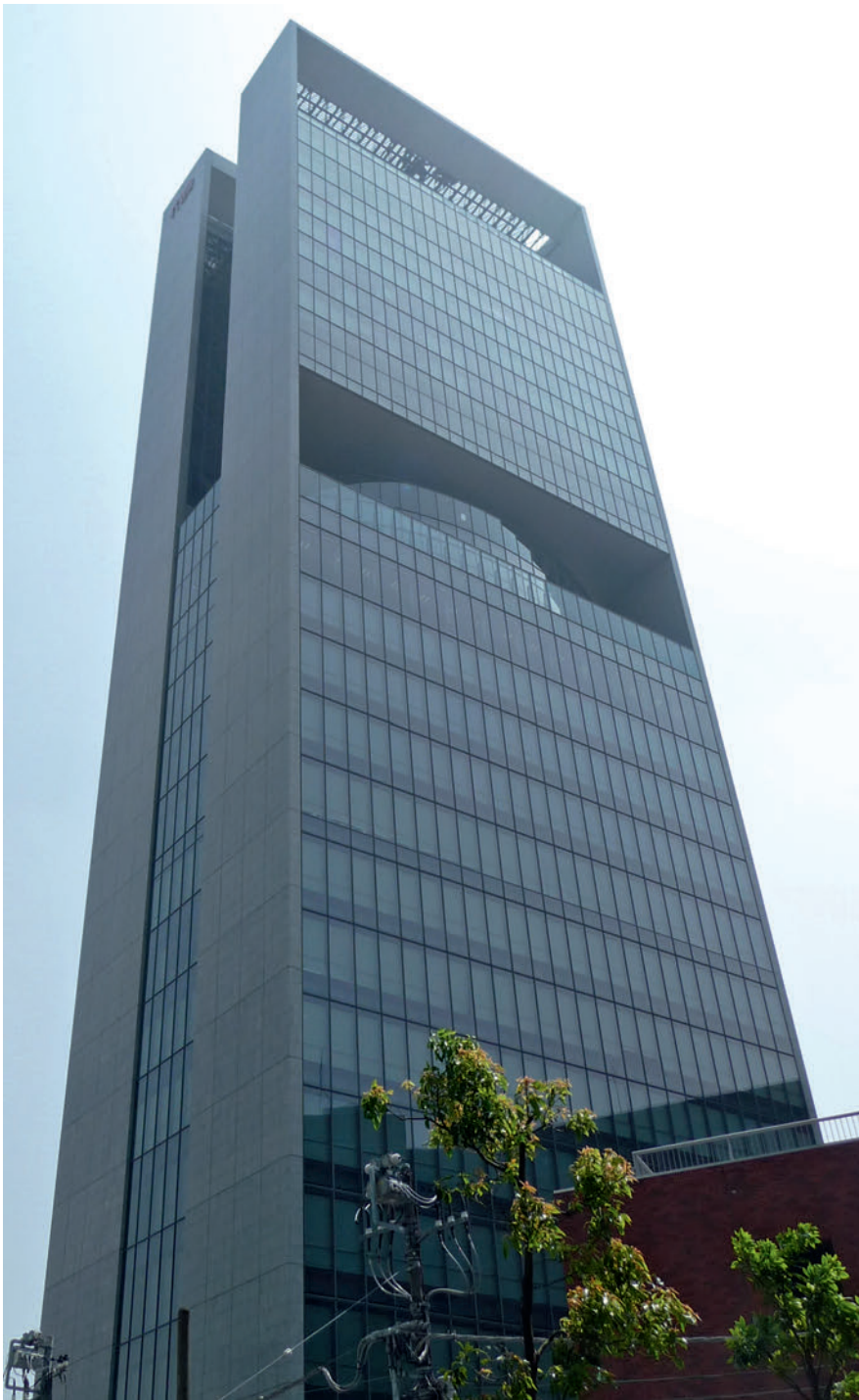
6.26 Yoyogi Seminar School building, also known as the Yozemi Tower, Tokyo, Japan. Taisei Corporation, 2008
