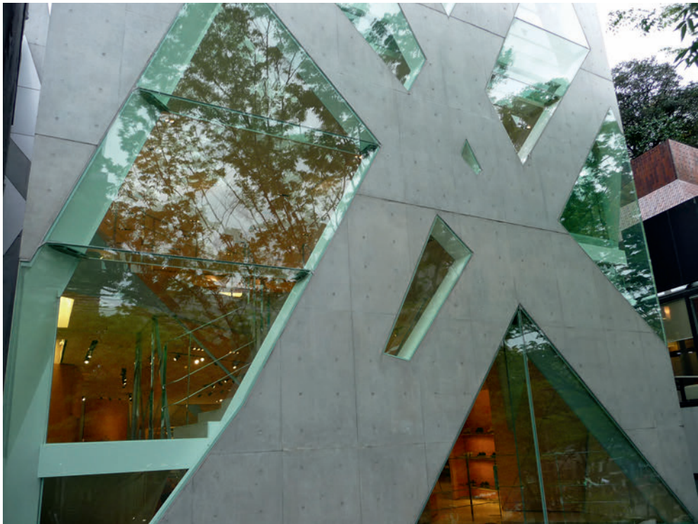
6.2 An area of the front façade
