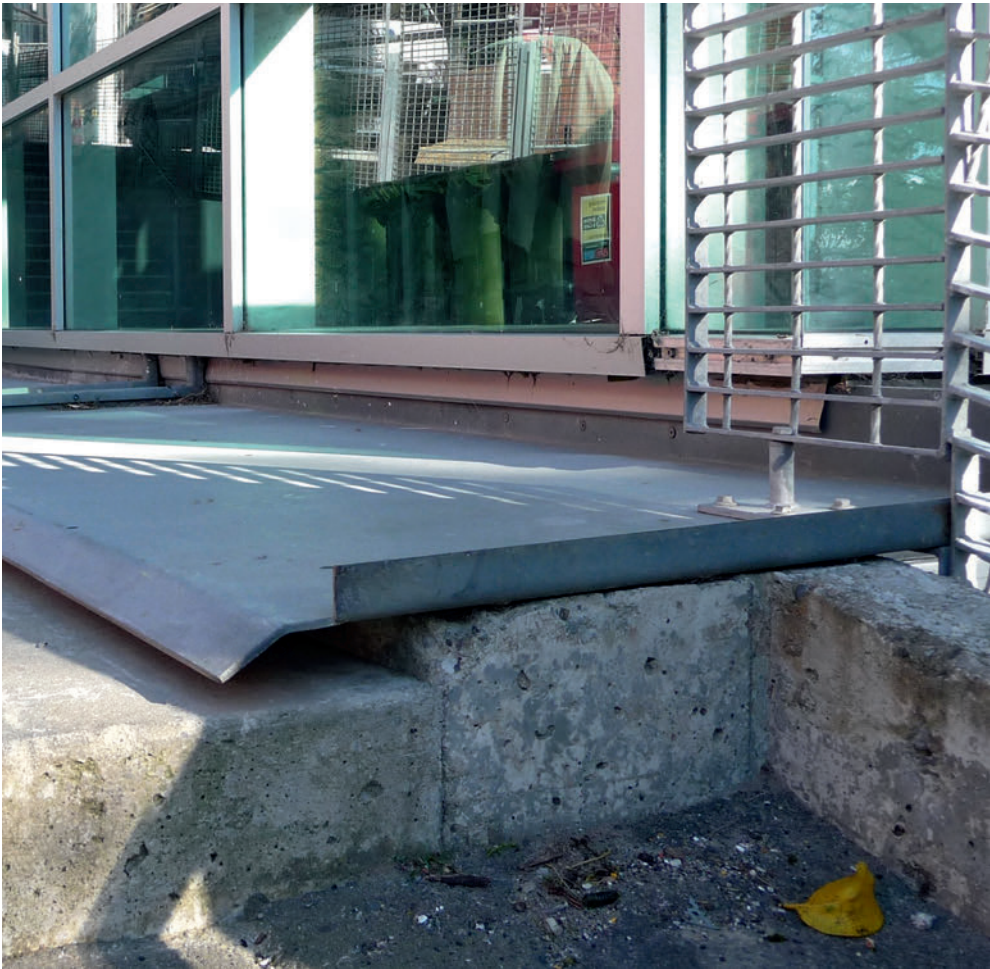
8.10 A steel plate moat cover attached to the isolated building on the right and able to slide over the retaining wall and paving to the left, Wellington, New Zealand
