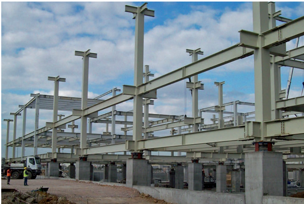
5.6 Sabiha Gökçen International Airport Terminal under construction
