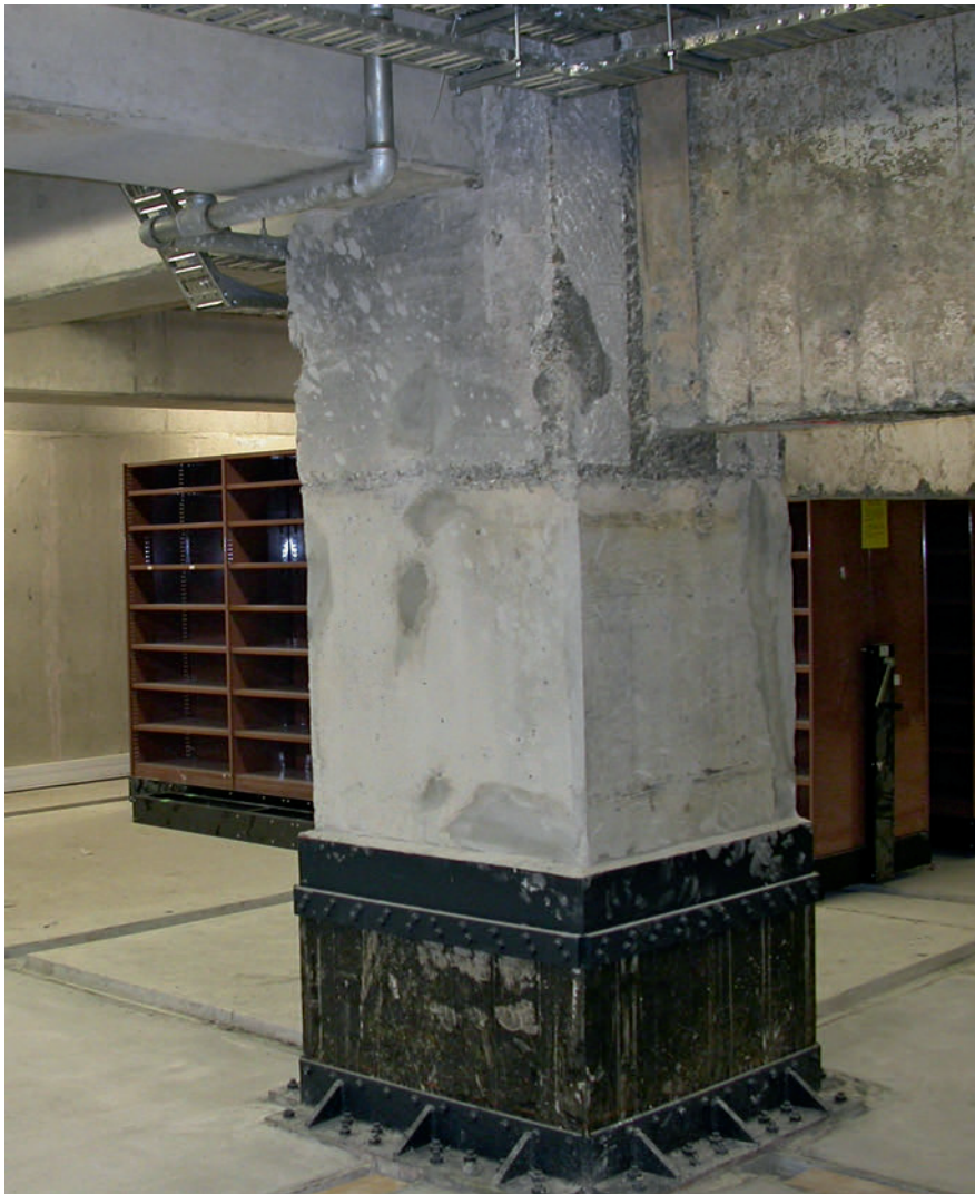
7.18 A column with a new bearing at its base
