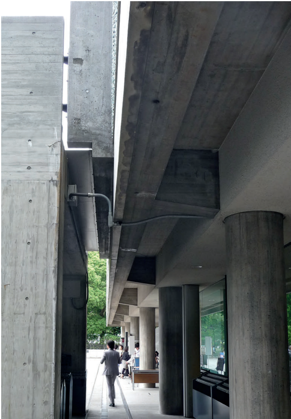
8.6 Horizontal clearance between an external stair to the left and an isolated building to the right, Tokyo, Japan
