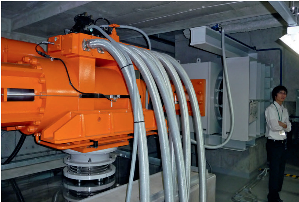
3.21 One of the computer-controlled hydraulic jacks
