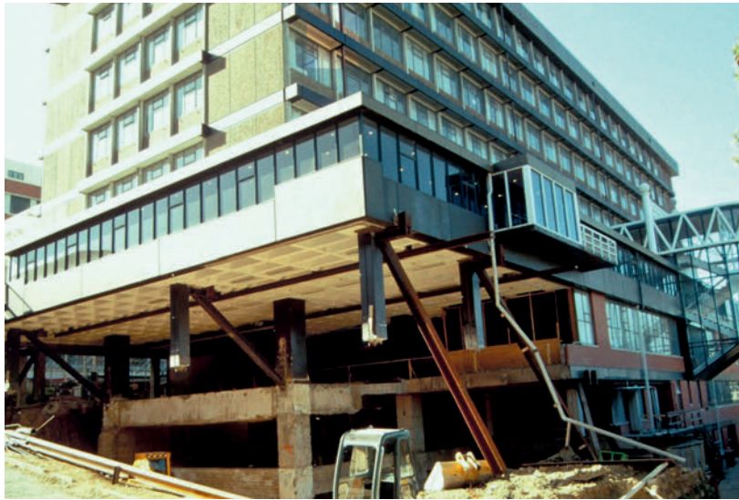
7.16 The propping of the podium during the excavation to existing foundation level
