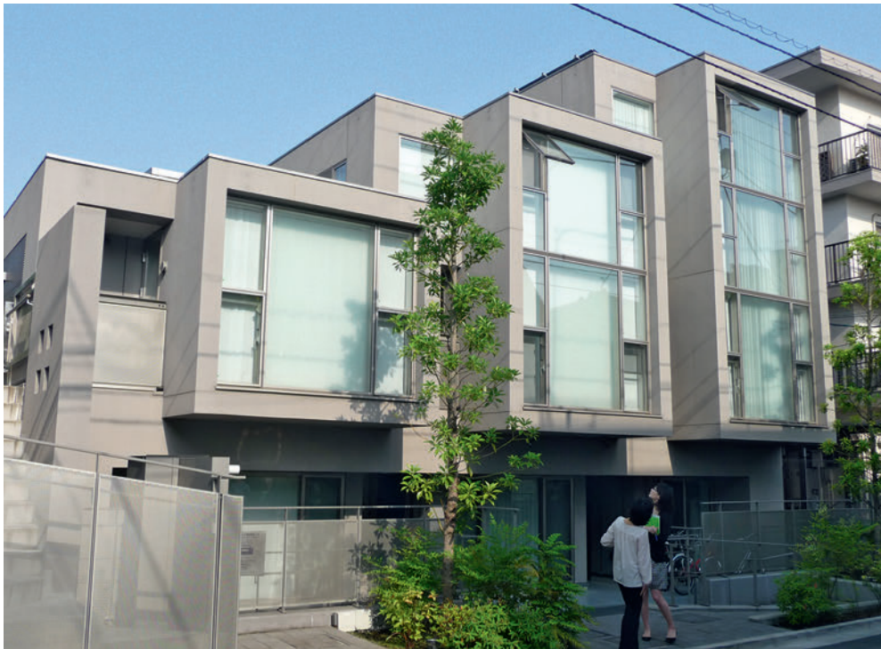
5.11 Chisuikan, Tokyo, Japan, designed by Kozo Keikaku Engineering and completed in 2011, is a housing complex and the first building in the world to be protected by 3-D seismic isolation
