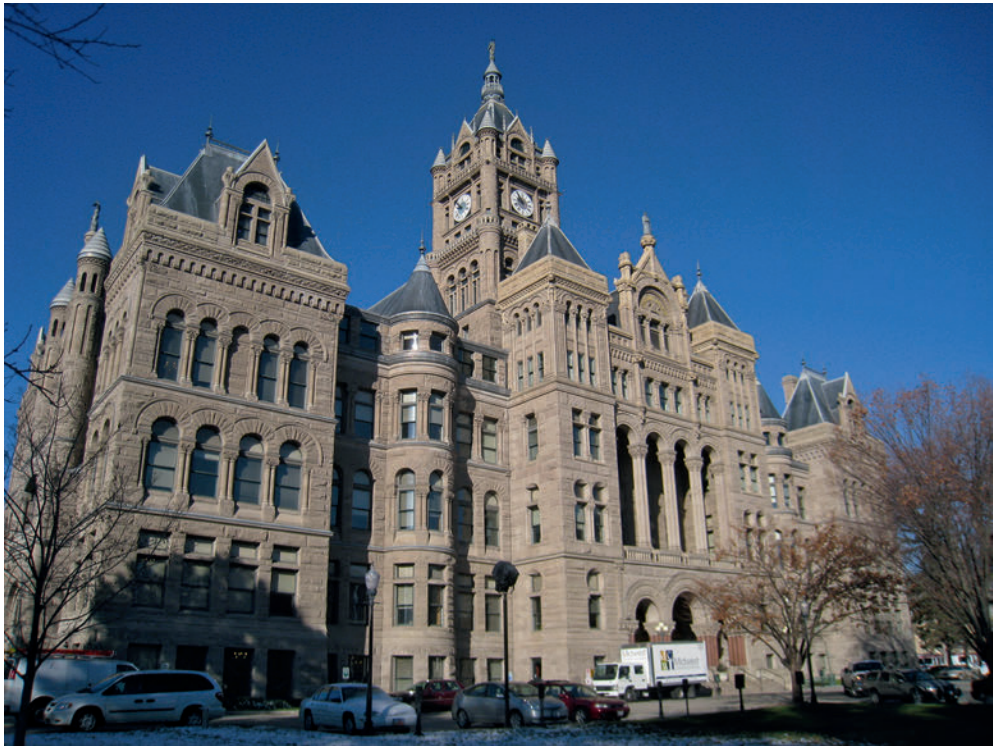
7.1 Salt Lake City and County Building, Utah, USA. The first building to be retrofitted using seismic isolation
