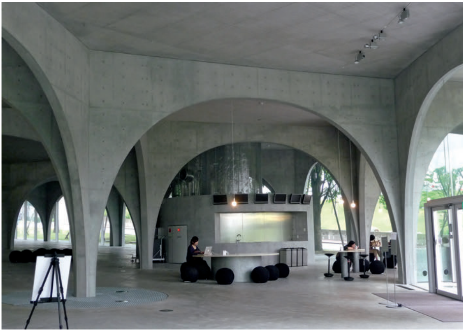
6.5 Interior arches with their fine bases, just inside the main entrance
