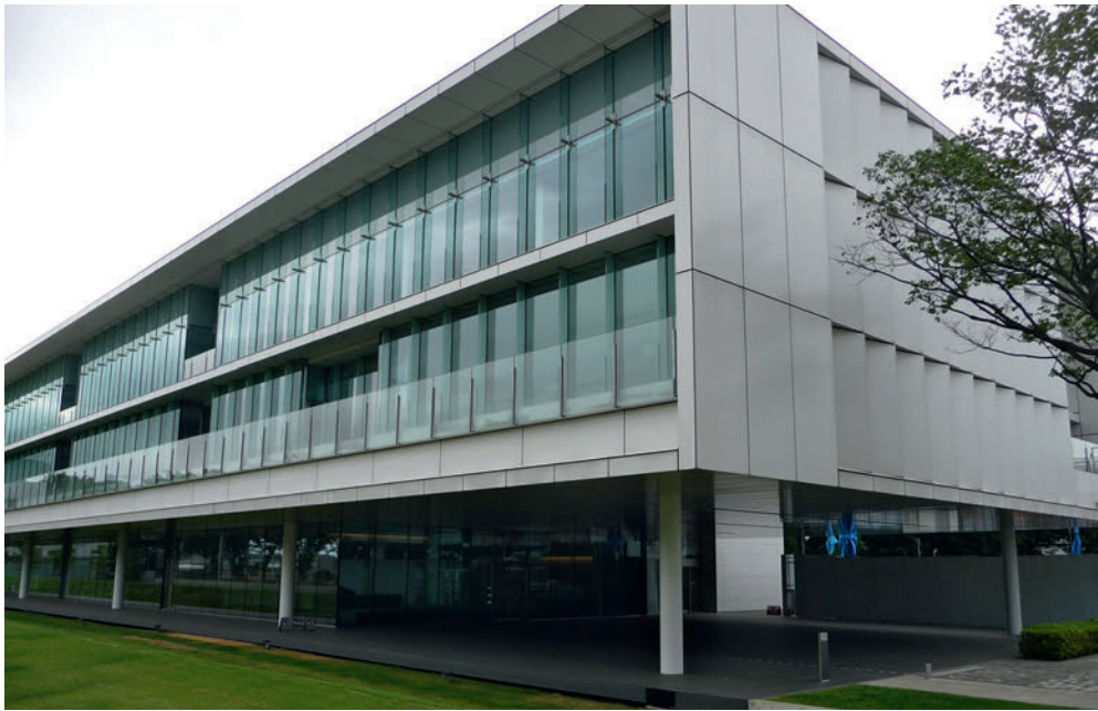
3.20 Technical Research Institute, Obayashi Corporation, Tokyo, Japan. An active isolation system protects the building
