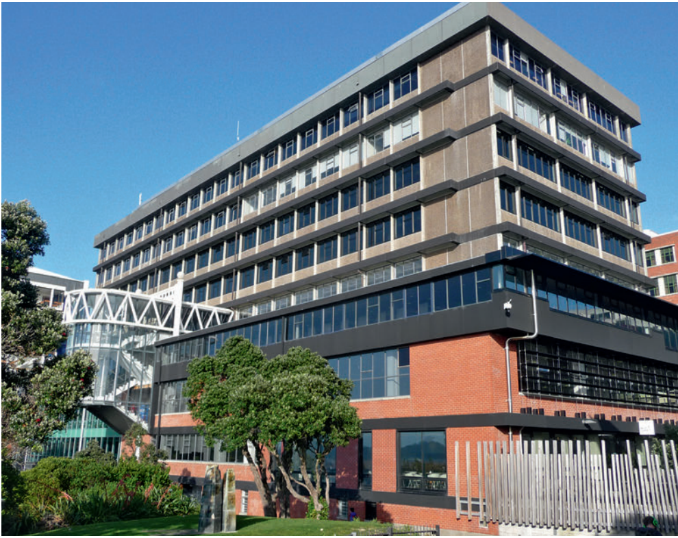
7.14 Rankine Brown Building, Victoria University of Wellington, New Zealand
