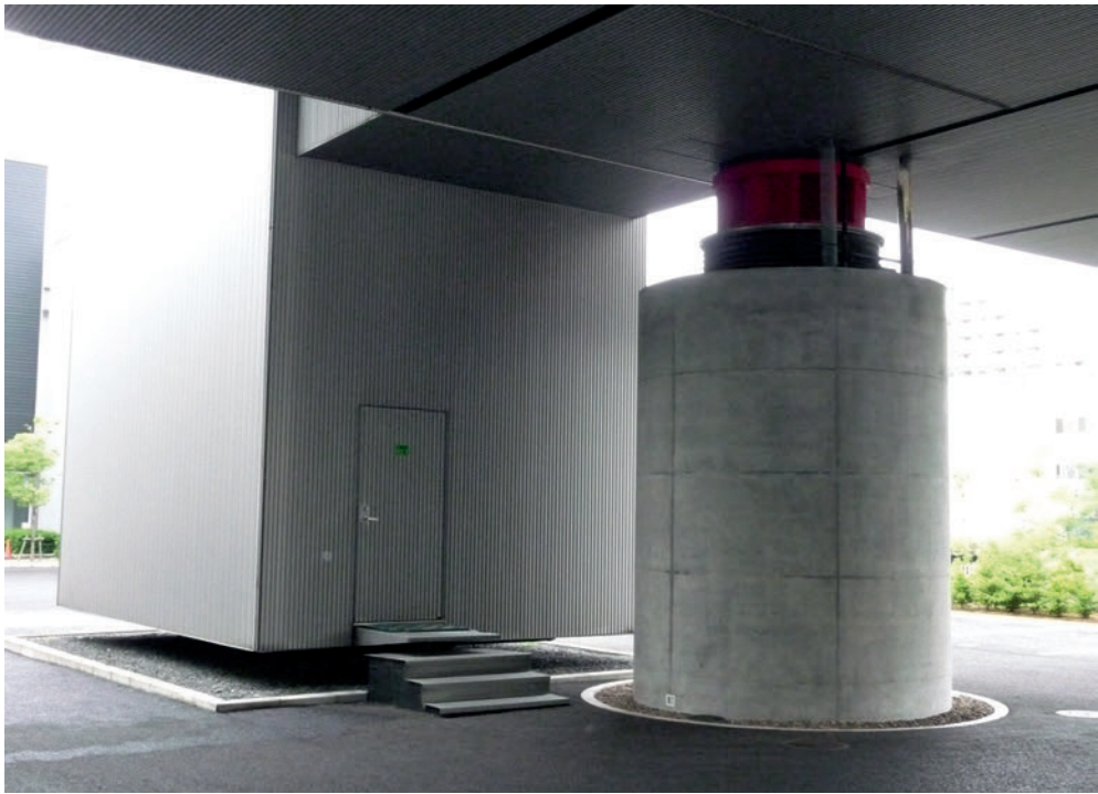
6.8 External escape stair
