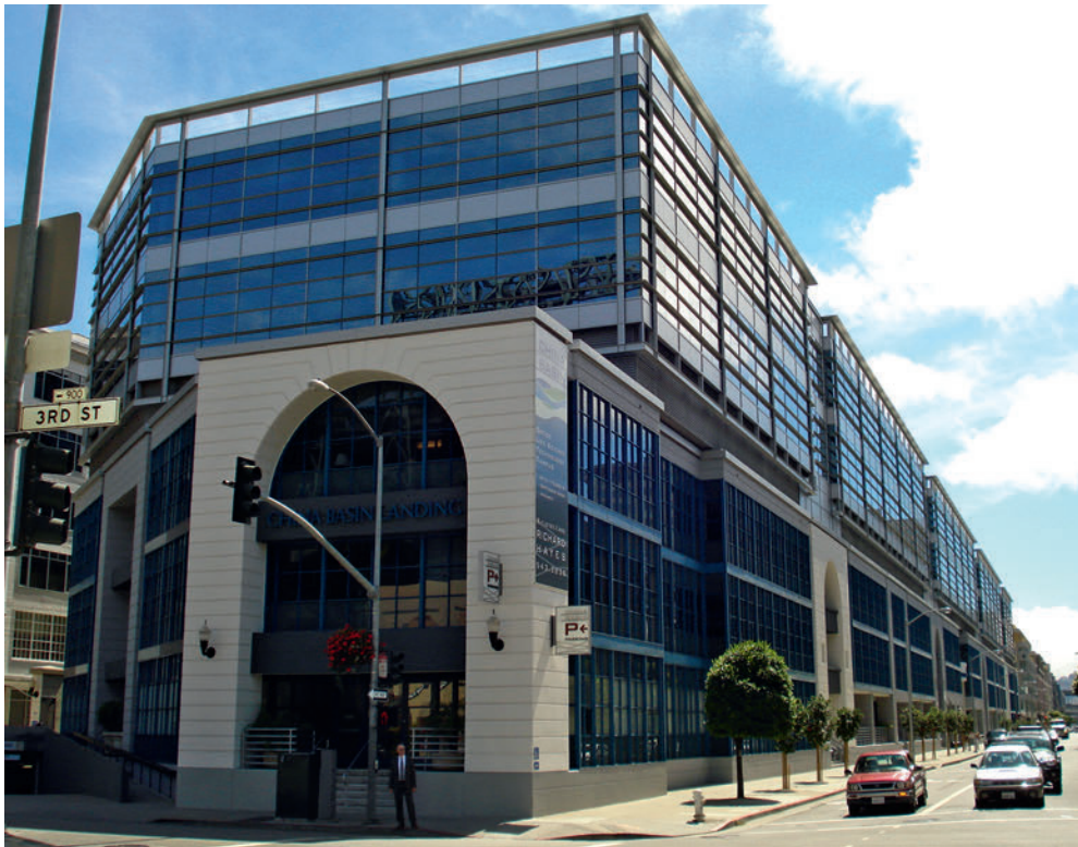
7.25 China Basin Landing office building, San Francisco, USA. The existing three-storey 1980s building was retrofitted by placing isolators at roof level and then constructing another two storeys
