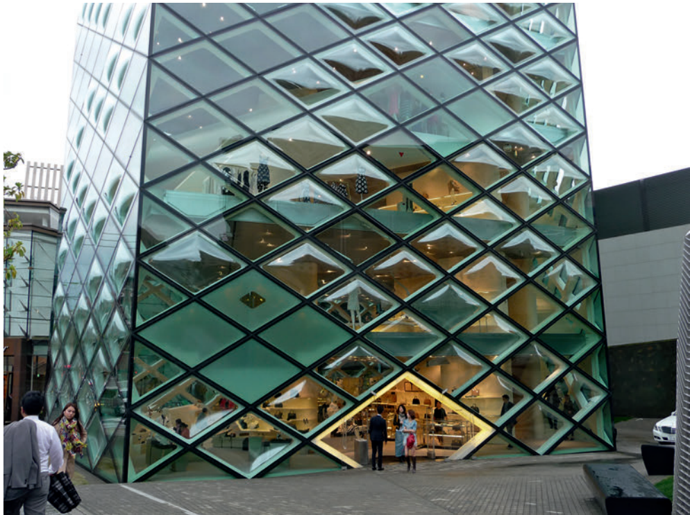
6.17 Prada Boutique Aoyama, Tokyo, Japan, Herzog & de Meuron, 2003. The main entry and the lower floors of the six storeys above ground level. The black glazing lines delineate the diagonal structural members while the floor structure is de-emphasised by a light-colour
