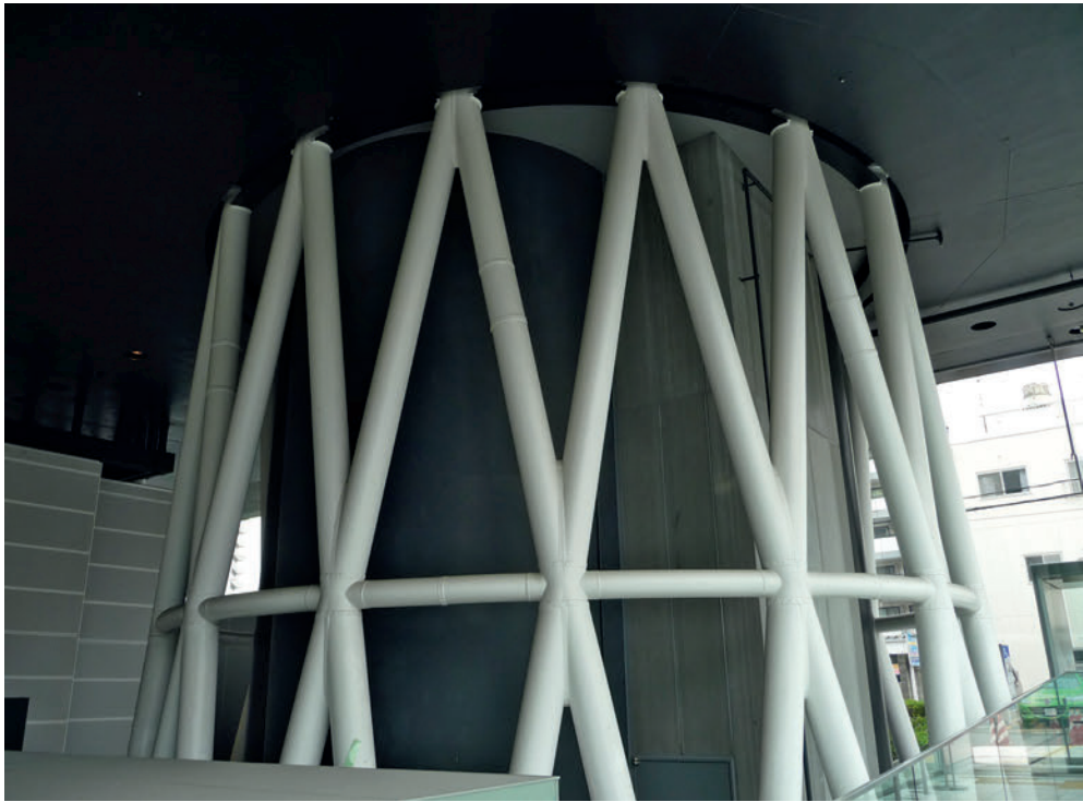
3.16 One of four braced hollow tubes that resist most of the seismic loads acting on the building
