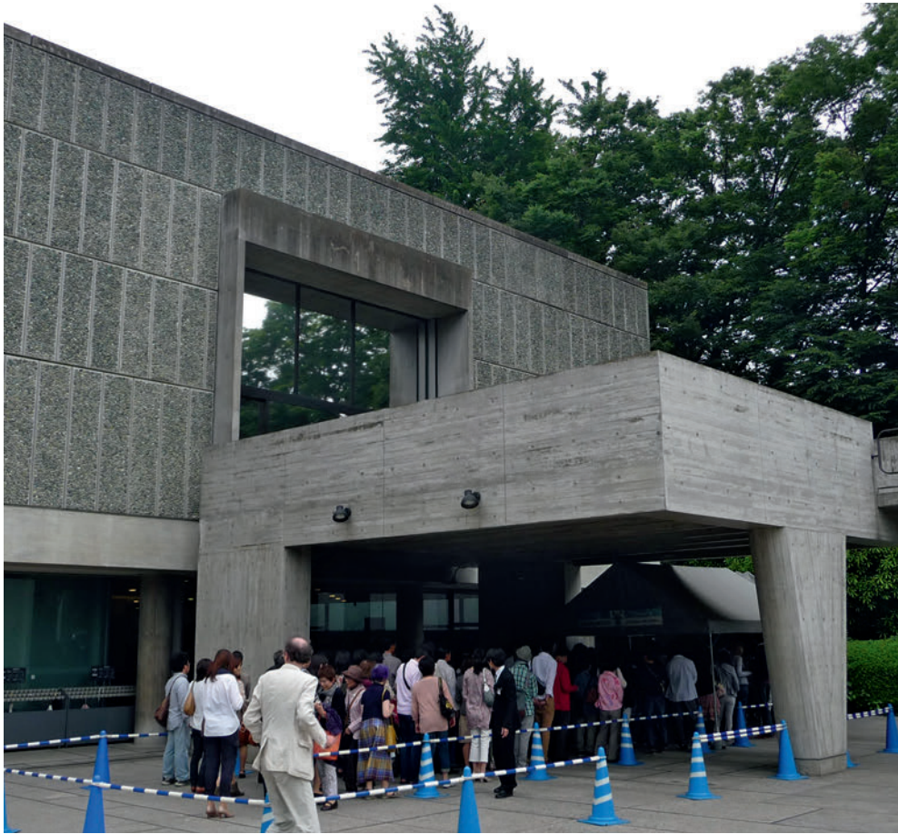
7.24 A seismic separation gap was created between the external stairs and the main building
