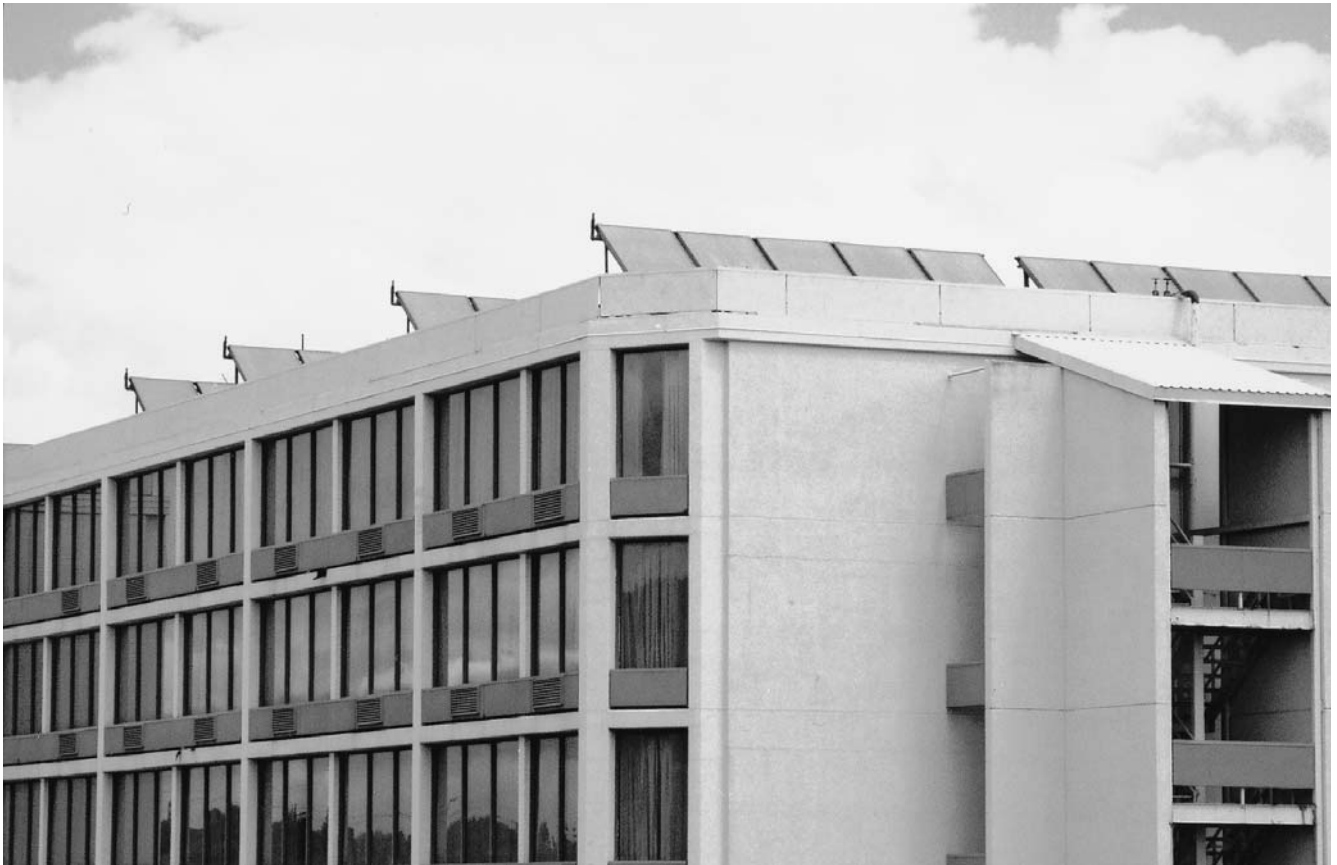
FIGURE 6.14. Hot water for this hotel is heated by the roof-mounted solar collectors. (Photo by Vaughn Bradshaw.)
