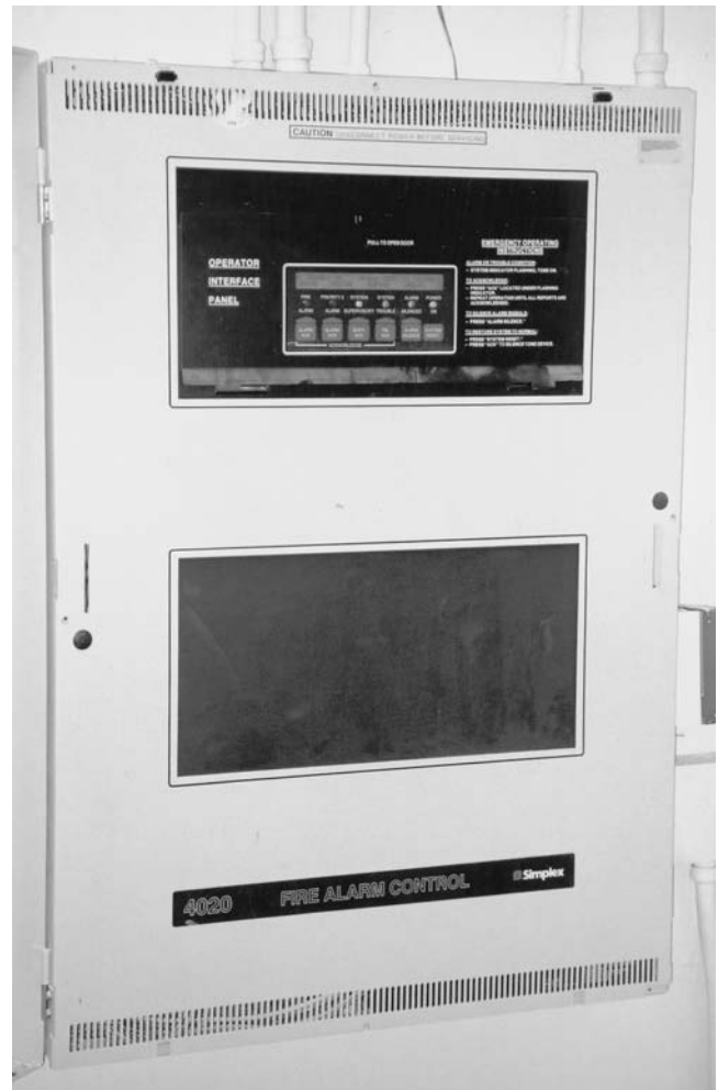
FIGURE 13.3. Fire alarm control panel. (Photo by Vaughn Bradshaw).
