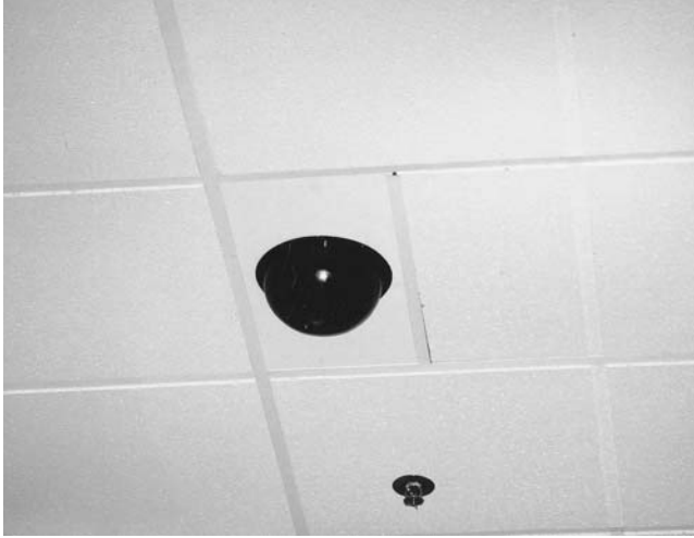
FIGURE 11.5. CCTV security camera. (Photo by Vaughn Bradshaw.)
