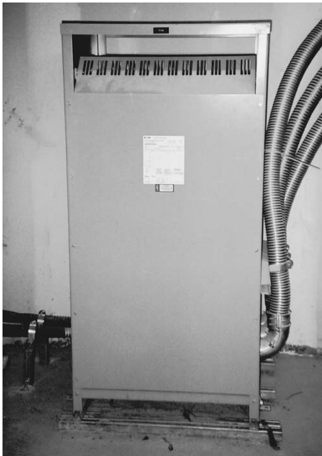
FIGURE 9.6. Indoor 300-kva dry-type transformer. (Photo by Vaughn Bradshaw.)
