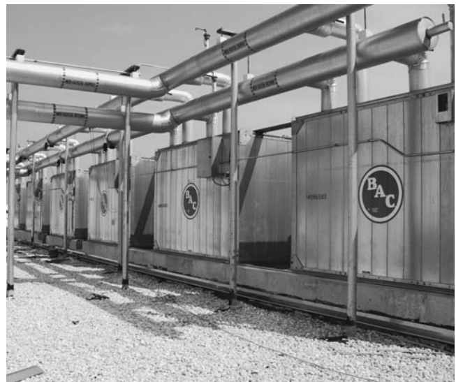
FIGURE 6.20. Cooling towers. (Image courtesy of Trane Commercial Systems.)
