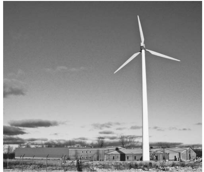
FIGURE 10.8. A 250-kilowatt Fuhrlaender wind turbine at the Harbec Plastics plant in Ontario, New York. The wind power system provides 20 to 25 percent of the company’s electricity requirements and is estimated to pay back its capital investment in 6 to 8 years. (Photo courtesy of Harbec Plastics, Inc., www.harbec.com .)
