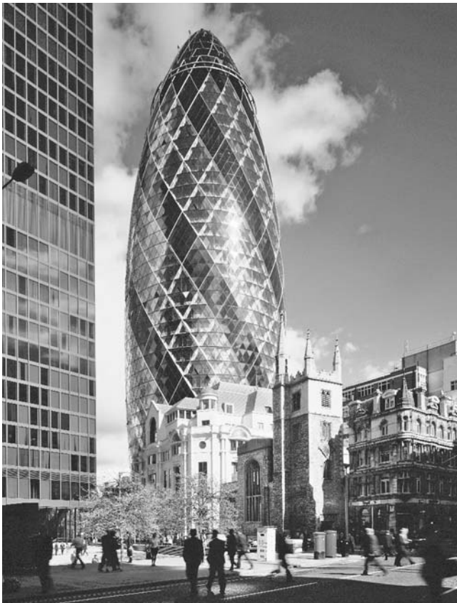
FIGURE 7.17. The Swiss Reinsurance Company's new headquarters—designed by Foster and Partners—is said to be London, England's, first environmentally sustainable skyscraper. It is estimated to use up to 50 percent less energy than a traditionally built office tower of similar size. (Photo courtesy of Nigel Young/Foster and Partners.)
