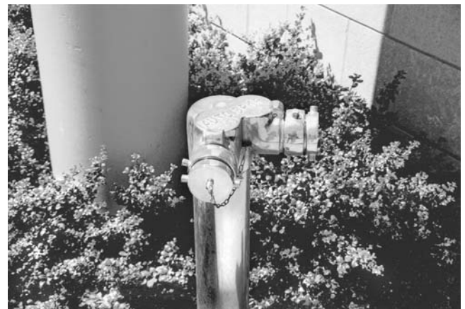
FIGURE 13.15. Siamese outdoor fire department connection. (Photo by Vaughn Bradshaw.)
