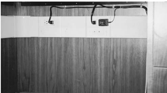
FIGURE 9.12. Surface wireway. For block and brick buildings, a surface-mounted raceway such as this is usually necessary for distribution of power wiring. It can also accommodate signal wiring. (Photo by Vaughn Bradshaw.)
