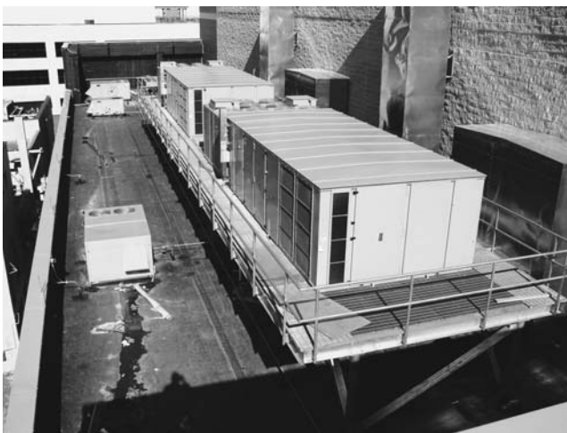
FIGURE 6.28. Unitary RTUs. (Image courtesy of Trane Commercial Systems.)
