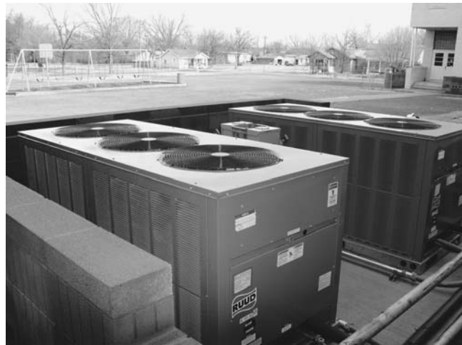
FIGURE 6.21. Air-cooled condensers. (Image courtesy of Trane Commercial Systems.)
