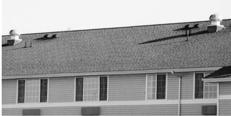
FIGURE 7.15. Wind-driven roof ventilators. (Photo by Vaughn Bradshaw.)
