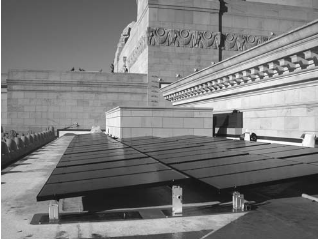
FIGURE 10.10. An array of 144 photovoltaic panels mounted on the state capitol building in Olympia, Washington. The panels generate 20 kilowatts of electricity, enough to light the dome and lantern of the Legislative Building from dusk to midnight every day. To avoid the expense of power storage, the solar-generated electricity is fed into the utility grid to offset the electricity purchased to run the lights in the dome and lantern. The panels—each measuring 63 inches (1.6 m) long and 31 inches (0.79 m) wide—were integrated into this historic building by placing them on the southern side of the fifth-floor roof and positioning them nearly parallel to the horizontal roof surface. Since the array is only about 1 foot (30.5 cm) high, it cannot be seen from the ground or nearby buildings. Concealing the futuristic-looking panels allowed the project to meet federal standards for historic preservation. (Photo courtesy of Michael L. Dean.)
