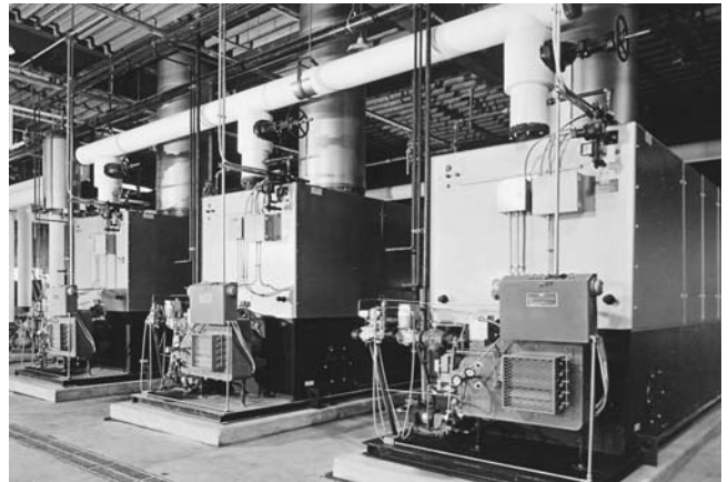
FIGURE 6.8. Watertube boilers providing heat for a 500,000-ft 2 airport terminal. (Photo courtesy of Bryan Steam LLC / Bryan Boilers.)
