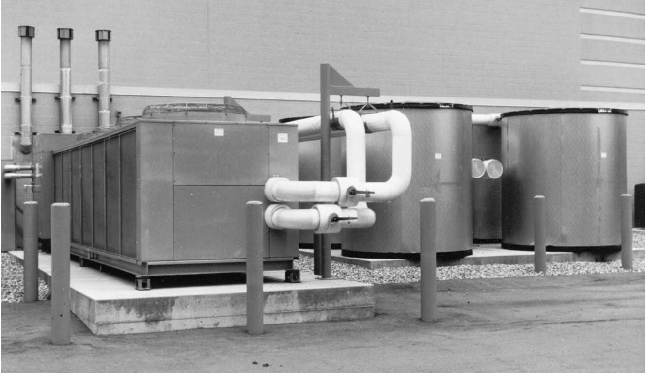
FIGURE 6.42. Ice storage system. The outdoor packaged air-cooled chiller on the left freezes water in the ice storage modules on the right. (Photo courtesy of The Trane Company.)
