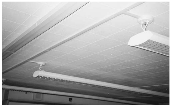
FIGURE 9.13. Surface raceways connecting light fixtures such as these are very helpful in remodel projects. (Photo by Vaughn Bradshaw.)
