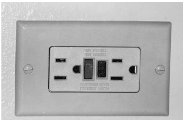
FIGURE 9.17. GFCI receptacle. (Photo by Vaughn Bradshaw.)
