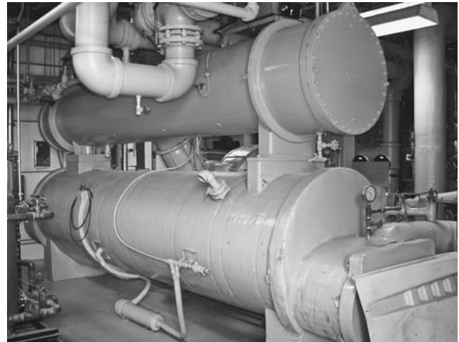
FIGURE 6.17. Indoor absorption chiller. (Image courtesy of Trane Commercial Systems.)
