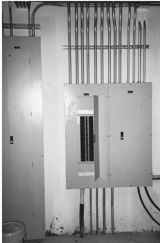
FIGURE 9.7. Panelboard. (Photo by Vaughn Bradshaw.)
