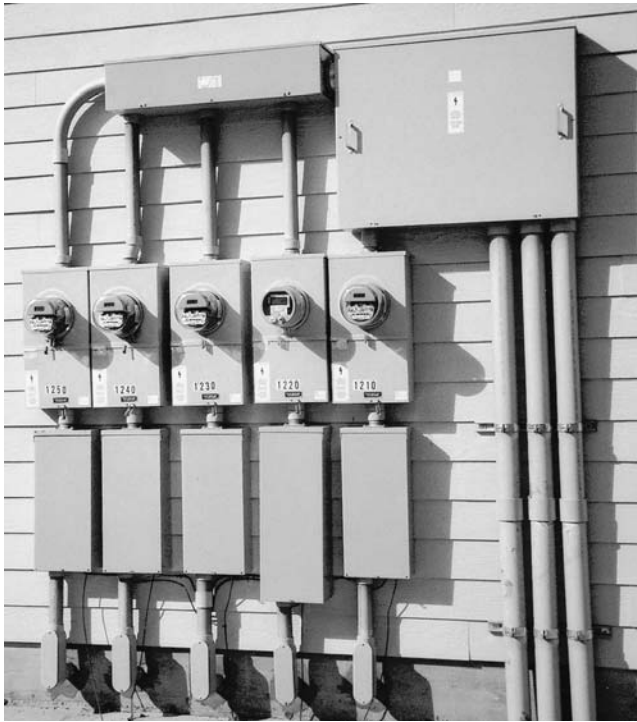
FIGURE 9.10. Meters. (Photo by Vaughn Bradshaw.)
