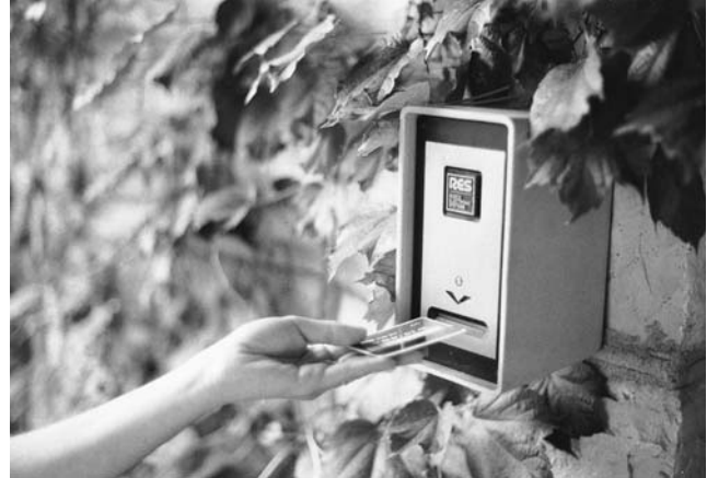
FIGURE 11.8. Access control system ID card reader. (Photo by Vaughn Bradshaw).
