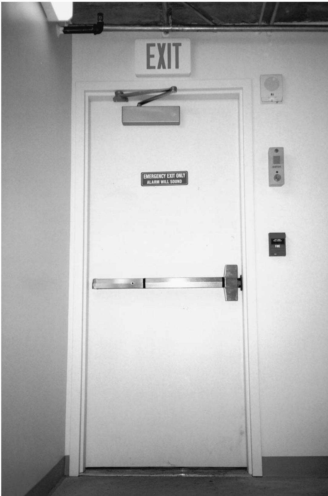
FIGURE 13.5. Panic hardware alarm. (Photo by Vaughn Bradshaw.)
