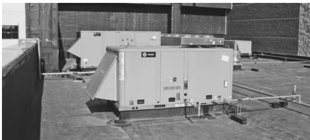
FIGURE 6.29. Gas-fired make-up air unit. (Image courtesy of Trane Commercial Systems.)
