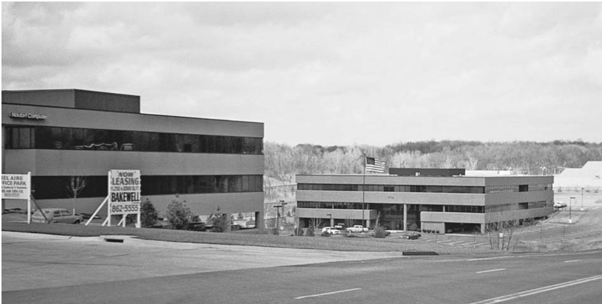
FIGURE 6.1. Rooftop equipment penthouses. (Photo by Vaughn Bradshaw.)
