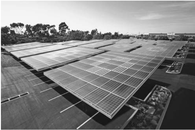
FIGURE 5.9. This “Solar Grove” models the life process of natural trees by converting sunlight into energy without adding carbon dioxide or other greenhouse gases to the atmosphere—while providing structures that are both shade-producing and aesthetically pleasing. The array of 25 “solar trees” converts a 186-vehicle parking lot into a 235-kilowatt solar electric generating system. The carport thus formed over an employee parking lot at the Kyocera North American headquarters in San Diego, California, utilizes a total of 1,400 Kyocera solar photovoltaic (PV) modules tilted slightly to maximize solar exposure. This installation is capable of generating 421,000 kilowatt-hours per year. According to the U.S. EPA, generating this amount of electricity from fossil fuel resources would annually release nearly 340,000 pounds of carbon dioxide, a contributor to global warming; 420 pounds of nitrous oxide, which has been linked to the destruction of the earth’s ozone layer; and 250 pounds of sulfur dioxide, the principal contributor to acid rain. (Photo courtesy of KYOCERA Solar, Inc.)
