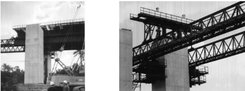
FIGURE 19.27 Mobile scaffolding for approach viaduct of the West Portion.
