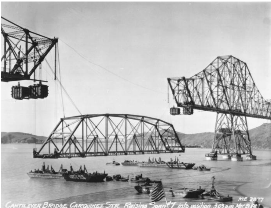
FIGURE 1.20 Raising of suspended span, Carquinez Strait Bridge, California, 1927. The 433 ft. (132 m) suspended span, weighting 650 tons, was raised into position in 35 min., driven by four counterweight boxes having a total weight of 740 tons.
