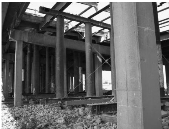
FIGURE 3.5 Falsework at I-680/24 Interchange South-East connector, Walnut Creek.
