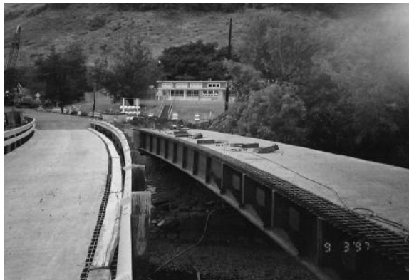
FIGURE 7.14 Use of modular system and concrete-filled grid deck for accelerated bridge construction staged construction. Sequence: Built first half adjacent to existing structure and switched traffic over to new; demolished existing structure and built second half. Skidded two sections together and completed with a closure pour.
