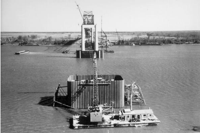
FIGURE 6.15 An open caisson positioned within steel jackets on pens.
