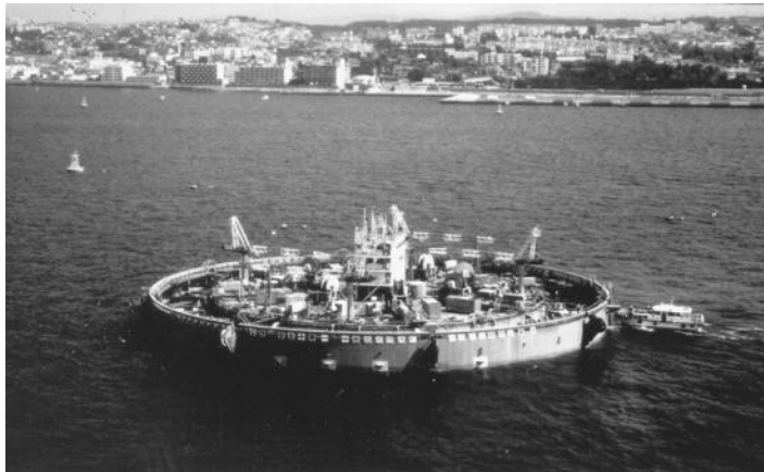
FIGURE 6.20 The Akashi Strait Suspension Bridge is founded on steel box caissons filled with tremie concrete.
