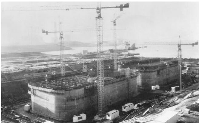
FIGURE 6.23 Large concrete box caissons fabricated in the construction basin for subsequent deployment to site by self-flotation, Great Belt Eastern Bridge.
