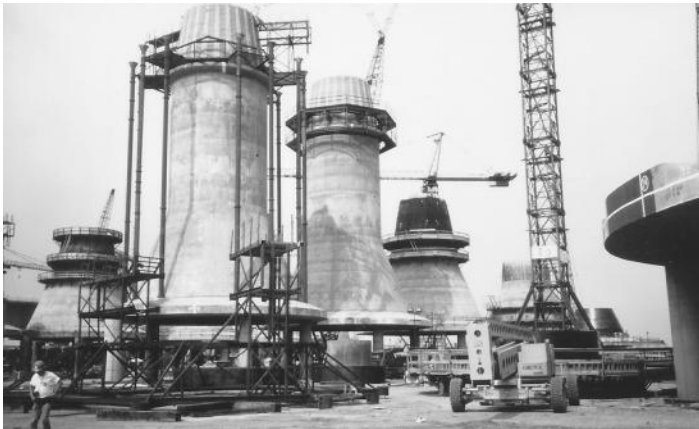
FIGURE 6.25 Prefabrication of pier bases for the Prince Edward Island Bridge.
