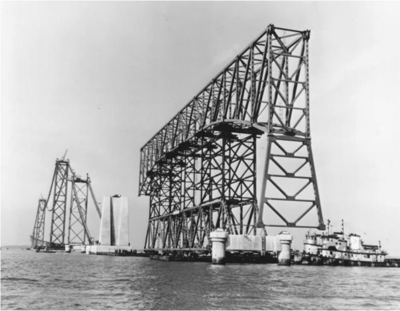
FIGURE 1.31 Floating-in erection of a truss span, first Chesapeake Bay Bridge, Maryland, 1952. A 480 ft. (146 m) truss span, weighting 850 tons, supported on falsework consisting of a permanent deck-truss span along with temporary members, is being floated-in for landing onto its piers. Suspension bridge cables are under construction in background. (Courtesy of Bethlehem Steel Corporation.)
