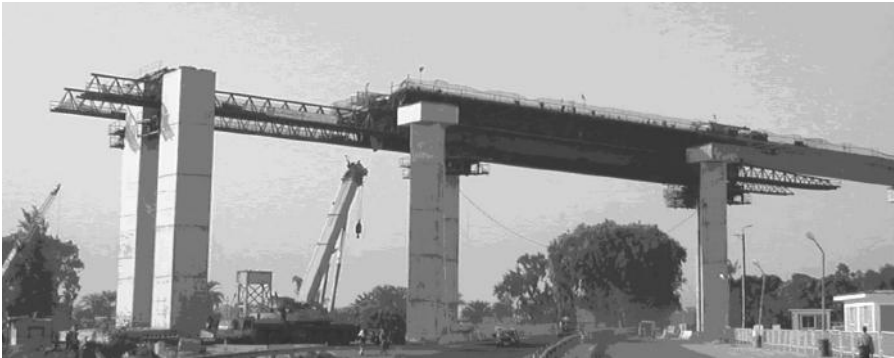
FIGURE 19.26 Construction of the approach viaduct in the West Portion (Nov. 99).
