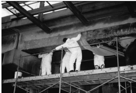
FIGURE 16.26 Glass fiber-reinforced polymer fabric to strengthen deteriorated reinforced concrete T-beam. (Courtesy of FHWA.)
