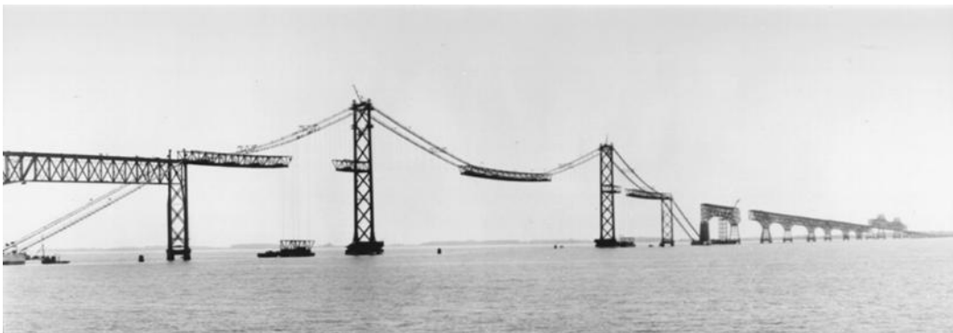
FIGURE 1.6 Suspension spans of first Chesapeake Bay Bridge, Maryland, 1952. Deck steelwork is under erection and is about 50% complete. A typical four-panel through-truss deck section, weighing about 100 tons, is being picked in west side span, and also in east side span in distance. Main span is 1600 ft. (488 m) and side spans are 661 ft. (201 m); towers are 324 ft. (99 m) high. Cables are 14 in. (356 mm) in diameter and are made up of 61 helical bridge strands each (see Figure 1.8).
