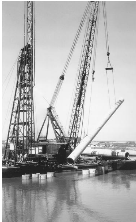
FIGURE 6.6 A large-diameter prestressed concrete pile for Napa River Bridge, California.
