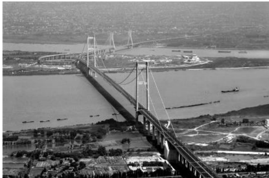
FIGURE 4.4 Runyang Bridge ( http://civil.seu.edu.cn/s/321/t/1688/a5/2f/info42287.htm ).
