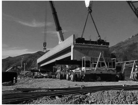
FIGURE 7.12 Full superstructure I-215 east over 3760 south being lifted into place by cranes.
