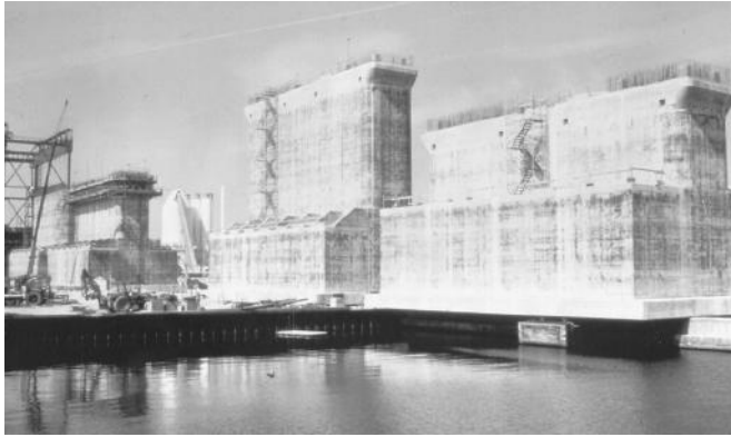
FIGURE 6.22 Prefabricated concrete box caissons are moved by jacks onto a pier for load-out.
