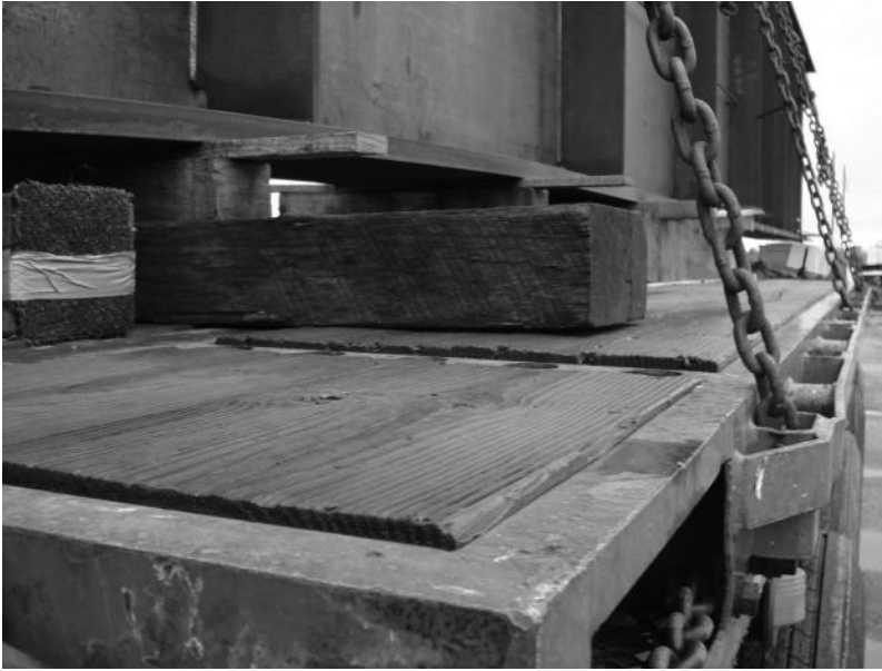
FIGURE 2.10 Trucking is the most common approach used for shipping steel girders.
