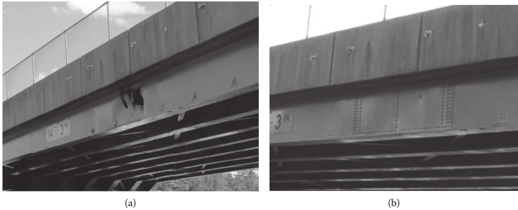
FIGURE 16.24 Repair and strengthening of steel girder web damage by vehicle impact: (a) damaged girder, (b) repaired girder.
