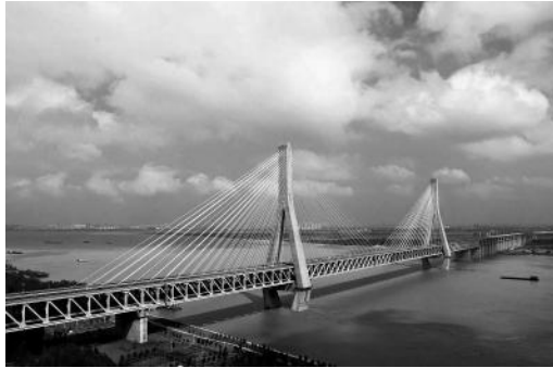
FIGURE 4.1 Tianxingzhou Bridge. (Courtesy of Wuhan Urban and Rural Construction Committee, http://online.whjs.gov.cn/node/node_545.htm .)
