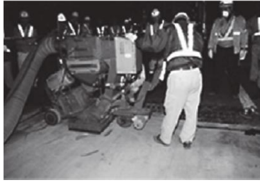
(2) Applying shot blast machine
