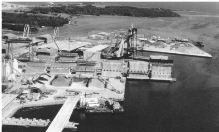
FIGURE 6.21 Prefabrication of box caisson piers for the Great Belt Western Bridge.
