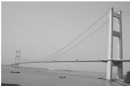
FIGURE 4.5 Jiangyin Bridge ( http://www.cots.com.cn/JingDian/JiangYinChangJiangDaQiao.html ).
