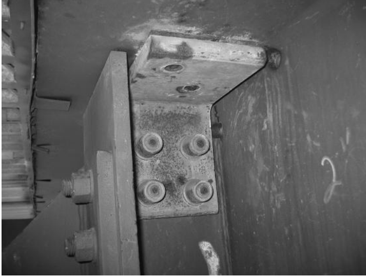
FIGURE 14.10 An unsuccessful repair of distortion-induced fatigue using Huck bolts.
