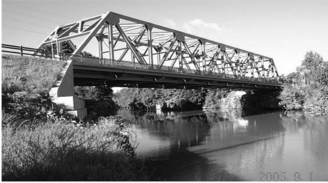
FIGURE 11.3 Through truss bridge. (Courtesy of the New York State Department of Transportation.)
