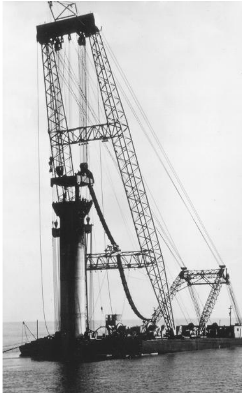
FIGURE 6.8 Installing a concrete cylinder pile by internal excavation, jetting, and pull-down force from a barge.
