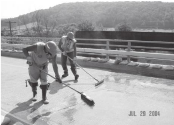
Spreading the polymer material
