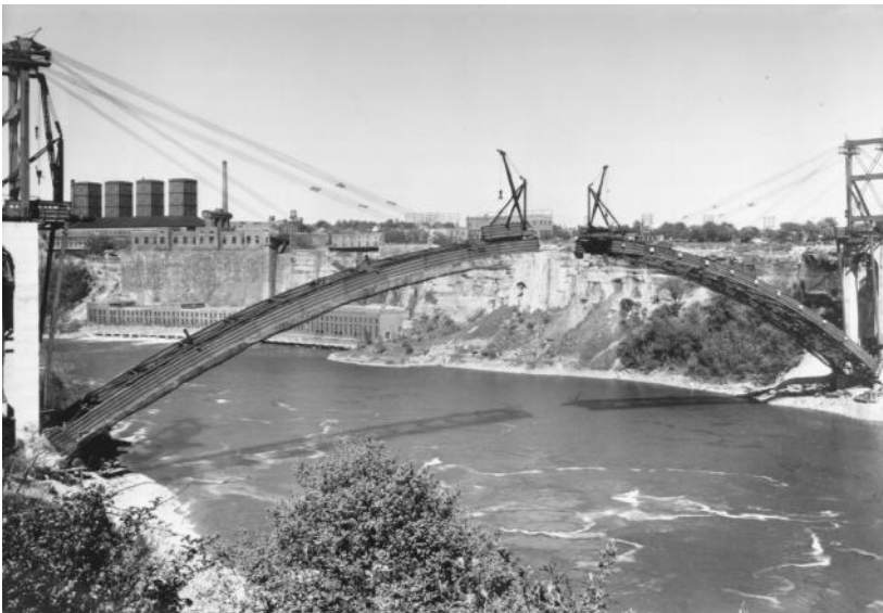
FIGURE 1.2 Erection of arch ribs, Rainbow Bridge, Niagara Falls, New York, 1941. Bridge span is 950 ft. (290 m), with rise of 150 ft. (46 m); box ribs are 3 \times 12 ft. ( 0.91 \times 3.66 m). Tiebacks were attached starting at the end of the third tier and jumped forward as erection progressed (see Figure 1.3). Much permanent steelwork was used in tieback bents. Derricks on approaches load steelwork onto material cars that travel up arch ribs. Travelers are shown erecting last full-length arch-rib sections, leaving only the short, closing crown sections to be erected. Canada is at right, the United States at left. (Courtesy of Bethlehem Steel Corporation.)
