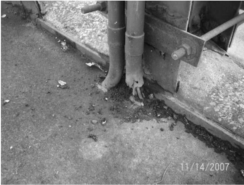
FIGURE 11.14 Safety Flag due to exposed wiring. (Courtesy of the New York State Department of Transportation.)
