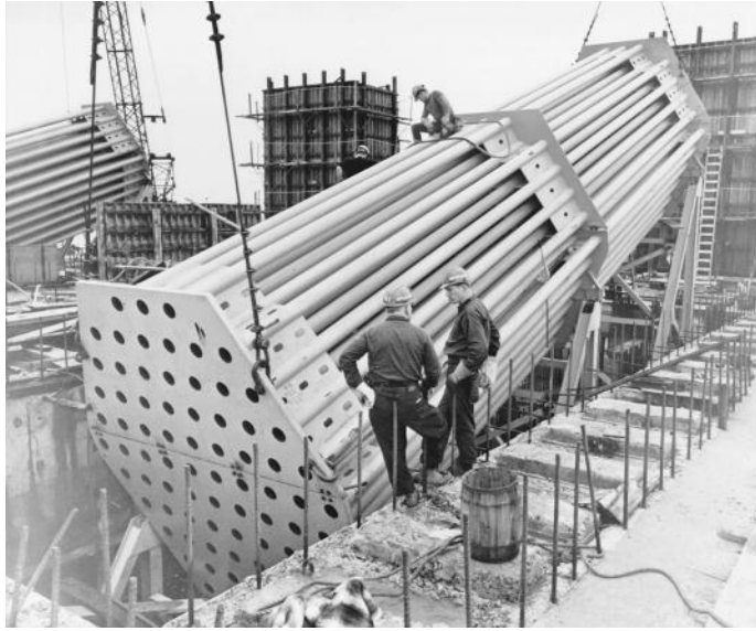
FIGURE 1.38 Pipe-type anchorage for parallel-wire-strand (PWS) cables, Newport Bridge suspension spans, Nar ragansett Bay, R.I., 1967. Pipe anchorages shown will be embedded in anchorage concrete. Socketed end of each PWS is pulled down its pipe from upper end, then seated and shim-adjusted against heavy bearing plate at lower end. Pipe-type anchorage is much simpler and less costly than standard anchor-bar type used with aerial-spun parallel-wire cables (see Figure 1.25B). (Courtesy of Bethlehem Steel Corporation.)
