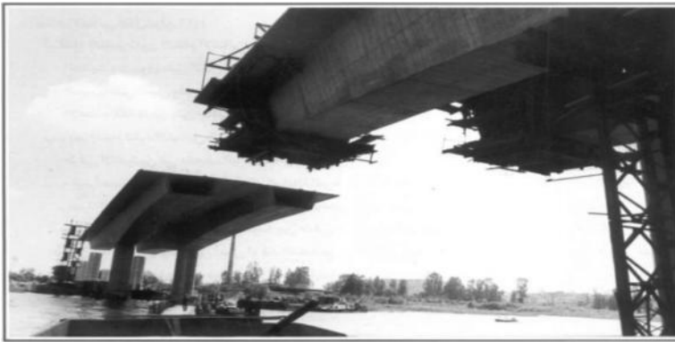
FIGURE 19.32 Casting of segment (Rod El-Farag Bridge).
