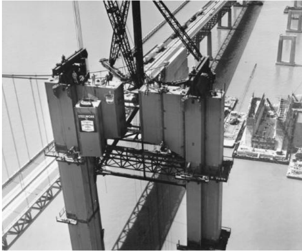
FIGURE 1.35 Tower erection, second Delaware Memorial Bridge, Wilmington, Del., 1966. Tower erection traveler has reached topmost erecting position and swings into place 23-ton closing top-strut section. Tower legs were jacked apart about 2 in. (50 mm) to provide entering clearance. Traveler jumping beams are in topmost working position, above cable saddles. Tower steelwork is about 418 ft. (127 m) high. Cable anchorage pier is under construction at right. First Delaware Memorial Bridge (1951) is at left. The main span of both bridges is 2150 ft. (655 m). (Courtesy of Bethlehem Steel Corporation.)
