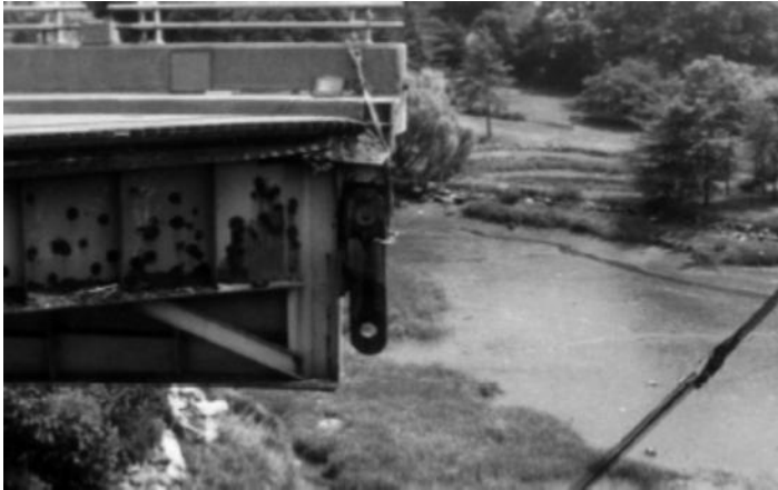
FIGURE 16.4 Pin-and-hanger assembly failure of Mianus Bridge over I-95. (Courtesy of FHWA, 1984.)
