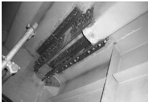
FIGURE 17.20 Partial replacement of longitudinal rib.
