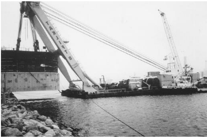
FIGURE 6.29 Lifting a box caisson from the quay wall on which it was prefabricated and transporting it to site while being suspended from the crane barge.
