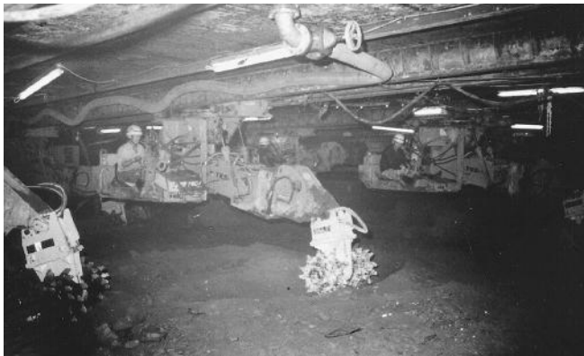
FIGURE 6.17 Excavating within the pressurized working chamber of the pneumatic caisson for the Rainbow Suspension Bridge. (Courtesy of Shiraishi Corporation, Japan.)
