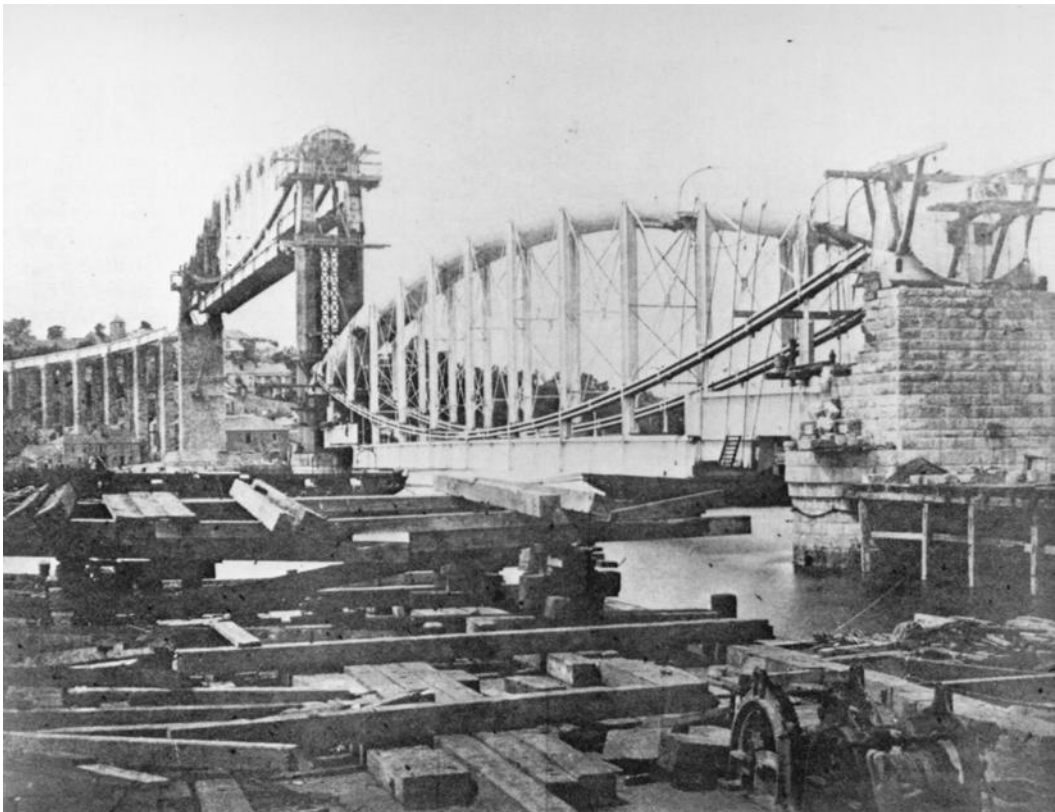
FIGURE 1.14 Royal Albert Bridge across River Tamar, Saltash, England, 1857. The two 455 ft. (139 m) main spans, each weighing 1060 tons, were constructed on shore, floated out on pairs of barges, and hoisted about 100 ft. (30 m) to their final position using hydraulic jacks. Pier masonry was built up after each 3 ft. (1 m) lift.
