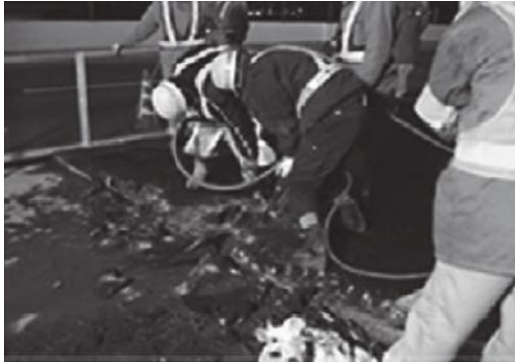
(1) Strip pavement off
