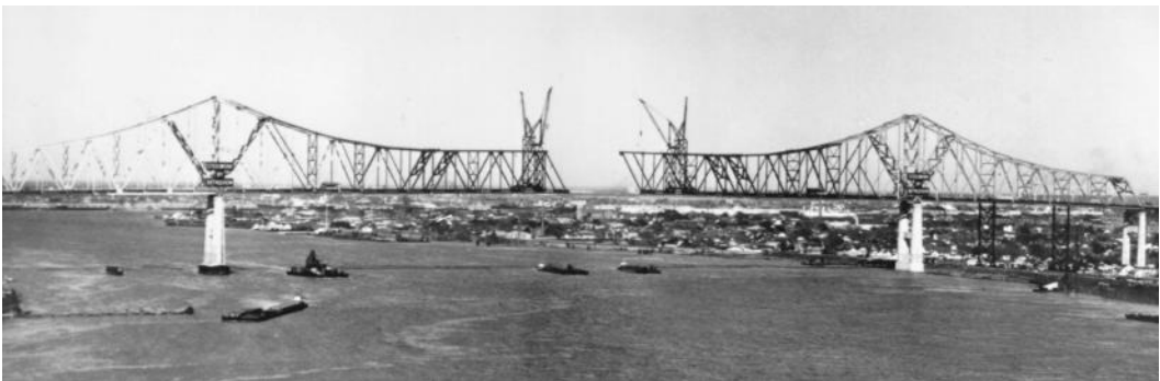
FIGURE 1.34 Greater New Orleans cantilever bridge, Louisiana, 1957. Tall double-boom deck travelers started at ends of main bridge and erected anchor spans on falsework, then the 1575 ft. (480 m) main span by cantilevering to midspan. (Courtesy of Bethlehem Steel Corporation.)
