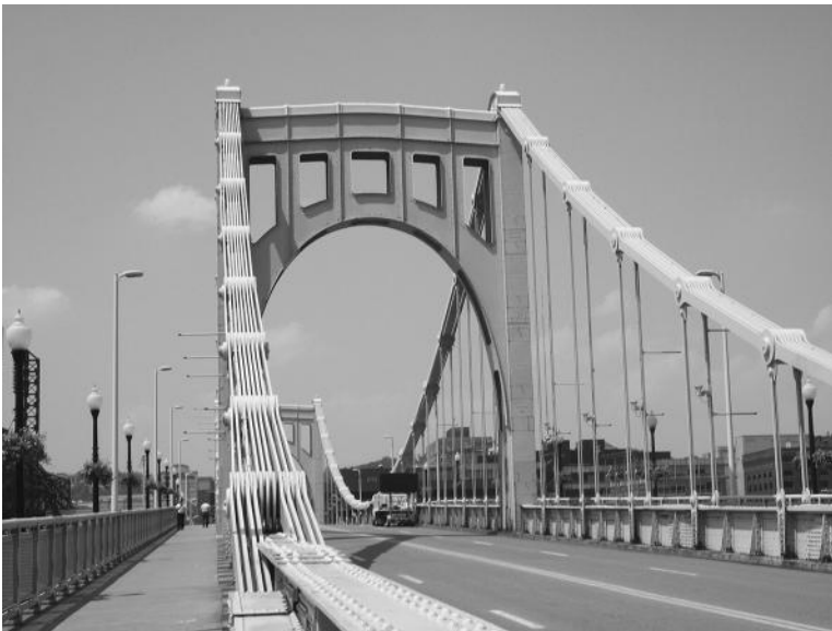
FIGURE 13.7 Fracture critical bridge superstructure.
