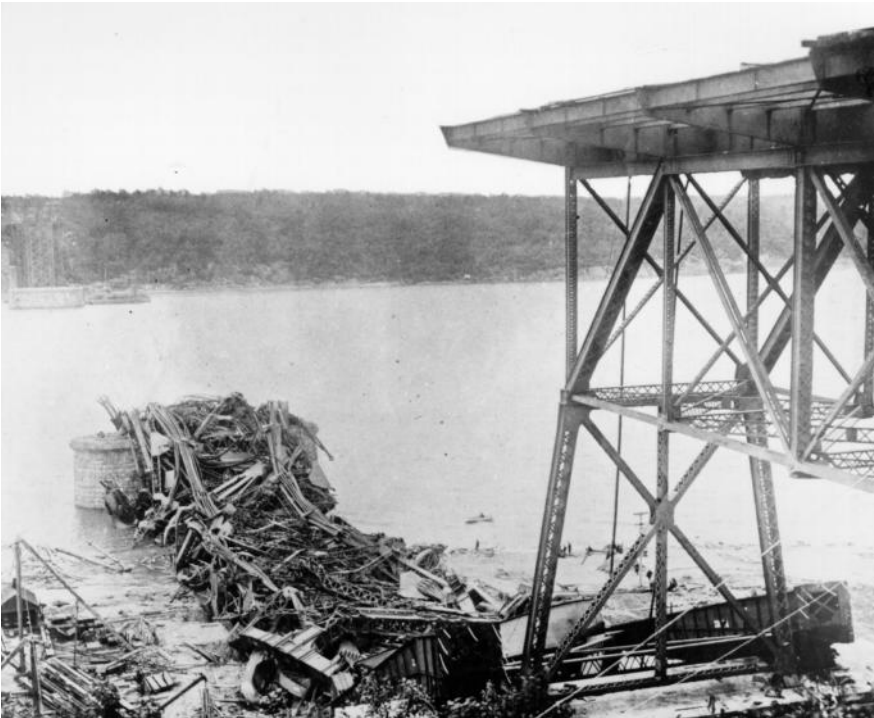
FIGURE 1.12 Wreckage of south anchor span of first Quebec railway cantilever bridge, 1907. View looking north from south shore a few days after collapse of August 29, 1907, the worst disaster in the history of bridge construction. About 20,000 tons of steelwork fell into the St. Lawrence River, and 75 workmen lost their lives.
