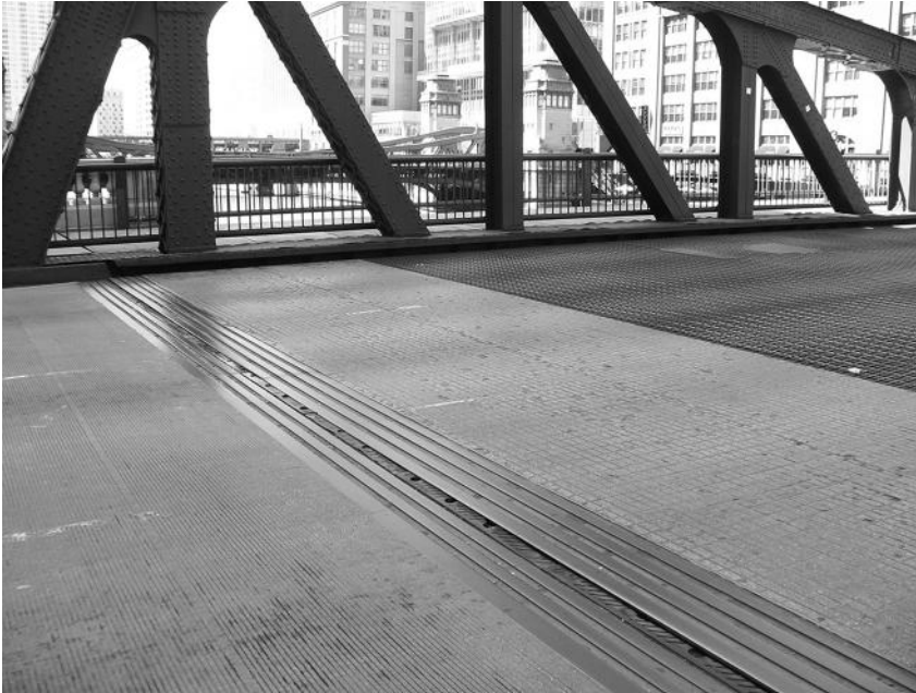
FIGURE 13.4 Bridge deck and joints.
