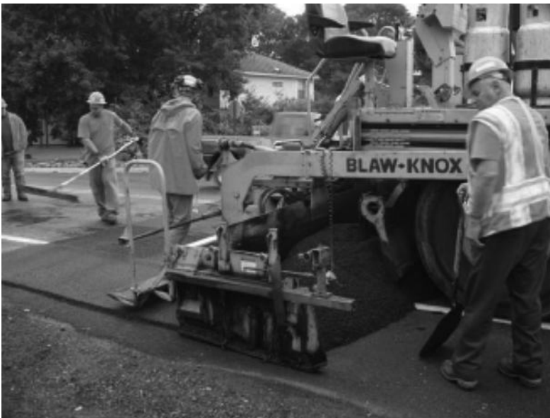
FIGURE 11.19 Wearing surface repairs. (Courtesy of the New York State Department of Transportation.)
