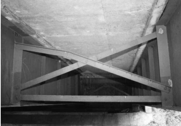
FIGURE 14.9 Modified cross frame between adjacent girders for softening repair.
