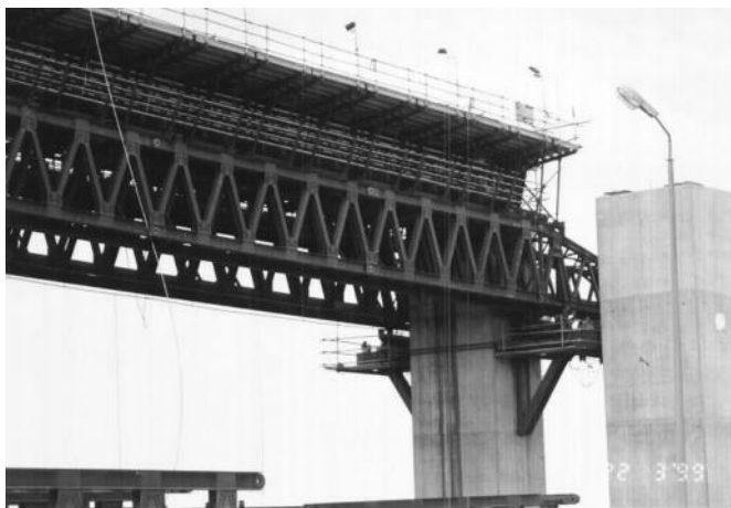
FIGURE 19.23 Mobile scaffolding for approach viaduct of the east portion.
