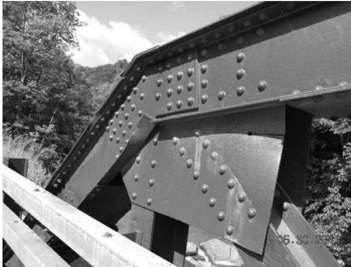
FIGURE 11.10 Visible problem in the truss compression member. (Courtesy of the New York State Department of Transportation.)
