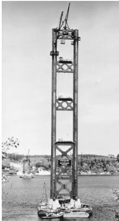
FIGURE 1.24 Tower erection, second Tacoma Narrows Bridge, Washington, 1949. This bridge replaced first Tacoma Narrows bridge, which blew down in a 40 mph (18 m/sec) wind in 1940. Tower legs are 60 ft. (18 m) on centers and 462 ft. (141 m) high. Creeper traveler is shown erecting west tower, in background. On east tower, creeper erected a Chicago boom at top of south leg; this boom dismantled creeper, then erected tower-top bracing and a stifflegged errick, which proceeded to dismantle Chicago boom. Tower manhoist can be seen at second-from-topmost landing platform. Riveting cages are approaching top of tower. Note tower-base erection kneebraces, required to ensure tower stability in free-standing condition (see Figure 1.27).
