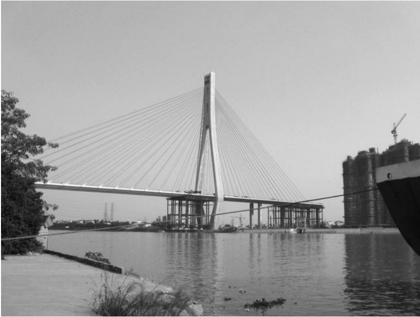
FIGURE 5.3 Overlook of the Dongsha Bridge, Guangzhou, China.
