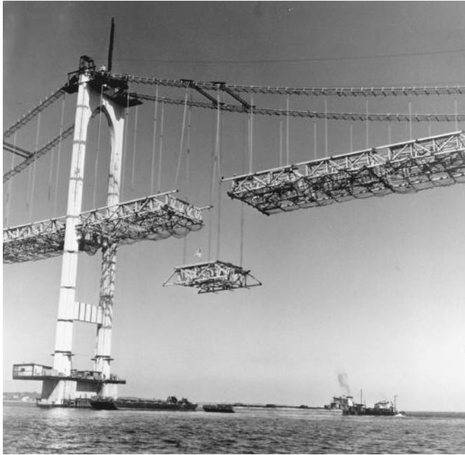
FIGURE 1.40 Suspended deck steelwork erection, Newport Bridge suspension spans, Narragansett Bay, R.I., 1968. Closing mainspan deck section is being raised into position by two cable travelers, each made up of a pair of 36 in. (0.91 m) wide-flange rolled beams that ride cables on wooden wheels. Closing section is 40-1/2 ft. (12 m) long at top-chord level, 66 ft. (20 m) wide and 16 ft. (5 m) deep, and weighs about 140 tons. (Courtesy of Bethlehem Steel Corporation.)
