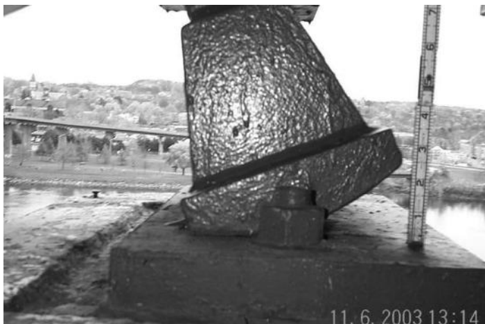
FIGURE 11.11 Red Flag due to overextended bearing. (Courtesy of the New York State Department of Transportation.)
