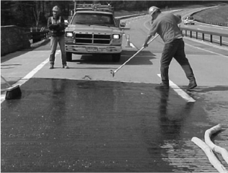
FIGURE 11.18 Concrete deck sealing. (Courtesy of the New York State Department of Transportation.)
