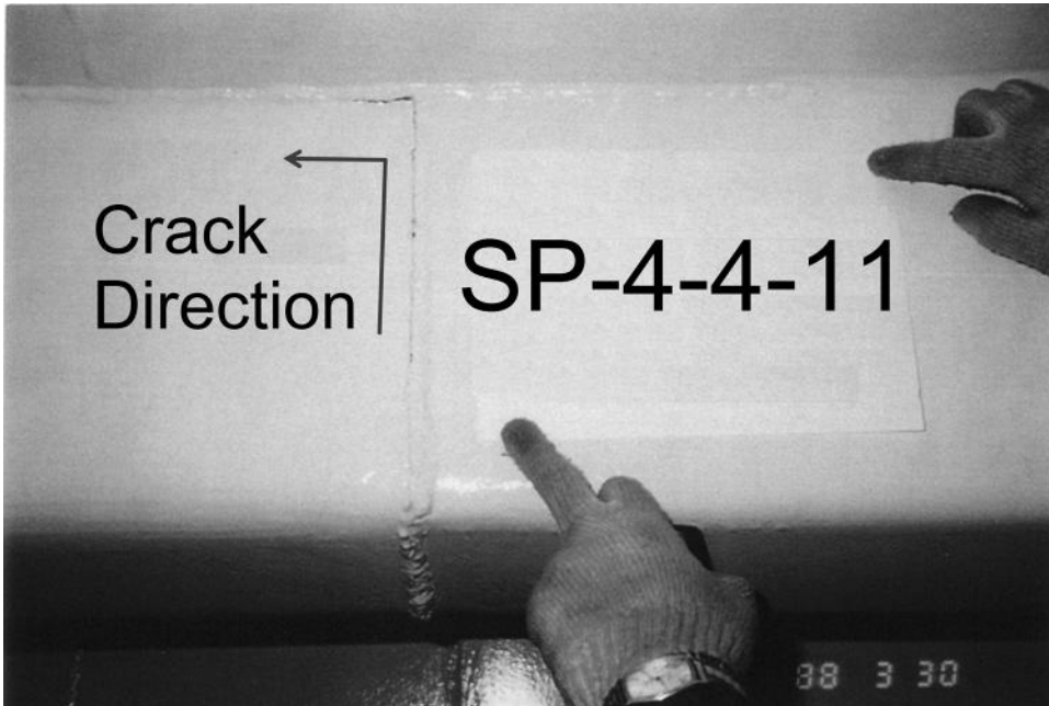
FIGURE 17.7 RR1-type fatigue crack.
