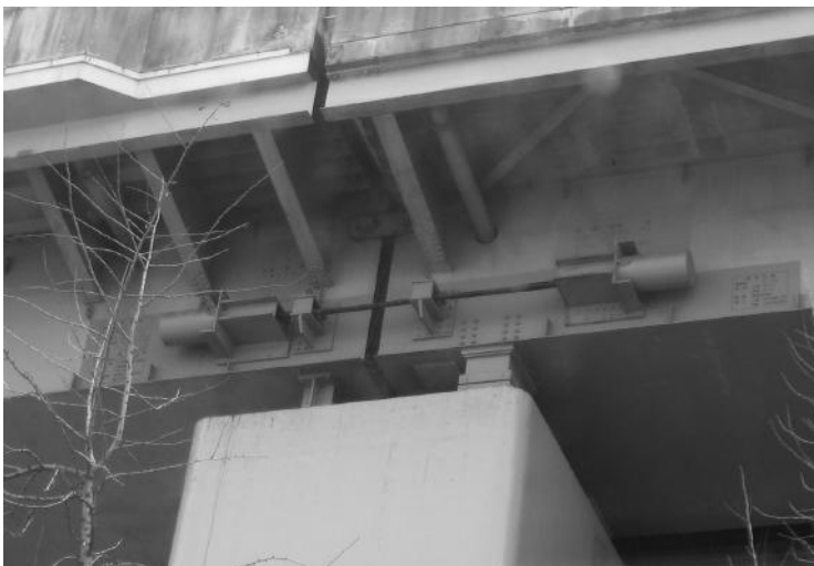
FIGURE 16.18 Seismic restrainer system.
