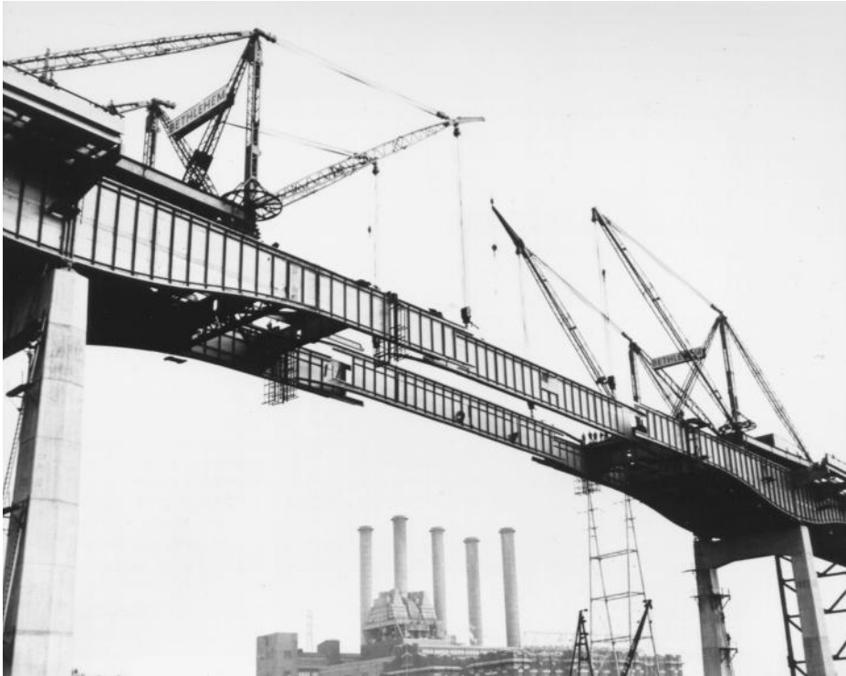
FIGURE 1.29 Erecting closing girder sections of Passaic River Bridge, New Jersey Turnpike, 1951. Huge double-boom travelers, each weighing 270 tons, erect closing plate girders of the 375 ft. (114 m) main span. Closing girders are 14 ft. (4.3 m) deep and 115 ft. (35 m) long and weigh 146 tons each. Sidewise entry was required (as shown) because of long projecting splice material. Longitudinal motion was provided at one pier, where girders were jacked to effect closure. Closing girders were laterally stable without floor steel fill-in, such that derrick falls could be released immediately. (Courtesy of Bethlehem Steel Corporation.)
