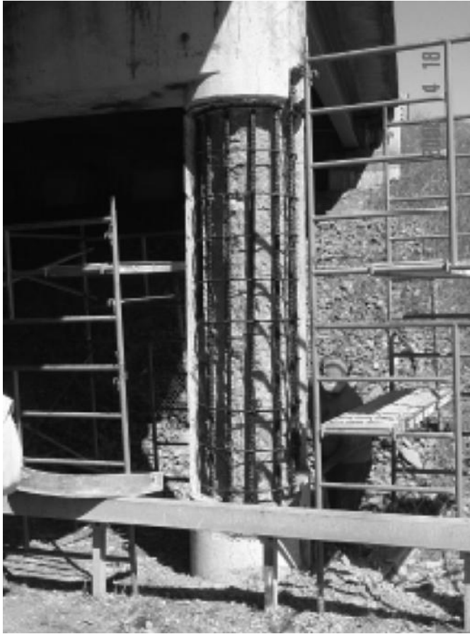
FIGURE 11.21 Repair of delaminated concrete columns. (Courtesy of the New York State Department of Transportation.)
