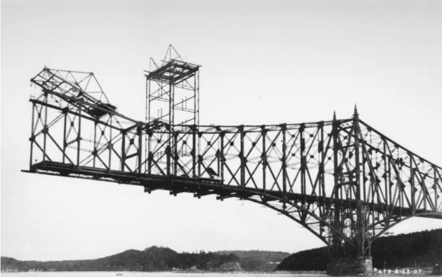
FIGURE 1.11 First Quebec railway cantilever bridge, August 23, 1907. Cantilever erection of south main span, 6 days before collapse. The tower traveler erected the anchor span (on falsework) and then the cantilever arm; then erected the top-chord traveler, which is shown erecting suspended span at end of cantilever arm. The main span of 1800 ft. (549 m) was the world's longest of any type. The sidespan bottom chords second from pier failed in compression because laticing connecting chord corner angles was deficient under secondary bending conditions.
