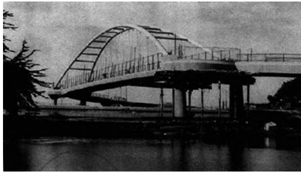
FIGURE 3.4 Berkeley Pedestrian Bridge—curved eastern approach ramp.
