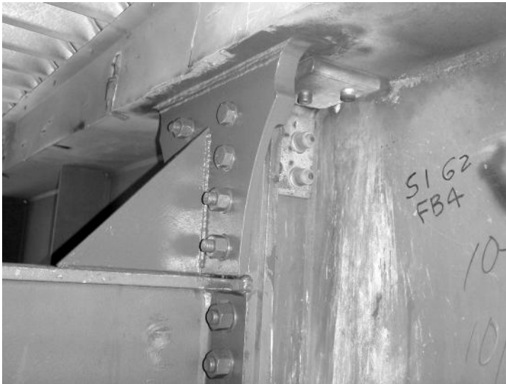
FIGURE 14.11 Repair of distortion-induced fatigue using field welding.
