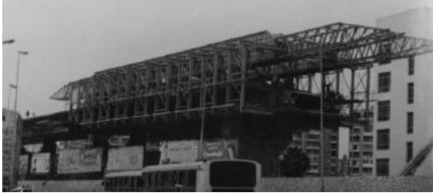
FIGURE 19.7 Stepping shuttering during concreting phase (6th October Bridge).
