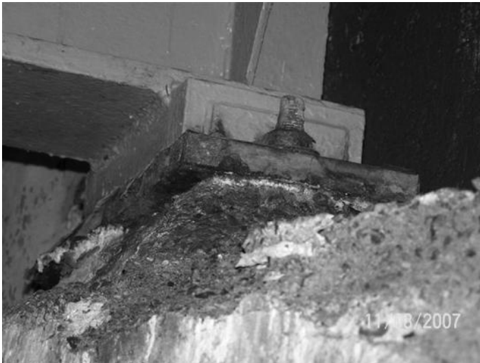
FIGURE 11.13 Yellow Flag due to loss of bearing area in a pedestal. (Courtesy of the New York State Department of Transportation.)
