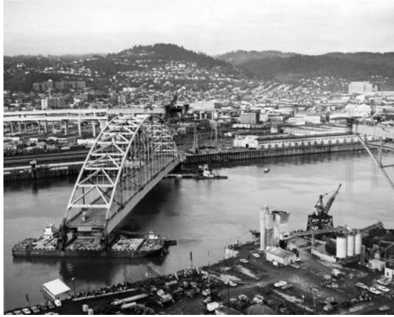
FIGURE 7.10 Floating the Fremont Bridge on barges on the Willamette River, Portland, Oregon (completed in 1973).
