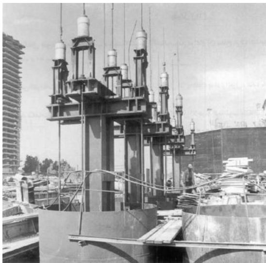
FIGURE 19.71 Erected steel frames and hydraulic jacks used for lifting the cap (El-Moneeb Bridge).
