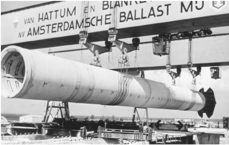
FIGURE 6.7 A prestressed concrete cylinder pile for Oosterschelde Bridge, the Netherlands.
