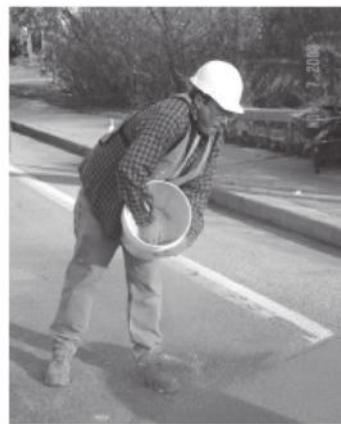
Placing aggregate
