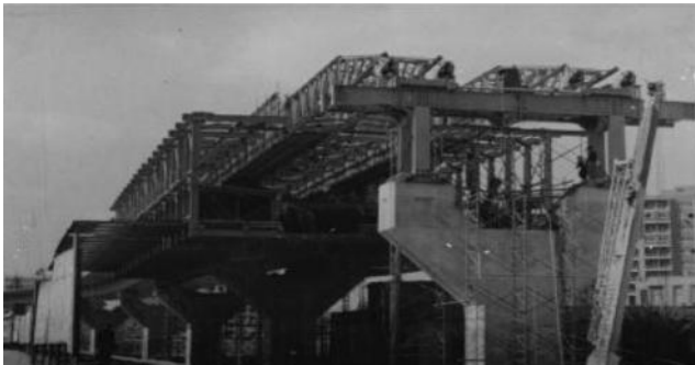
FIGURE 19.8 Stepping shuttering during advancing phase (6th October Bridge).
