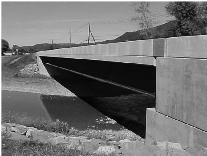
FIGURE 11.5 Concrete girder bridge. (Courtesy of the New York State Department of Transportation.)
