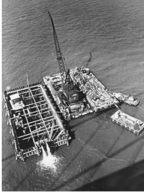
FIGURE 6.12 Dewatering the cofferdam for the main tower pier of Second Delaware Memorial Bridge.
