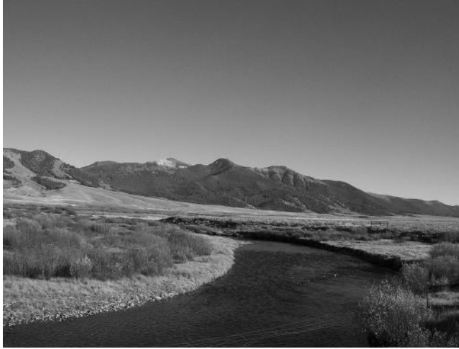
FIGURE 13.12 Eroded channel banks near the bridge.
