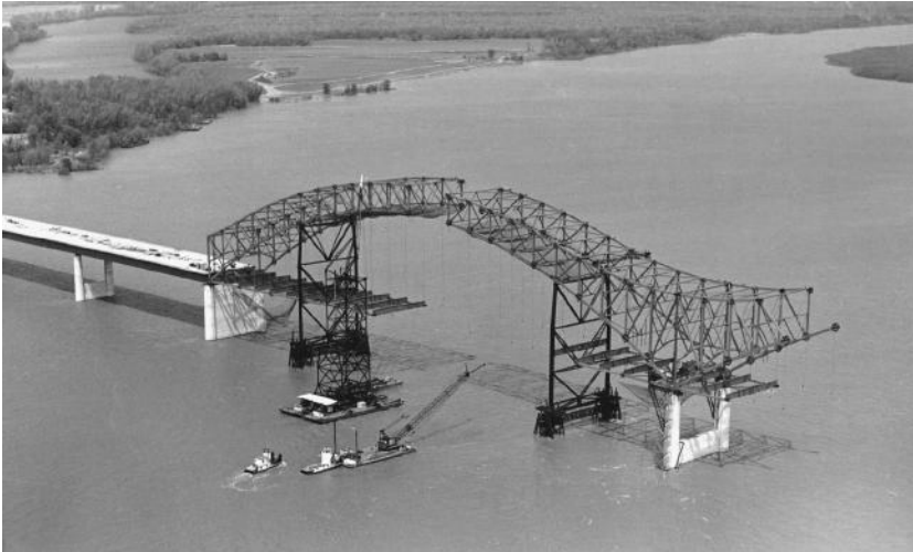
FIGURE 1.43 Erection of west arch span of twin-arch Hernando de Soto Bridge, Memphis, Tenn., 1972. The two 900 ft. (274 m) continuous-truss tied-arch spans were erected by a high-tower derrick boat incorporating a pair of barges. West-arch steelwork (shown) was cantilevered to midspan over two pile-supported falsework bents. Projecting east-arch steelwork (at right) was then cantilevered to midspan (without falsework) and closed with falsework-supported other half-arch. (Courtesy of Bethlehem Steel Corporation.)
