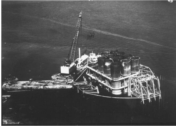
FIGURE 6.16 Open caisson for Sunshine Bridge across the Mississippi River: this caisson tipped during the removal of false bottoms and is shown being righted by jacking against dolphins.
