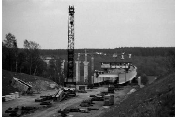
FIGURE 7.8 Spans were assembled behind the abutment and launched forward on roller bearings.
