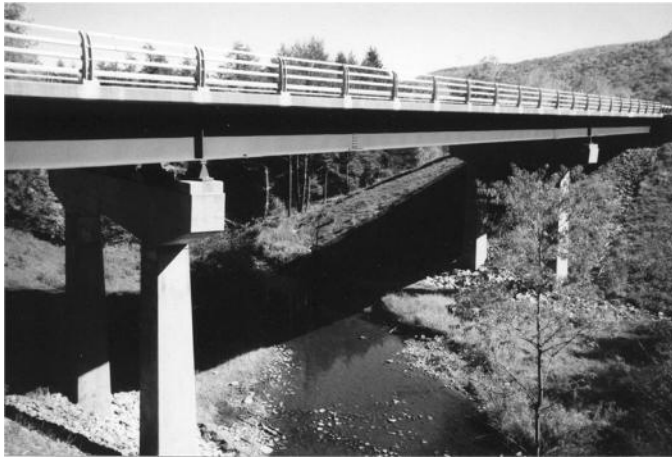
FIGURE 11.4 Steel-girder bridge with concrete deck. (Courtesy of the New York State Department of Transportation.)
