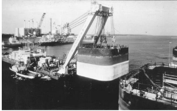
FIGURE 6.30 Setting a prefabricated box caisson on which a temporary cofferdam is mounted, the Great Belt Eastern Bridge.
