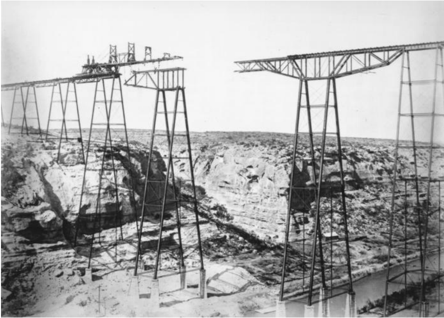
FIGURE 1.19 Pecos River railway viaduct, Texas, 1892. Erection by massive steam-powered wood traveler having many sets of falls and very long reach. Cantilever-truss main span has 185 ft. (56 m) clear opening.
