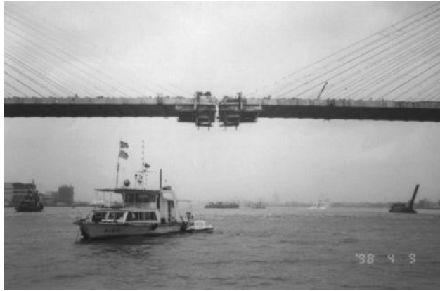
FIGURE 5.15 Two cantilever ends are meeting very well.
