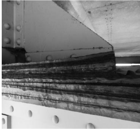
FIGURE 16.27 Severe pack rust in riveted connections of steel bridge.
