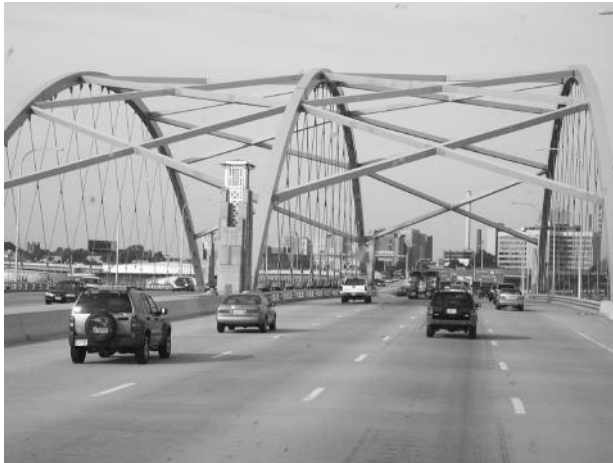
FIGURE 13.14 Bridge superstructure paint.
