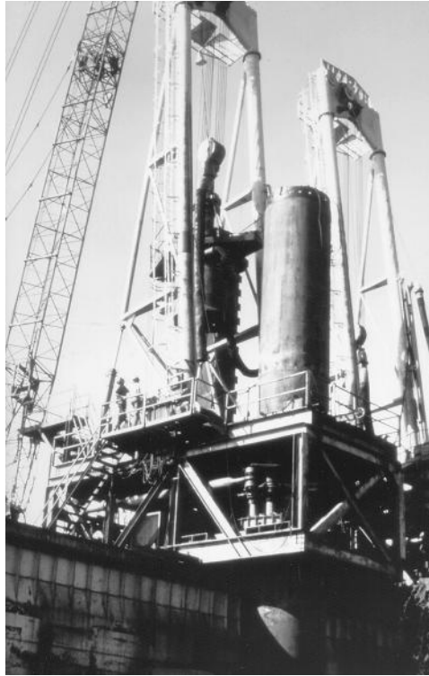
FIGURE 6.3 A steel tubular pile being installed from a jack-up barge: the socket will be drilled into rock and the entire pile filled with tremie concrete.
