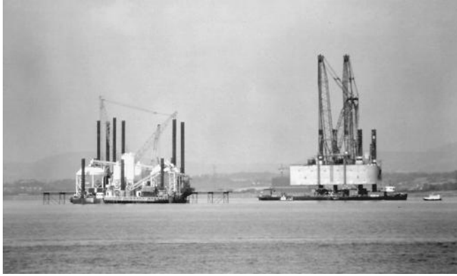
FIGURE 6.28 Installing precast concrete box caissons for the Second Severn Crossing: an extreme tidal range of 10 m and a high tidal current imposed severe demands on installation procedures and equipment.
