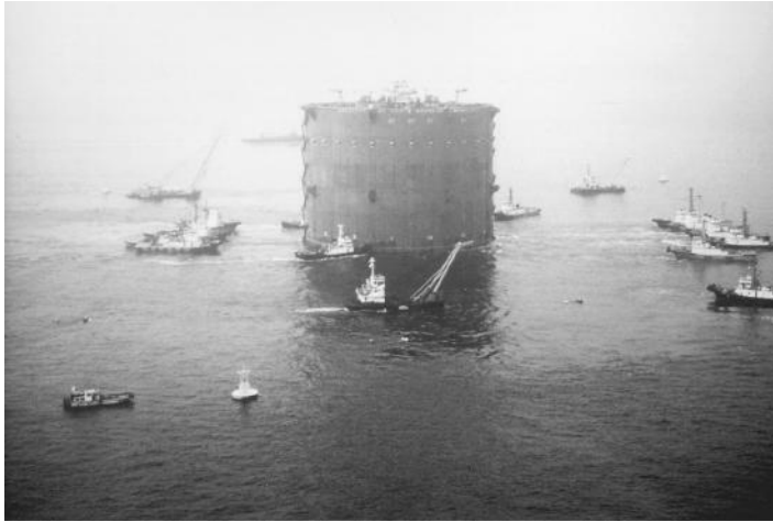
FIGURE 6.19 Steel box caisson being positioned for the Akashi Strait Suspension Bridge despite strong currents.
