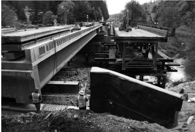
FIGURE 7.9 New span (left) being moved laterally into position after existing span was skidded off to the side (right).
