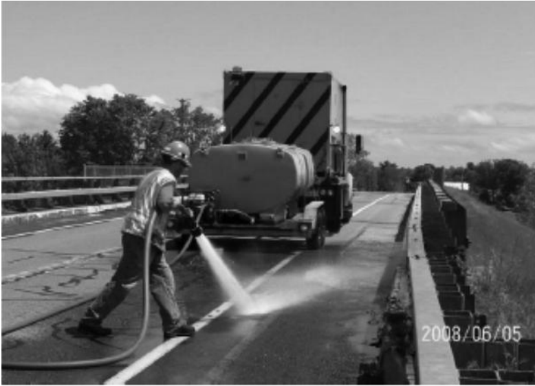
FIGURE 11.16 Bridge washing. (Courtesy of the New York State Department of Transportation.)
