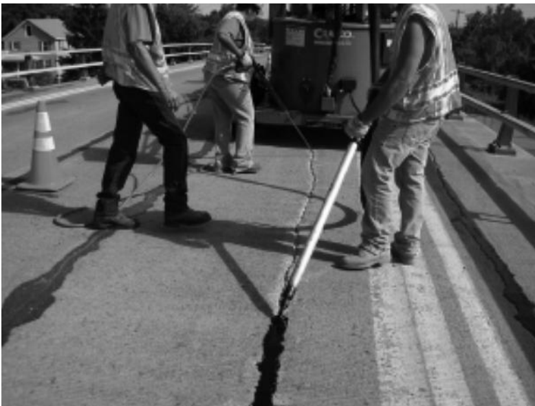
FIGURE 11.17 Crack sealing. (Courtesy of the New York State Department of Transportation.)
