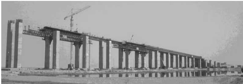
FIGURE 19.22 Construction of the approach viaduct in the east portion (Nov. 99).
