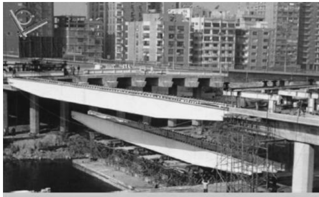
FIGURE 19.48 First group of steel beams during lifting (El-Moneeb Bridge).
