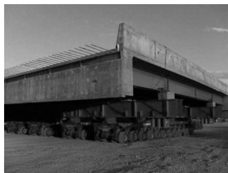
FIGURE 7.13 Moving full superstructure I-80 State to 1300 east using self-propelled modular transporters.
