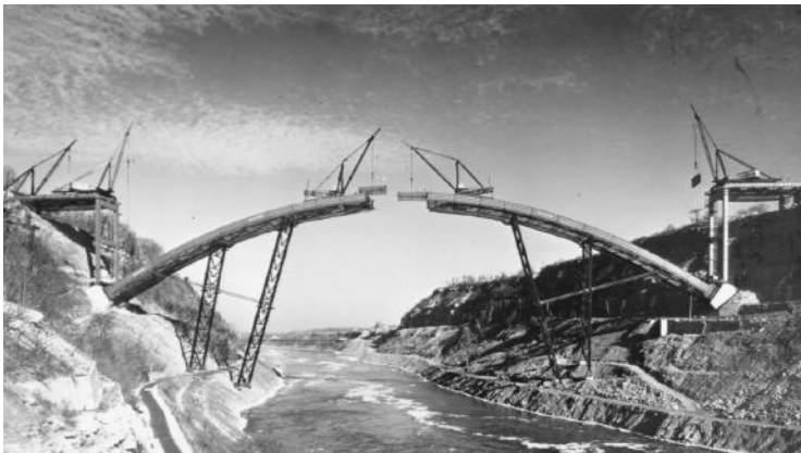
FIGURE 1.4 Lewiston-Queenston arch bridge, near Niagara Falls, New York, 1962. The longest fixed-arch span in the United States at 1000 ft. (305 m); rise is 159 ft. (48 m). Box arch-rib sections are typically about 3 × 13 1/2 ft. (0.9 × 4.1 m) in cross-section and about 44 1/2 ft. (13.6 m) long. Job was estimated using erection tiebacks (same as shown in Figure 1.3), but subsequent studies showed the long, sloping falsework bents to be more economical (even if less secure looking). Much permanent steelwork was used in the falsework bents. Derricks on approaches load steelwork onto material cars that travel up arch ribs. The 115-ton-capacity travelers are shown erecting the last full-length arch-rib sections, leaving only the short, closing crown sections to be erected. Canada is at left, the United States at right. (Courtesy of Bethlehem Steel Corporation.)
