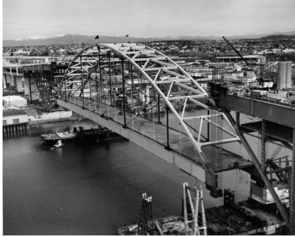
FIGURE 7.11 Lifting the Fremont Bridge main arch span using strand jacks.
