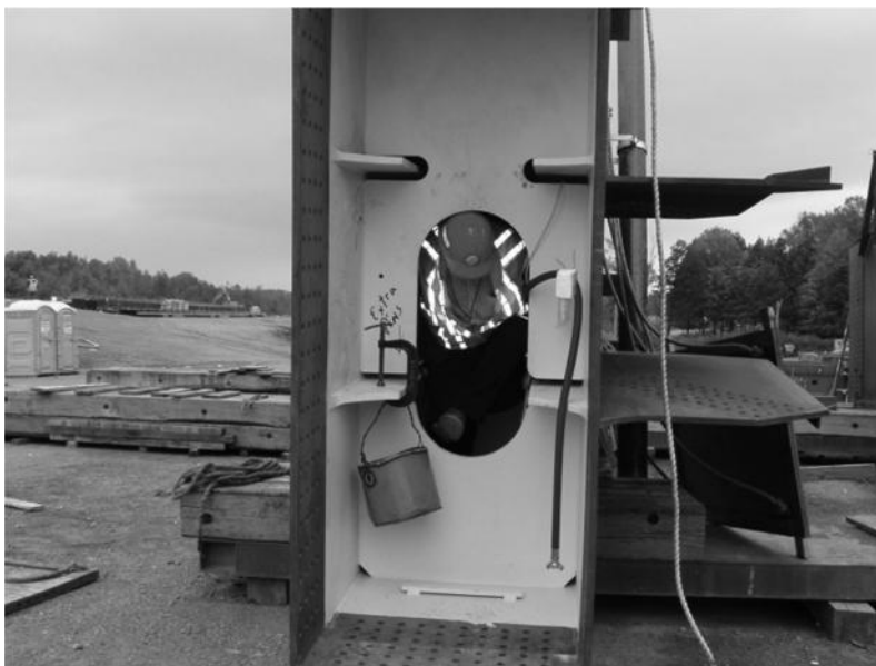
FIGURE 11.6 Bridge detail with maintenance access.
