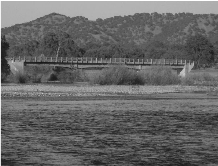
FIGURE 13.11 Scour at both ends of bridge.
