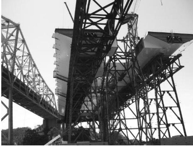
FIGURE 13.13 Existing bridge and bridge replacement.
