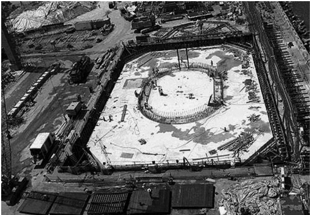
FIGURE 4.14 Tower foundation construction, Stonecutters Bridge ( http://www.zgjw.net ).
