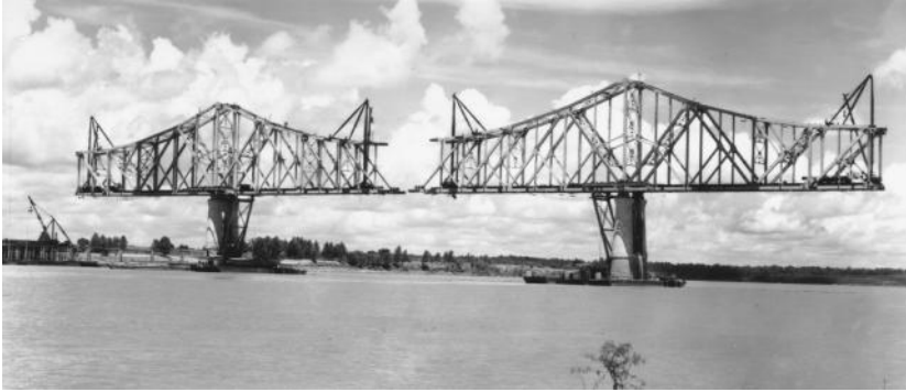
FIGURE 1.23 Balanced-cantilever erection, Governor O.K. Allen railway/highway cantilever bridge, Baton Rouge, La., 1939. First use of long balanced-cantilever erection procedure in the U.S. On each pier 650 ft. (198 m) of steelwork, about 4000 tons, was balanced on the 40 ft. (12 m) base formed by a sloping falsework bent. The compression load at the top of the falsework bent was measured at frequent intervals and adjusted by positioning a counterweight car running at bottom-chord level. The main spans are 848-650-848 ft. (258-198-258 m); 650 ft. span shown. (Courtesy of Bethlehem Steel Corporation.)
