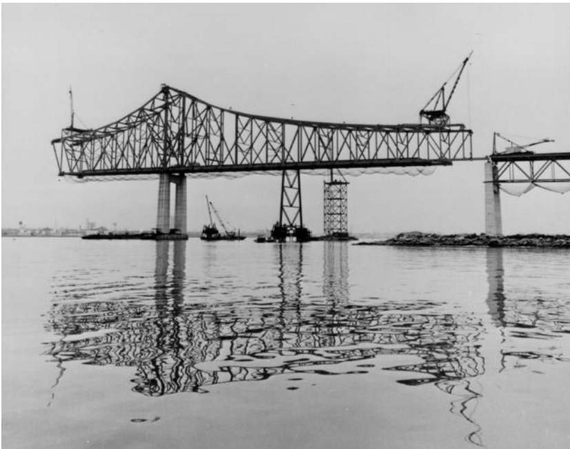
FIGURE 1.44 Closure of east side span, Commodore John Barry cantilever truss bridge, Chester, Pa., 1973. High-tower derrick boat (in background) started erection of trusses at both main piers, supported on falsework; then erected top-chord travelers for main and side spans. Sidespan traveler carried steelwork erection to closure, as shown, and falsework bent was then removed. East-mainspan traveler then cantilevered steelwork (without falsework) to midspan, concurrently with cantilever erection by west-half mainspan traveler, and trusses were closed at midspan. Commodore Barry has 1644 ft. (501 m) main span, longest cantilever span in the U.S., and 822 ft. (251 m) side spans. (Courtesy of Bethlehem Steel Corporation.)
