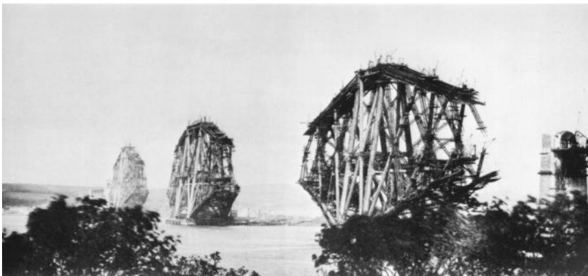
FIGURE 1.18 The massive cantilevers of the Forth bridge, shown under erection, were conceived in the shadow of the Tay bridge disaster.
