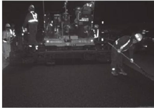
(4) Covering with asphalt pavement
