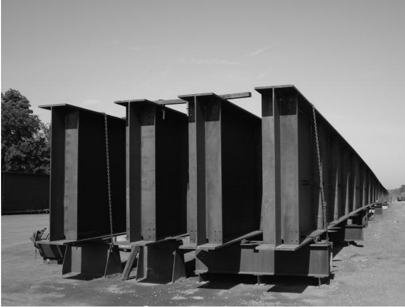
FIGURE 2.7 Girders in line assembly. Such assembly may be accomplished with the girders vertical, as shown, or horizontal, in the “lay down” position.
