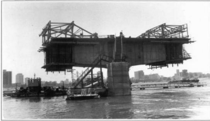
FIGURE 19.31 Moving travelers on the stump (Rod El-Farag Bridge).
