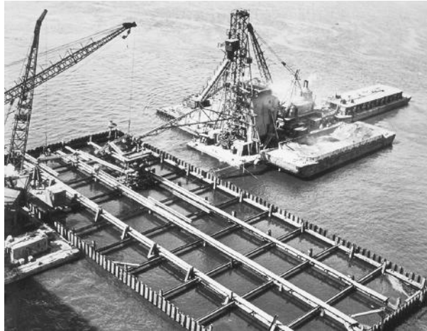
FIGURE 6.9 Large steel sheet pile cofferdam for Second Delaware Memorial Bridge, showing bracing frames.
