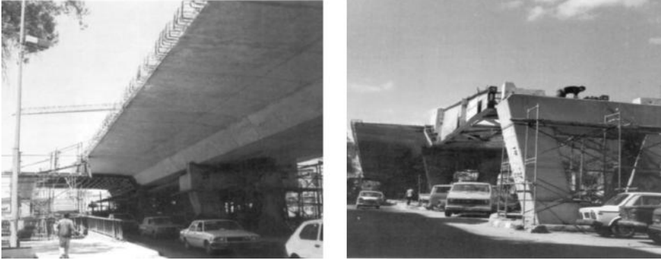
FIGURE 19.37 Deck pushing system in Zamalek Bridge, Cairo, Egypt.
