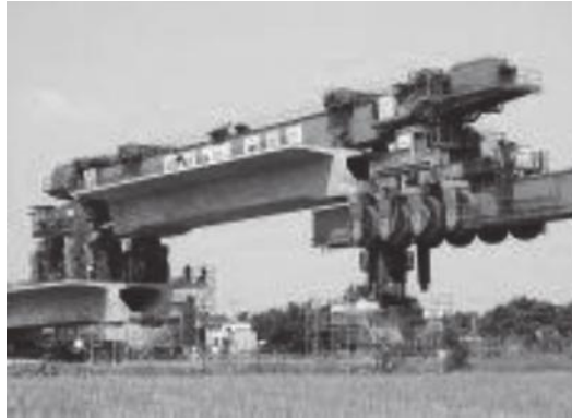
FIGURE 19.55 Example of full-span precast method. (From VSL. Bridge Construction Partner , VSL International, Köniz, Switzerland, 2013.)
