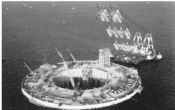
FIGURE 6.10 Slurry wall cofferdam for Kawasaki Island ventilation shaft, Trans-Tokyo Bay Tunnels and Bridge.
