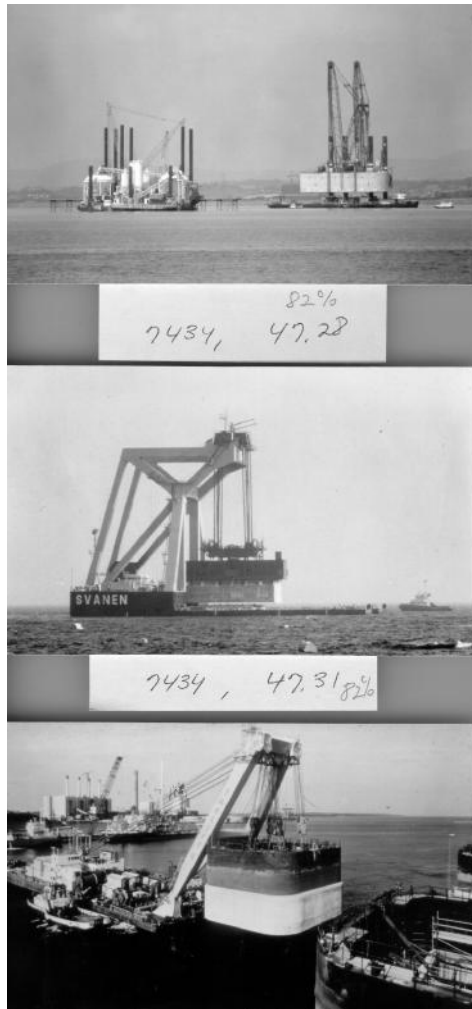
FIGURE 6.31 Setting a 7000 t prefabricated box caisson, the Great Belt Western Bridge.
