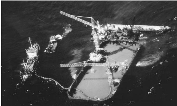
FIGURE 6.27 A prefabricated box caisson is floated into position, the Great Belt Eastern Bridge: note the temporary cofferdam above the concrete caisson.
