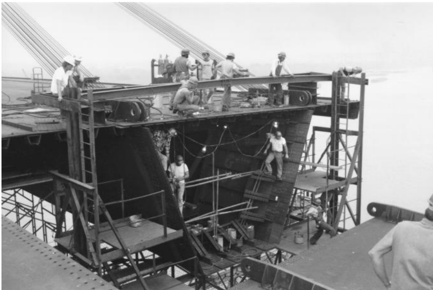
FIGURE 1.10 Luling Bridge deck steelwork erection, 1982; view looking northeast (refer to Figure 1.9). The twin box girders are 14 ft. (4.3 m) deep; the deck plate is 7/16 in. (11 mm) thick. Girder section 16-east is being raised into position (lower right) and will be secured by large-pin hinge bars prior to fairing-up of joint holes and permanent bolting. Temporary erection stays are jumped forward as girder erection progresses.
