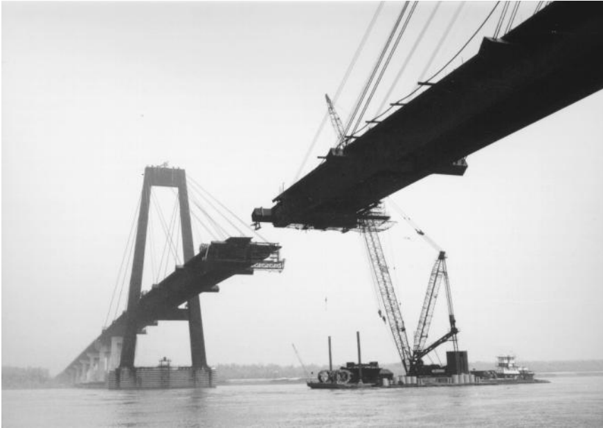
FIGURE 1.9 Cable-stayed orthotropic-steel-deck bridge over Mississippi River at Luling, Louisiana, 1982; view looking northeast. The main span is 1222 ft. (372 m); the A-frame towers are 350 ft. (107 m) high. A barge-mounted ringer derrick erected the main steelwork, using a 340 ft. (104 m) boom with a 120 ft. (37 m) jib to erect tower components weighing up to 183 tons, and using a shorter boom for deck components. Cable stays at the ends of projecting cross girders are permanent; others are temporary erection stays. Girder section 16-west of north portion of bridge, erected a few days previously, is projecting at left; companion girder section 16-east is on barge ready for erection (see Figure 1.10).
