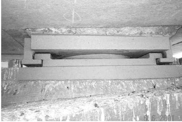
FIGURE 1.11 Pot bearing application.
