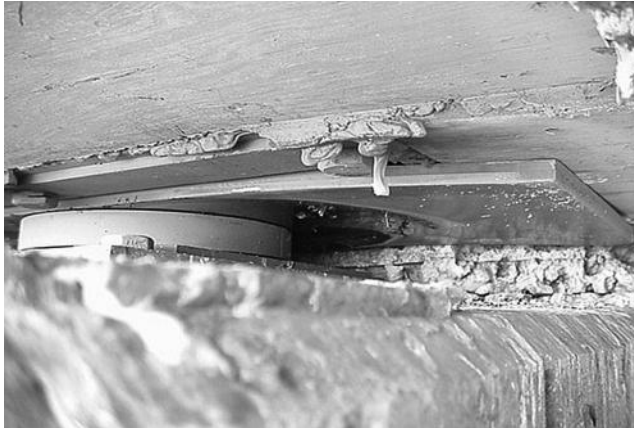
FIGURE 1.15 Spherical bearing application.
