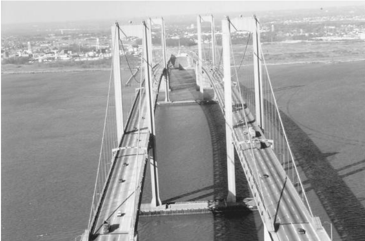
FIGURE 3.15 Delaware Memorial Bridges. (Courtesy of D. Sailors.)
