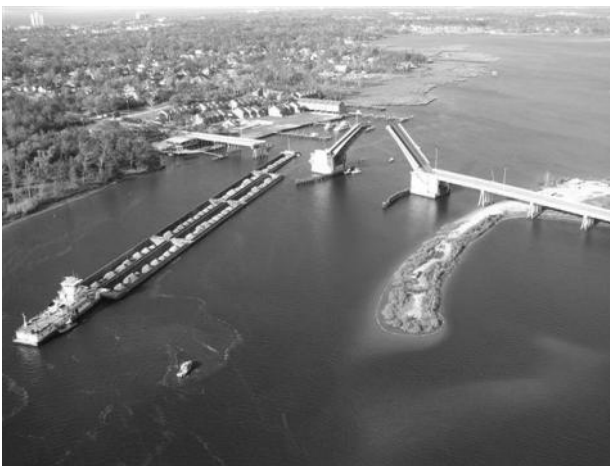
FIGURE 4.3 Popps Ferry Bridge, MS (2009).
