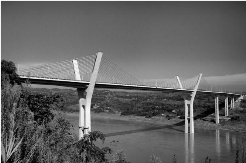
FIGURE 3.14 Jiayue Bridge, in Chongqing City, China. (Courtesy of Man-Chung Tang.)
