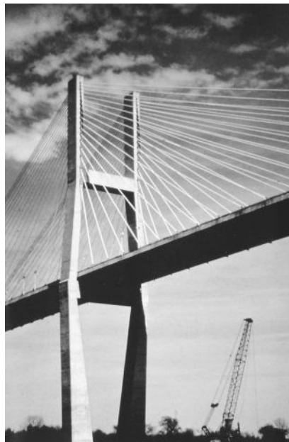
FIGURE 3.20 Talmadge Bridge, Georgia. (Courtesy of T. Y. Lin International.)
