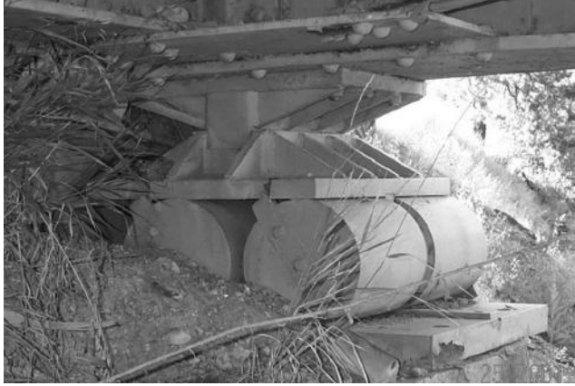
FIGURE 1.9 Nested roller bearing application.
