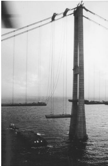
FIGURE 3.23 Great Belt Bridge, Denmark. (Courtesy of Ben C. Gerwick, Inc.)
