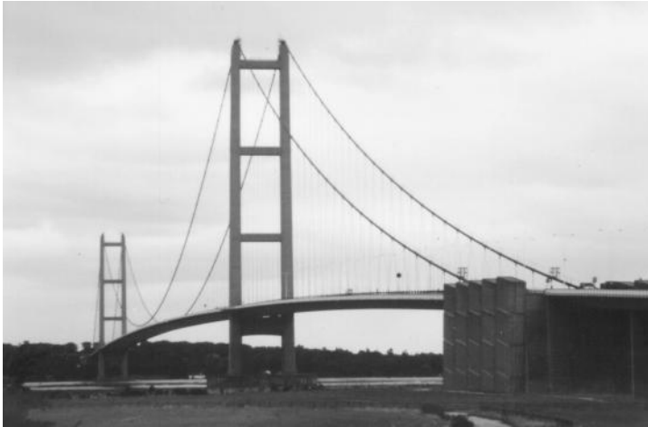
FIGURE 3.22 Humber Bridge, England. (Courtesy of Charles Seim.)
