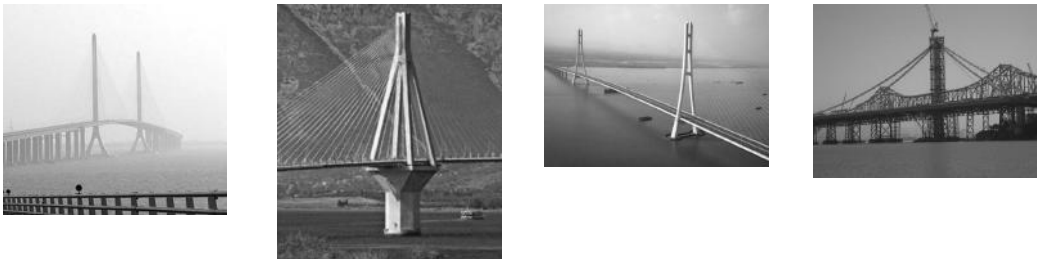
FIGURE 3.19 Distinctive towers for cable-stayed and suspension bridges.
