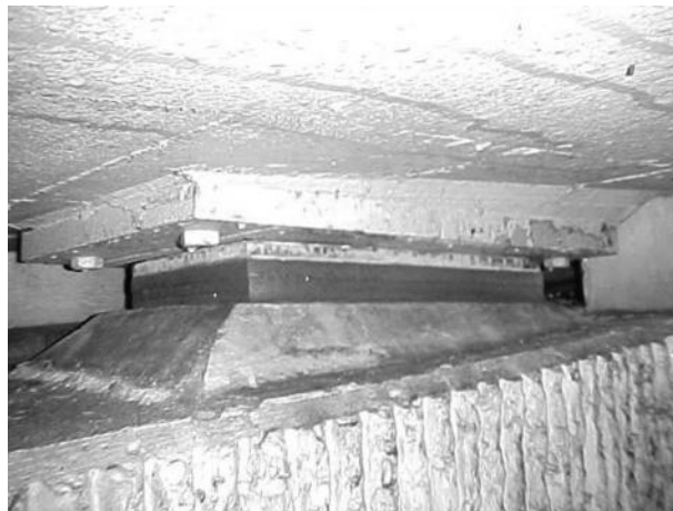
FIGURE 1.4 Fabric pad sliding bearing application.
