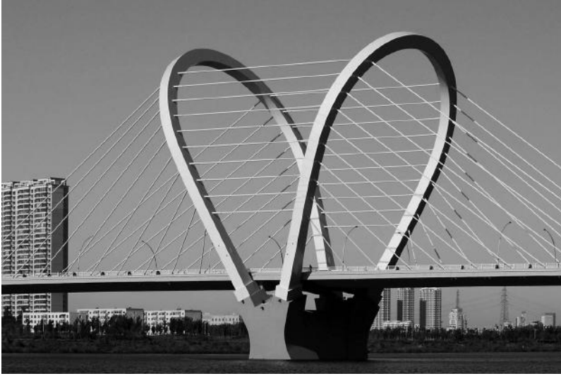
FIGURE 3.13 Sanhao Bridge, Shenyang, China. (Courtesy of Man-Chung Tang.)
