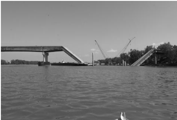
FIGURE 4.2 I-40 Bridge over Arkansas River, OK (2002).
