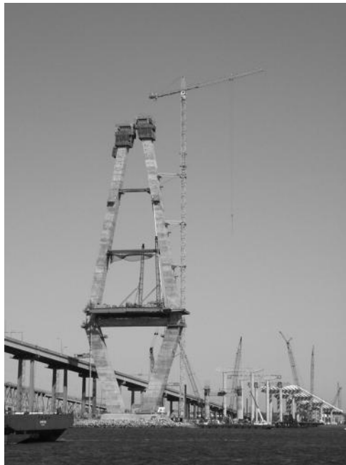
FIGURE 3.8 Cooper River Bridge, Charleston, South Carolina, under construction. (Courtesy of Charles Seim.)
