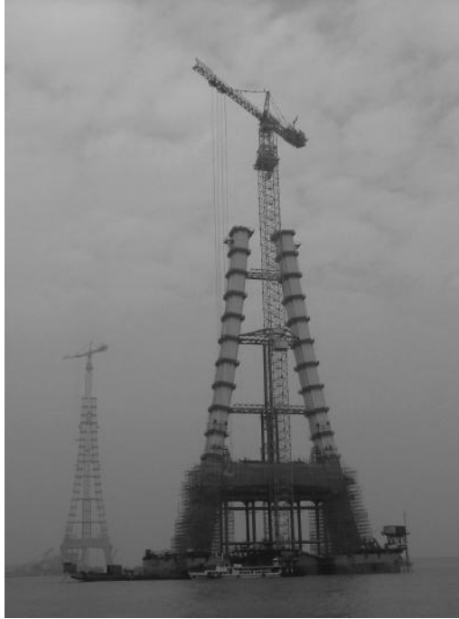
FIGURE 3.12 Third Nanjing Yangtze River Bridge Towers under construction. (Courtesy of Charles Seim.)
