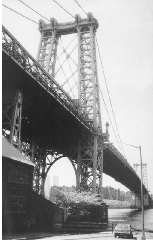
FIGURE 3.5 Williamsburg Bridge, New York. (Courtesy of Charles Seim.)
