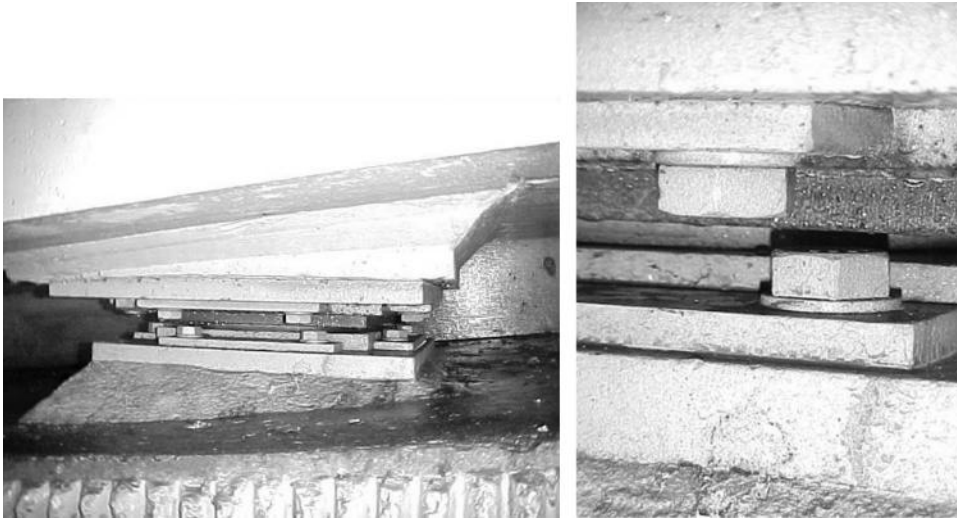
FIGURE 1.13 Disc bearing application.
